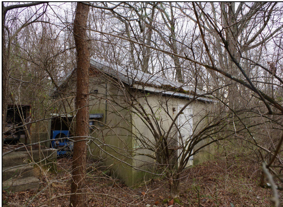
Photo 91: Building 0324A, north elevation
