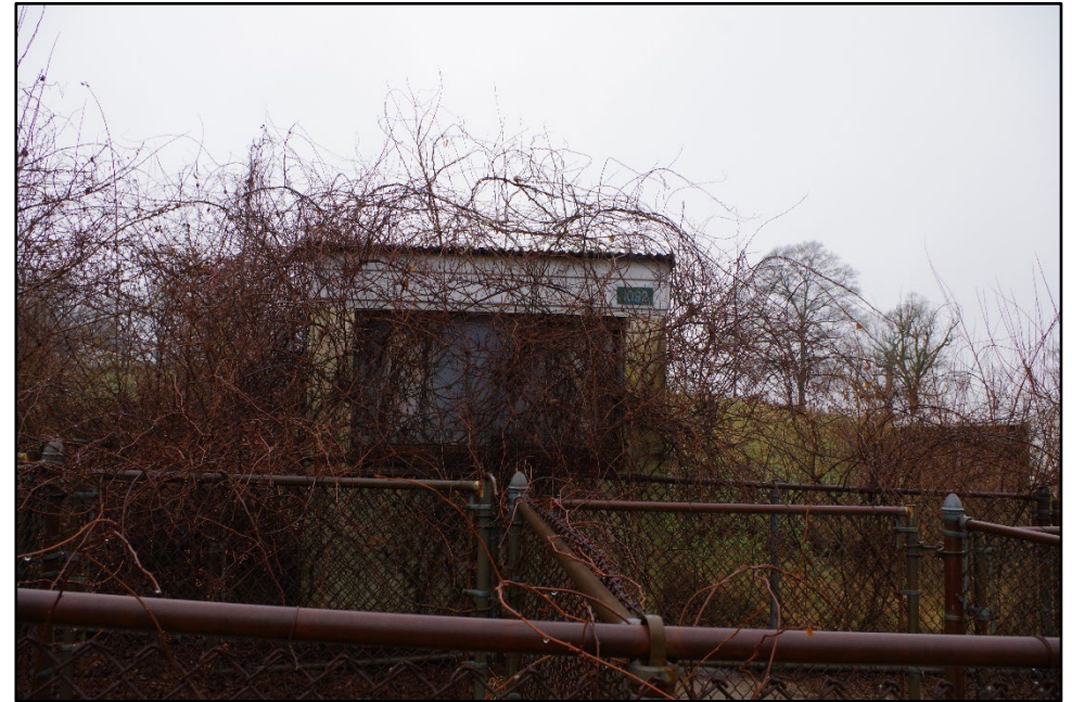
Photo 360: Building 1092, view of building and pen
