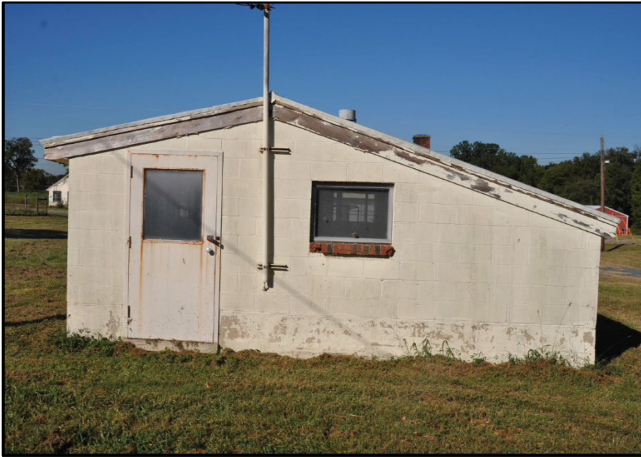
Photo 399: Building 1328, east elevation; photograph courtesy of Brian Clevon, 2017
