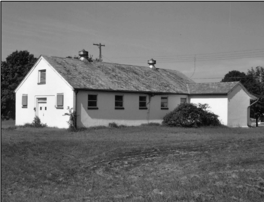
Photo 337: Building 1064, south and east elevations; photograph courtesy of Brian Clevon, 2017
