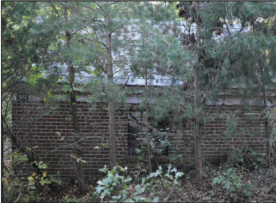
Photo 357: Building 1073, west elevation; photograph courtesy of Brian Clevon, 2017
