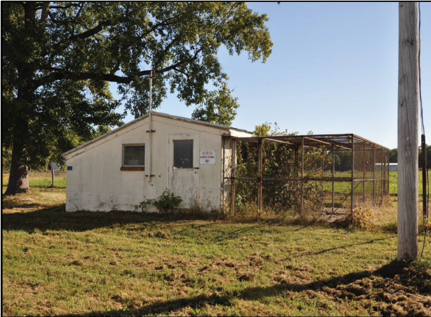
Photo 405: Building 1329, west and south elevations; photograph courtesy of Brian Clevon, 2017
