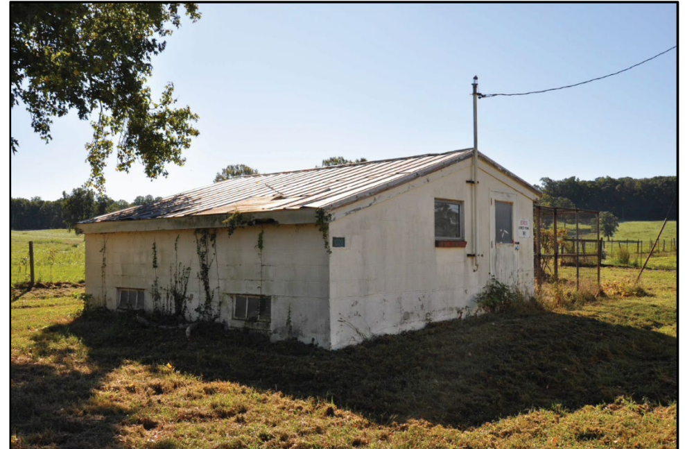
Photo 406: Building 1329, north and west elevations; photograph courtesy of Brian Clevon, 2017
