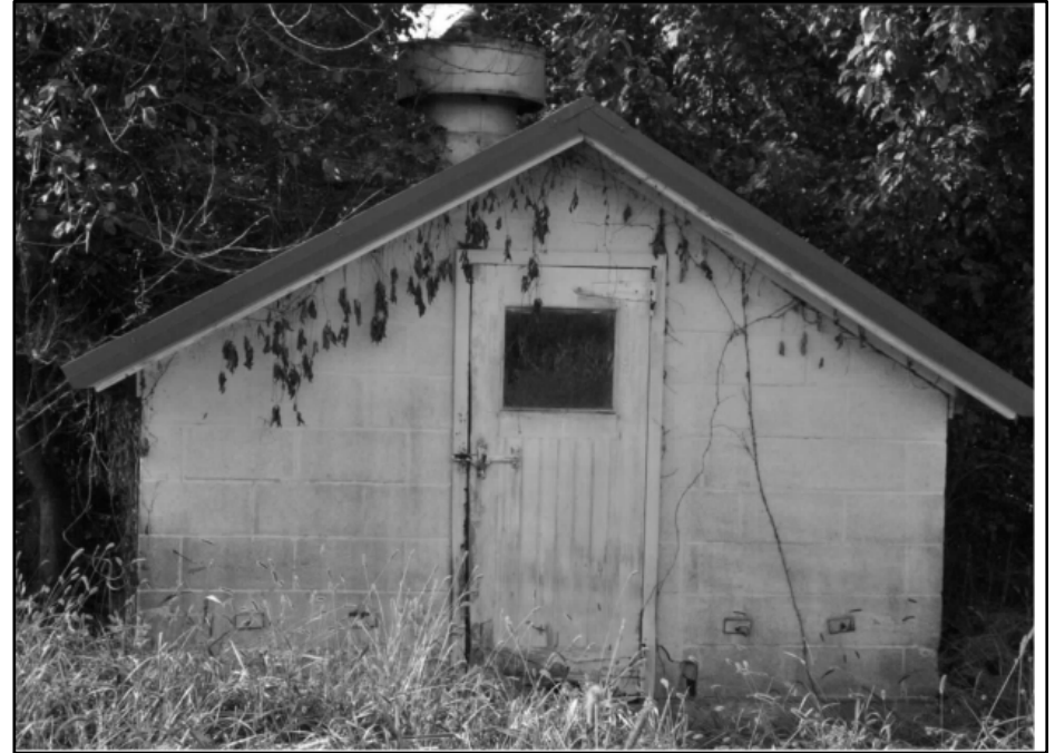
Photo 294: Building 04541C, north elevation; photograph courtesy of Mark Edwards and Brian Clevon, 2016
