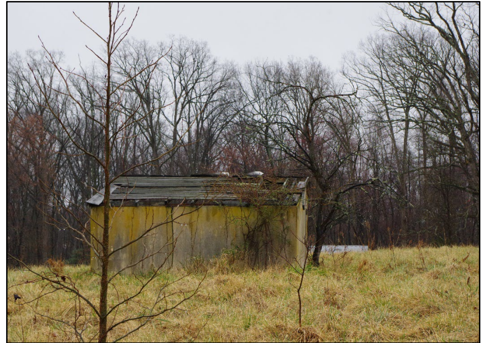
Photo 129: Building 0336B and 0336C, overview
