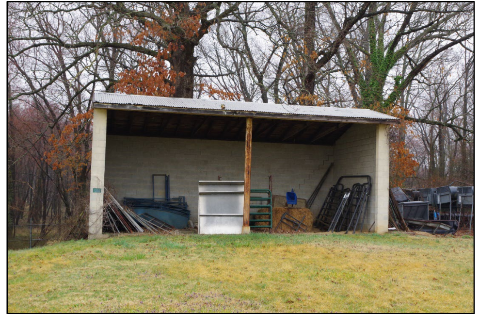
Photo 408: Building 1330, north elevation
