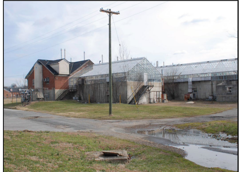
Photo 29: Building 0050, west and south elevations; photograph courtesy of Mark Edwards and Brian Clevin, 2016
