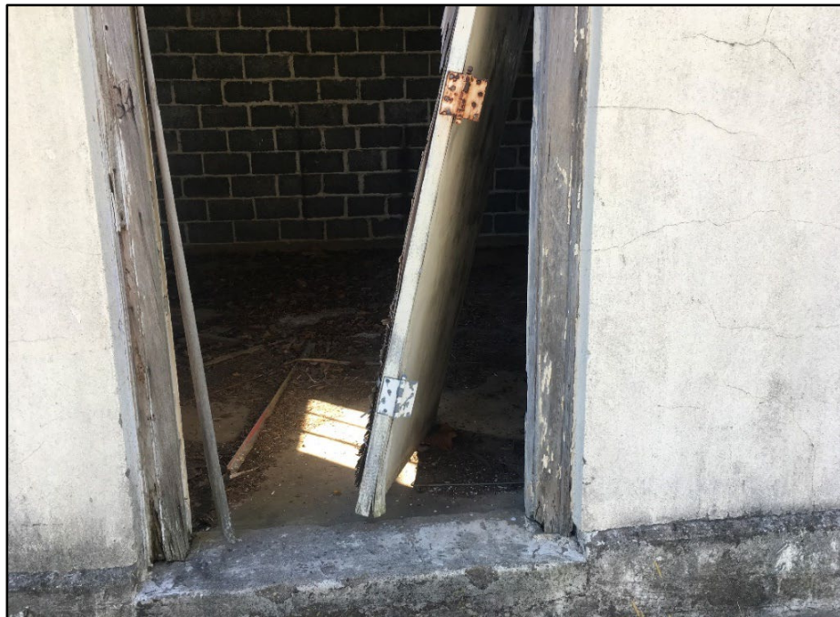
Photo 377: Building 1183, entrance detail on north elevation
