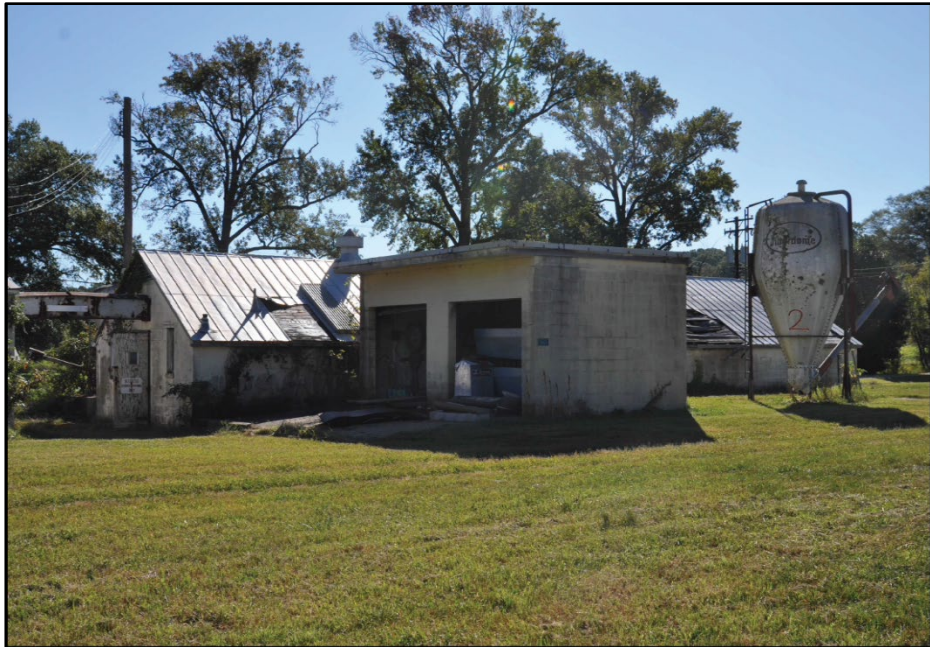
Photo 417: Building 1422, north and west elevations; photograph courtesy of Brian Clevin, 2017
