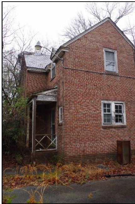
Photo 353: Building 1072, south elevation
