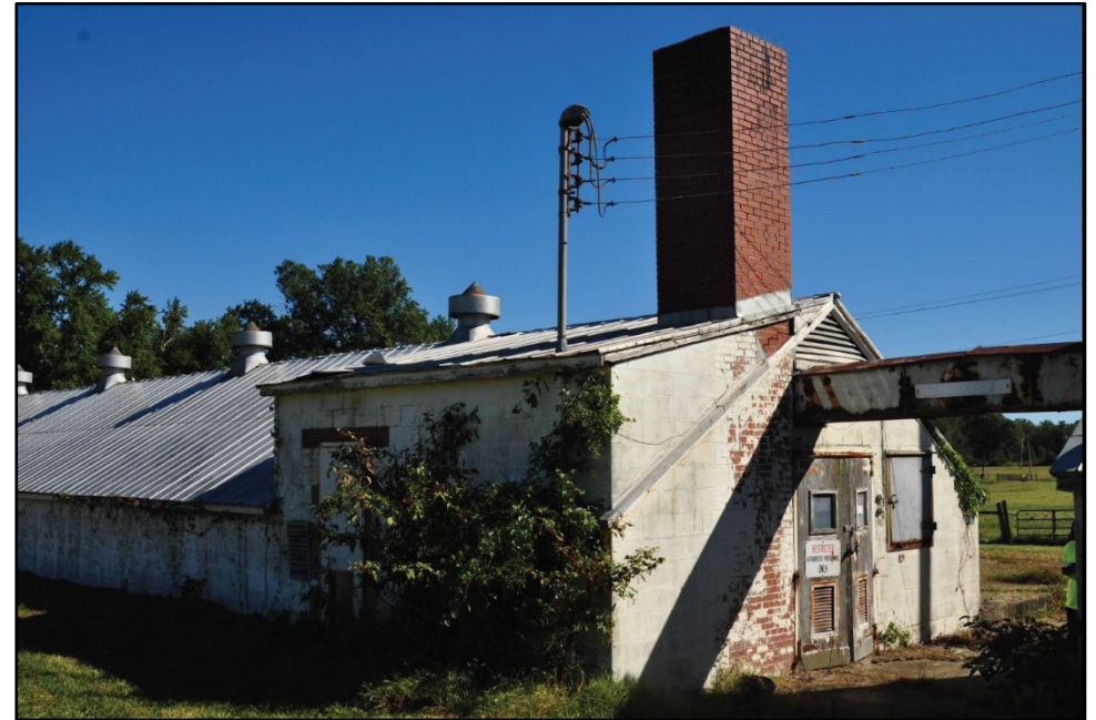
Photo 420: Building 1425, west and south elevations; photograph courtesy of Brian Clevin, 2017
