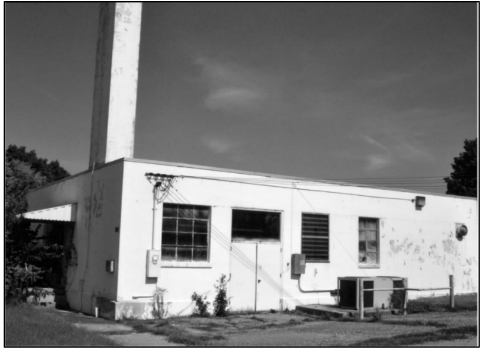
Photo 372: Building 1120, west and south elevations; photograph courtesy of Brian Clevin, 2017
