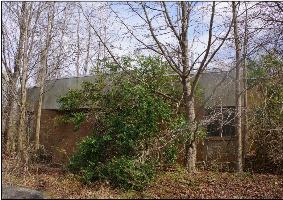
Photo 154: Building 0339F, overview
