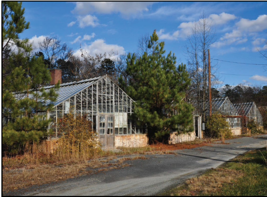
Photo 246: Building 0470, west and south elevations; photograph courtesy of Brian Clevon, 2017.
