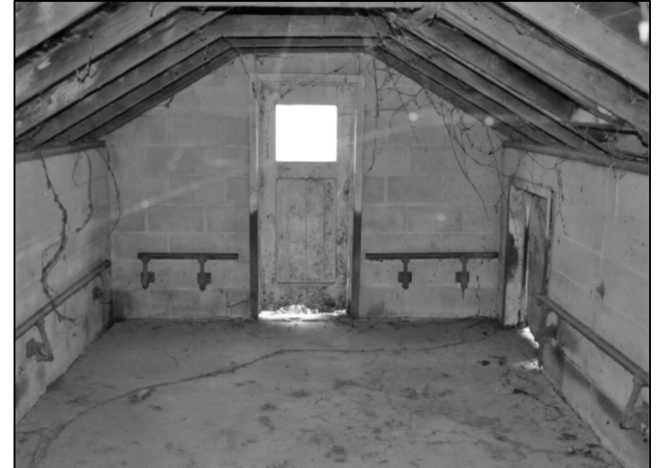
Photo 296: Building 04541C, interior; photograph courtesy of Mark Edwards and Brian Clevon, 2016
