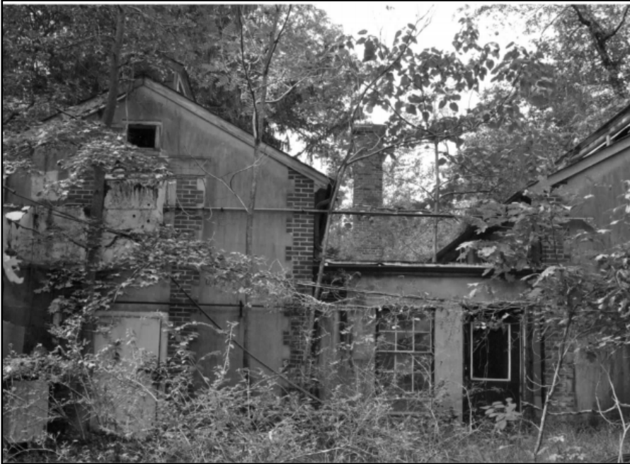
Photo 262: Building 0474, east elevation; photograph courtesy of Mark Edwards and Brian Clevon, 2016
