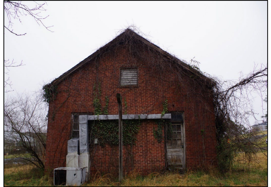
Photo 25: Building 0044, southwest elevation
