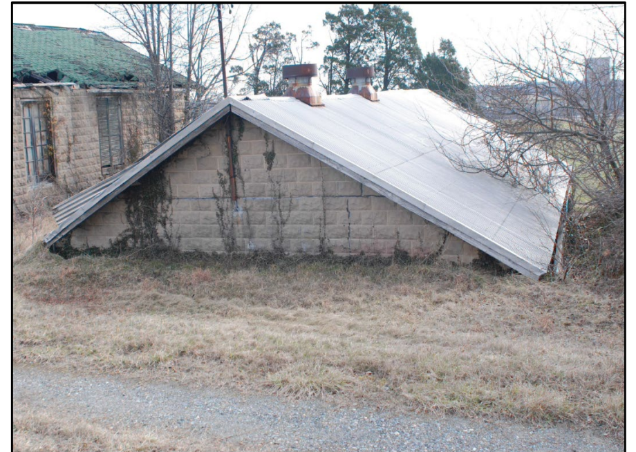
Photo 20: Building 0040, west elevation; photograph courtesy of Mark Edwards and Brian Clevon, 2016
