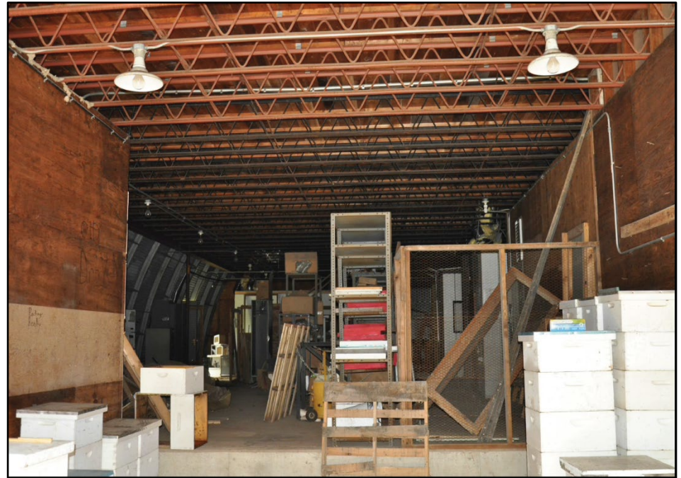
Photo 253: Building 0470B, view of interior; photograph courtesy of Brian Clevon, 2017.
