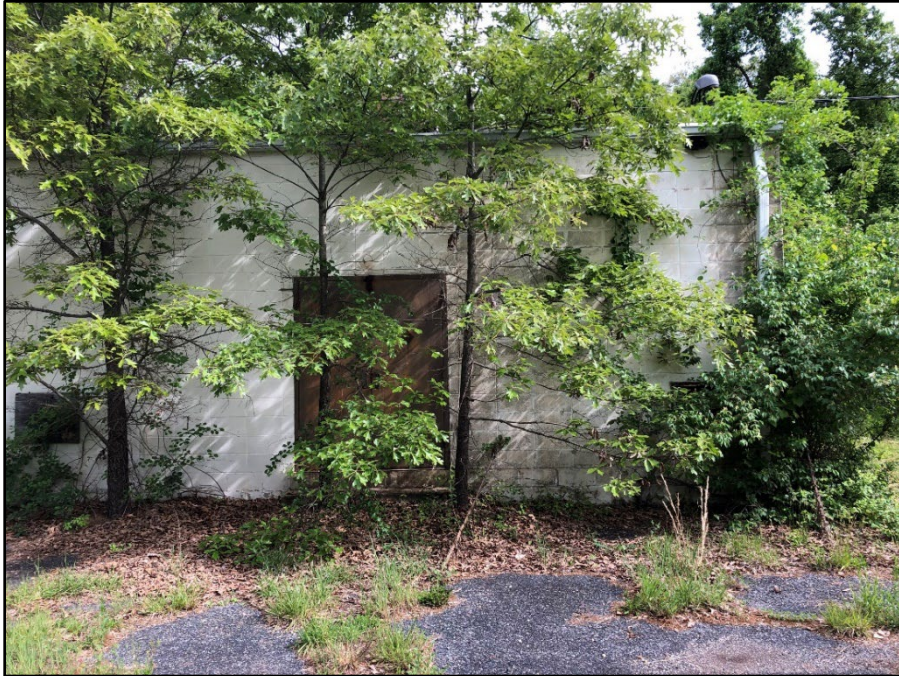
Photo 61: Building 0288, western elevation
