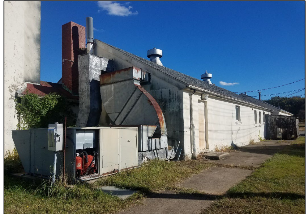
Photo 312: Building 1002, equipment on north elevation
