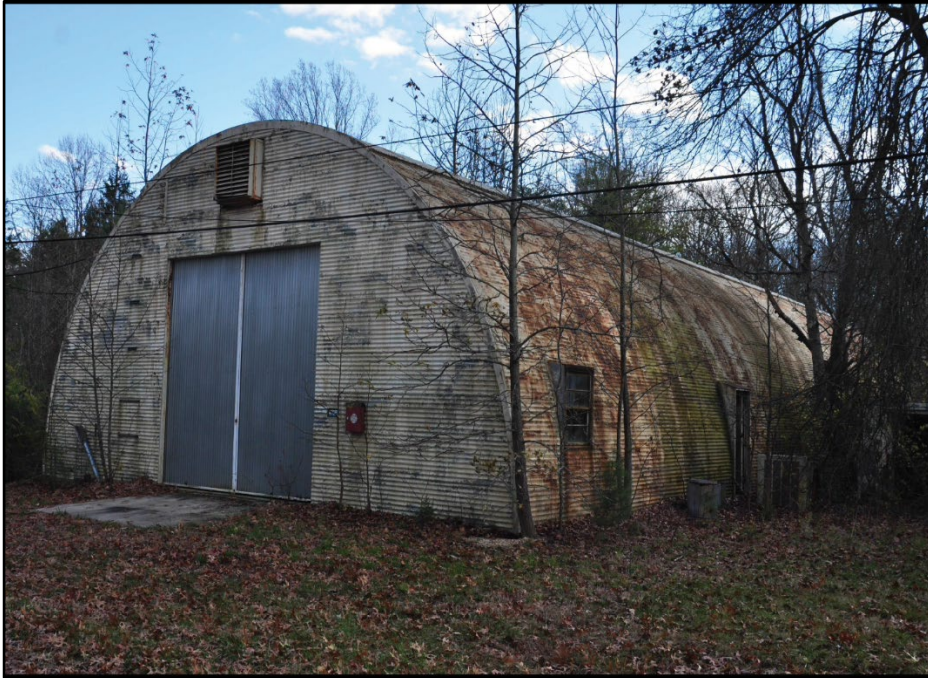
Photo 250: Building 0470B, north and west elevations; photograph courtesy of Brian Clevon, 2017.
