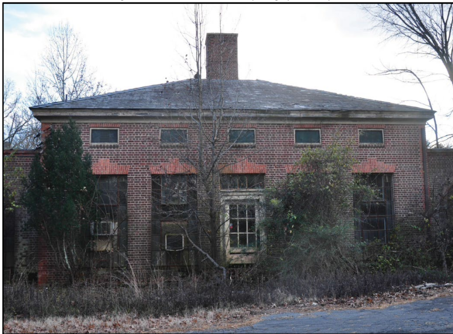
Photo 244: Building 0470, north elevation; photograph courtesy of Brian Clevin, 2017.
