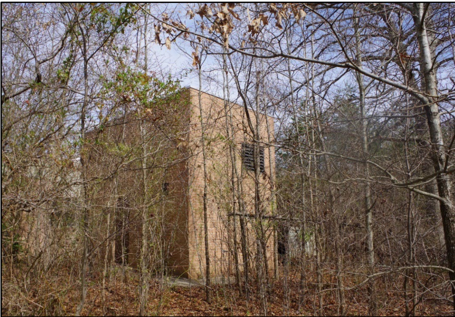
Photo 156: Building 339F, rear equipment
