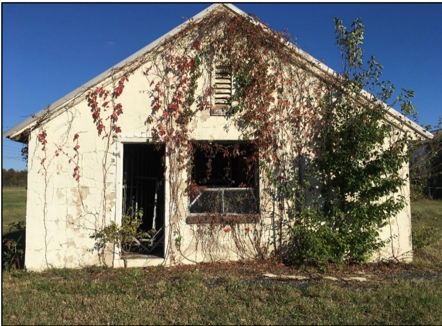
Photo 397: Building 1292, west elevation
