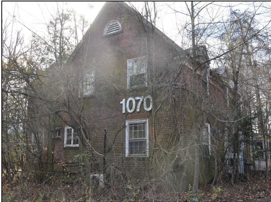
Photo 341: Building 1070, east elevation; photograph courtesy of Brian Clevon, 2017
