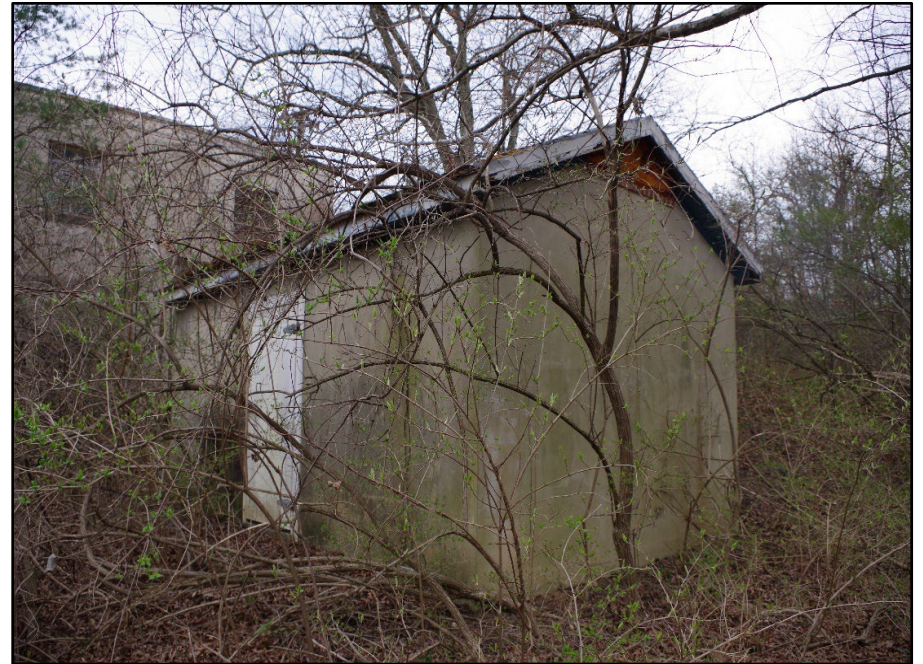
Photo 90: Building 0324A, north elevation
