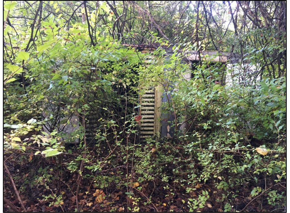
Photo 282: Building 0488, north elevation
