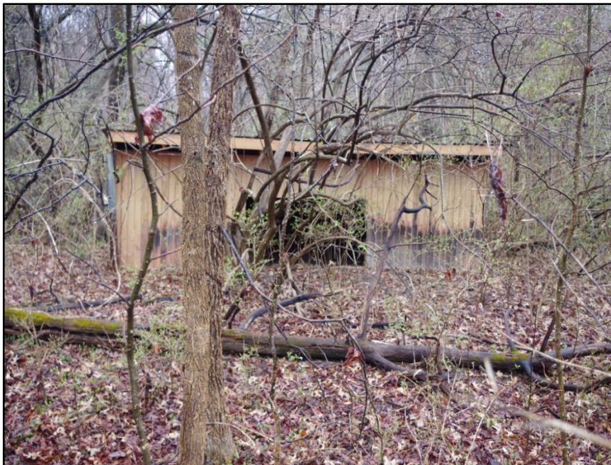
Photo 167: Building 0342B, overview
