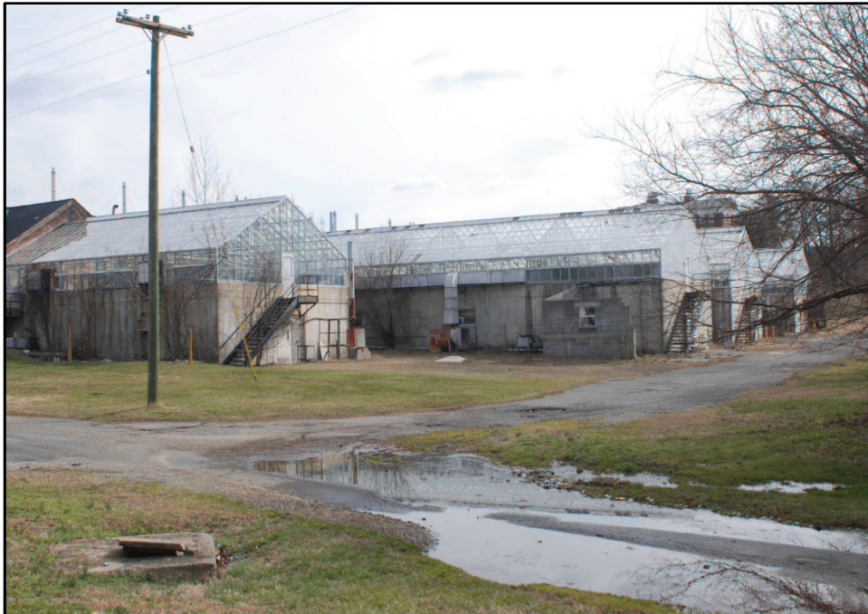
Photo 30: Building 0050, west and south elevations; photograph courtesy of Mark Edwards and Brian Clevin, 2016
