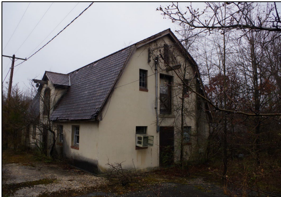
Photo 160: Building 0340, south elevation
