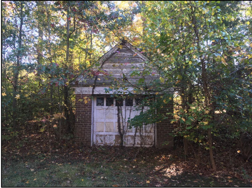
Photo 355: Building 1073, north elevations
