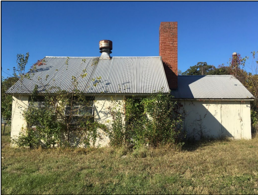
Photo 395: Building 1292, south elevation
