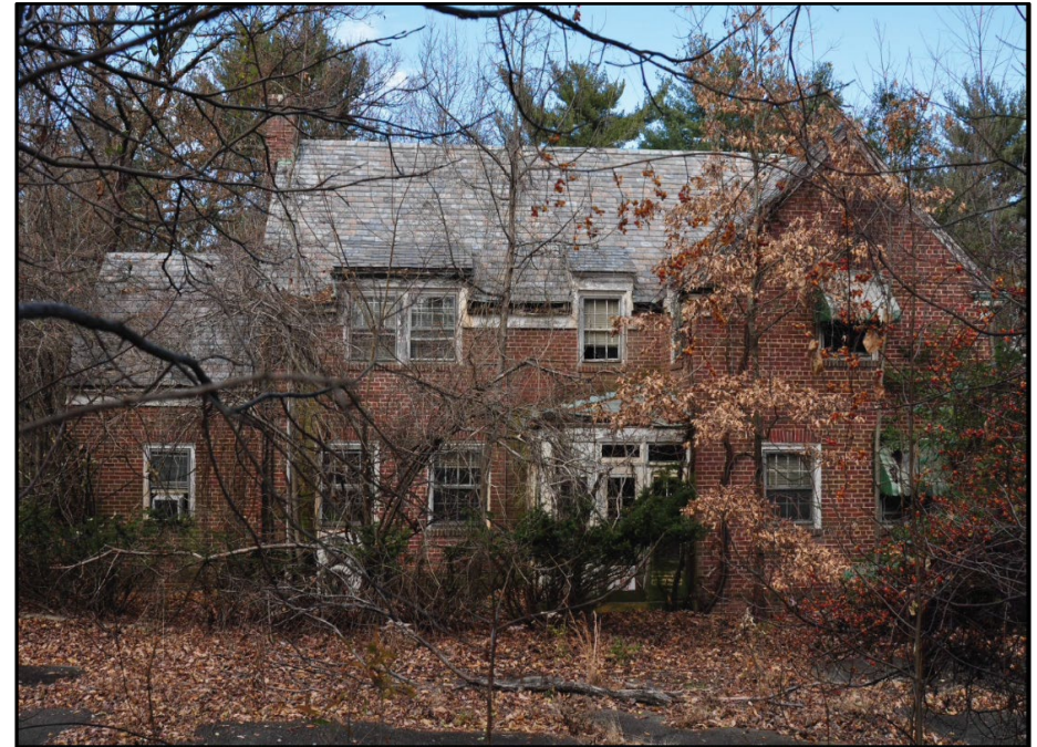
Photo 342: Building 1070, south elevation; photograph courtesy of Brian Clevon, 2017
