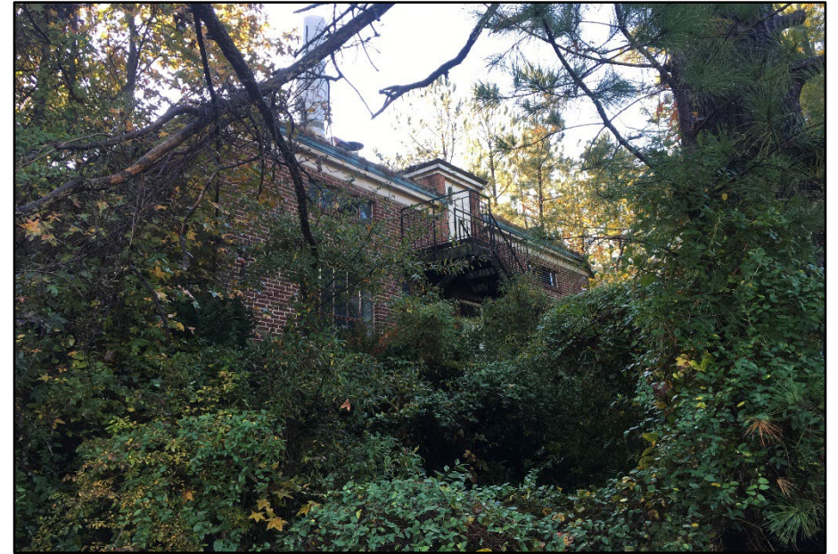
Photo 230: Building 0467, west elevation
