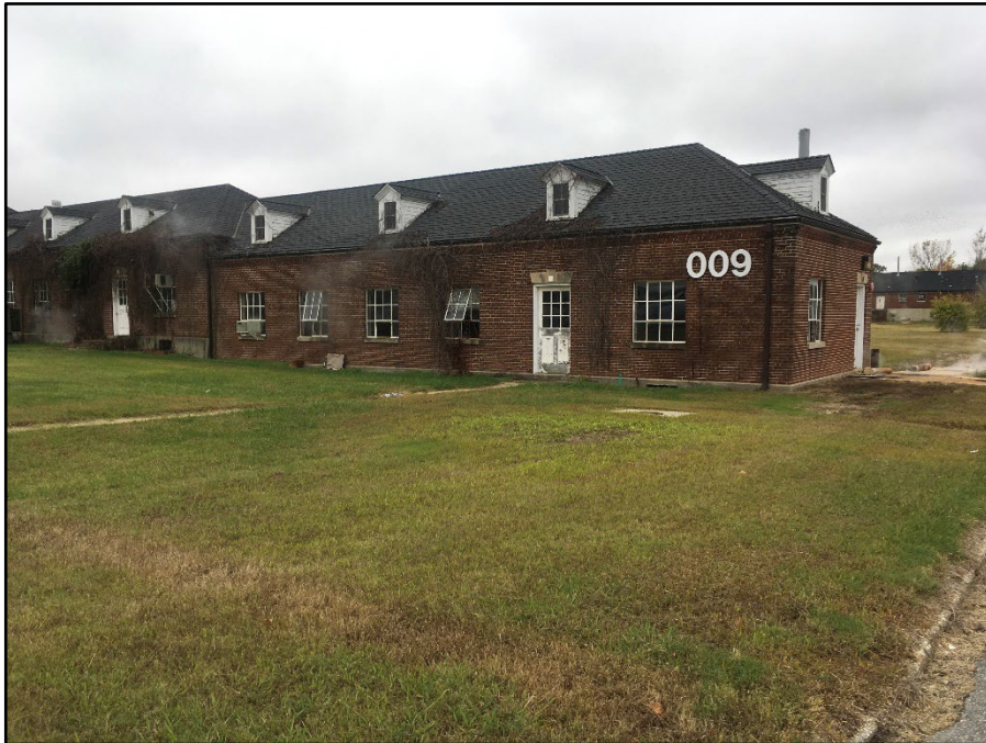
Photo 01: Building 0009, northwest elevation
