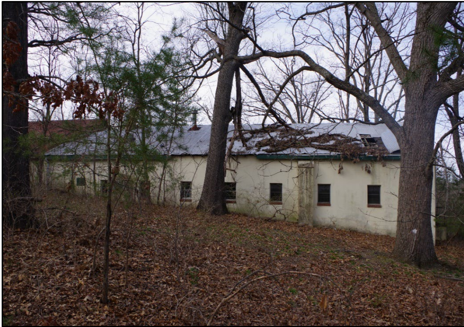
Photo 69: Building 0321, south elevation
