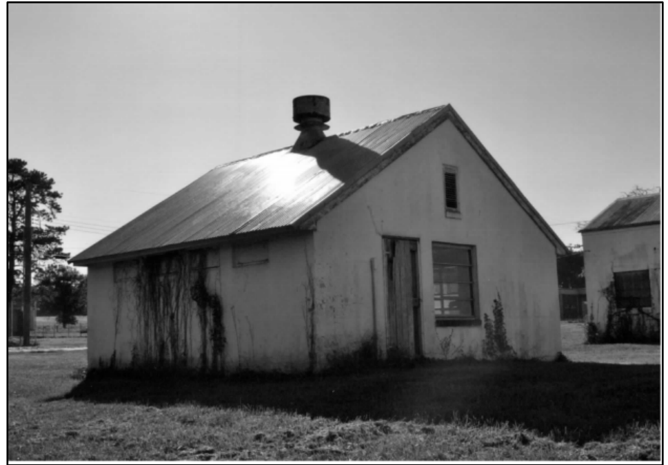
Photo 392: Building 1289, north and west elevations; photograph courtesy of Brian Cleven, 2017
