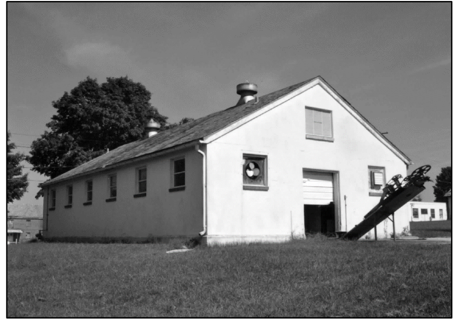
Photo 332: Building 1063, west and south elevations; photograph courtesy of Brian Clevon, 2017
