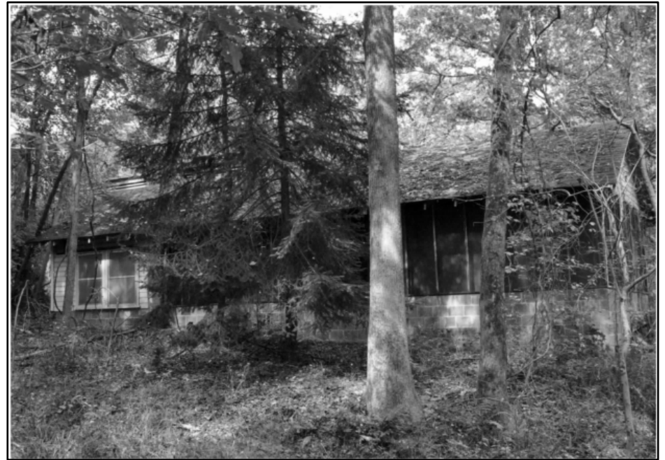
Photo 267: Building 0475, south elevation; photograph courtesy of Brian Clevon, 2017
