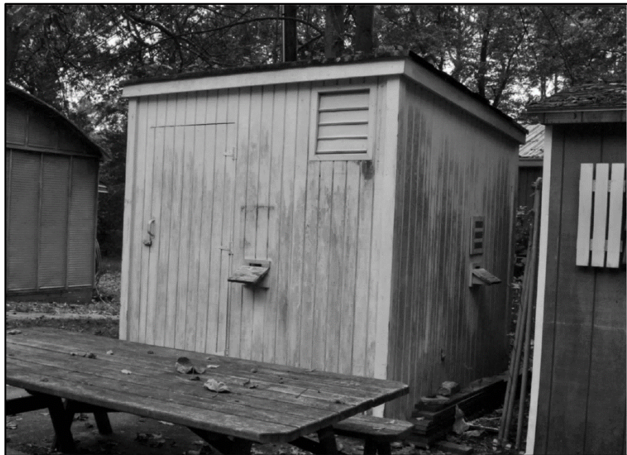
Photo 276: Building 0485, north and west elevations; photograph courtesy of Brian Clevon, 2017
