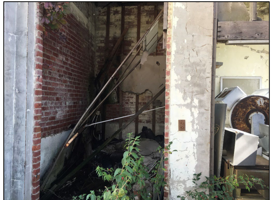
Photo 56: Building 0204A, interior
