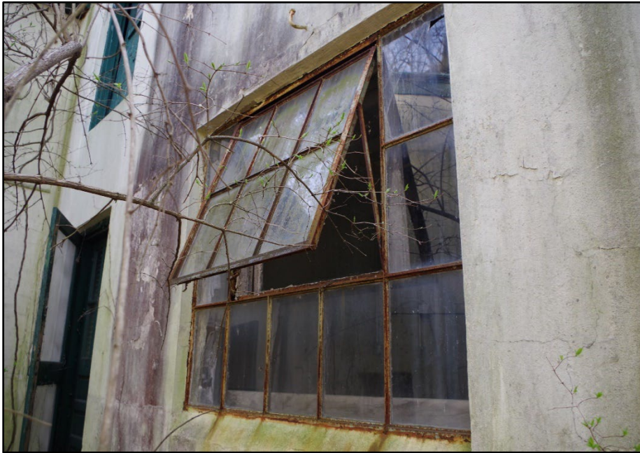
Photo 73: Building 0321, detail view of window
