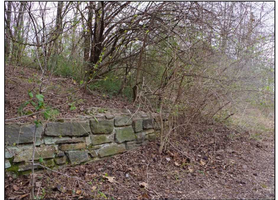
Photo 84: Building 0322, remaining stonewall
