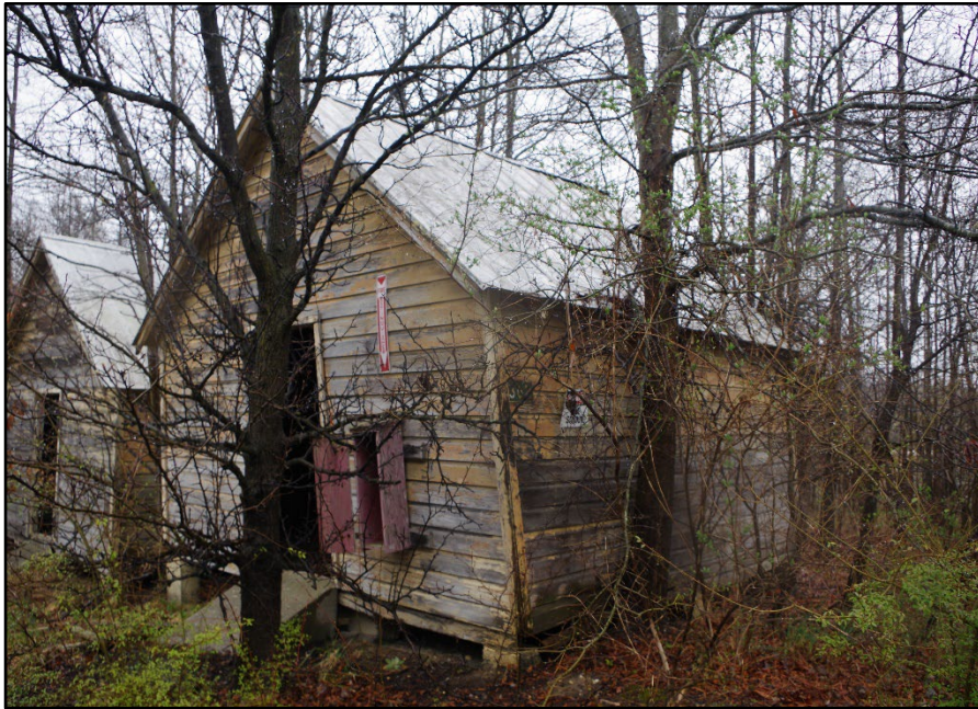
Photo 181: Building 0362, obstructed overview
