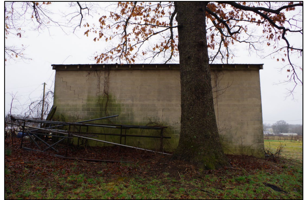
Photo 410: Building 1330, south elevation
