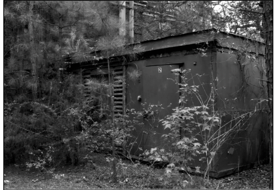
Photo 278: Building 0487-1, west and south elevations; photograph courtesy of Brian Clevon, 2017
