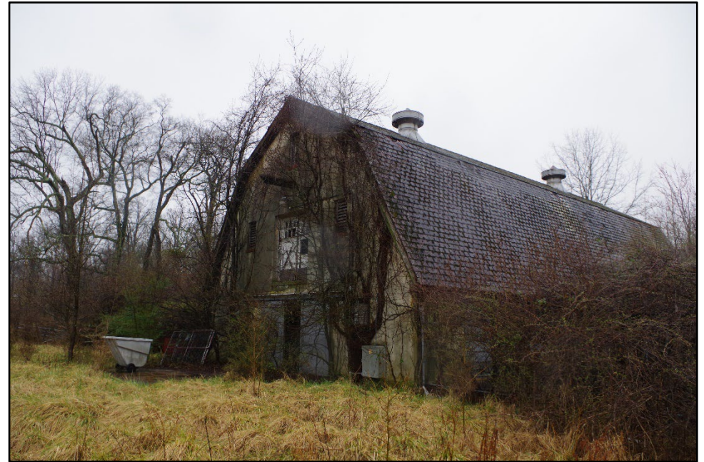
Photo 174: Building 0344, rear overview
