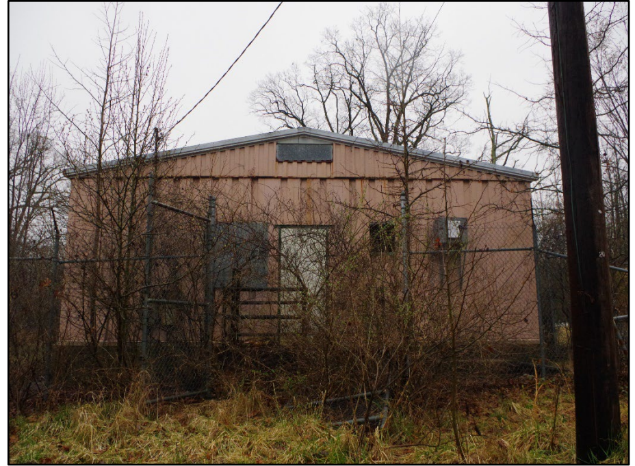
Photo 136: Building 0337A, north elevation
