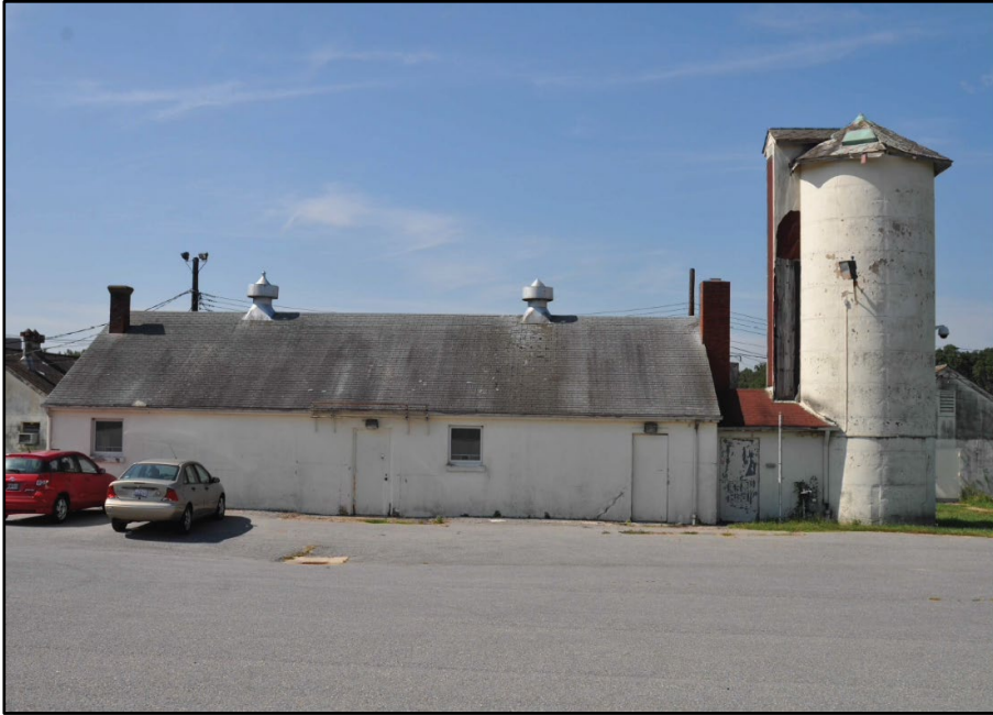
Photo 309: Building 1002, east elevation; photograph courtesy of Brian Clevin, 2017
