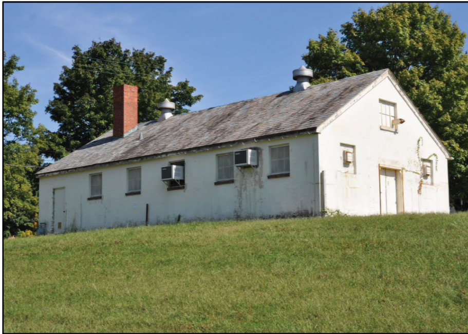
Photo 329: Building 1062, west and south elevations; photograph courtesy of Brian Clevin, 2017
