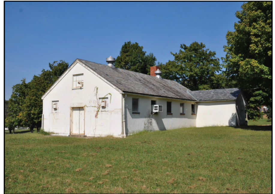
Photo 330: Building 1062, south and east elevations; photograph courtesy of Brian Clevin, 2017
