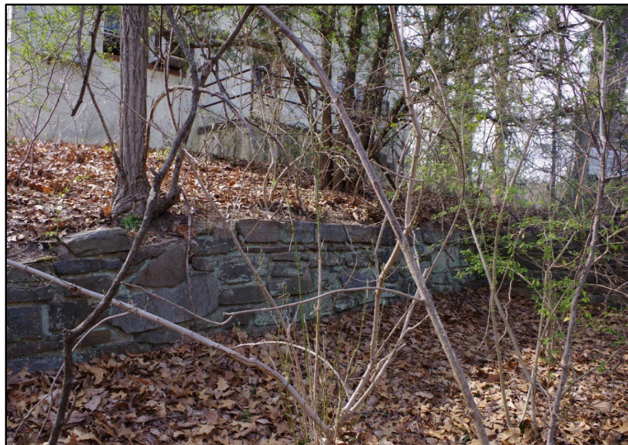
Photo 75: Building 0321, remaining stonewall
