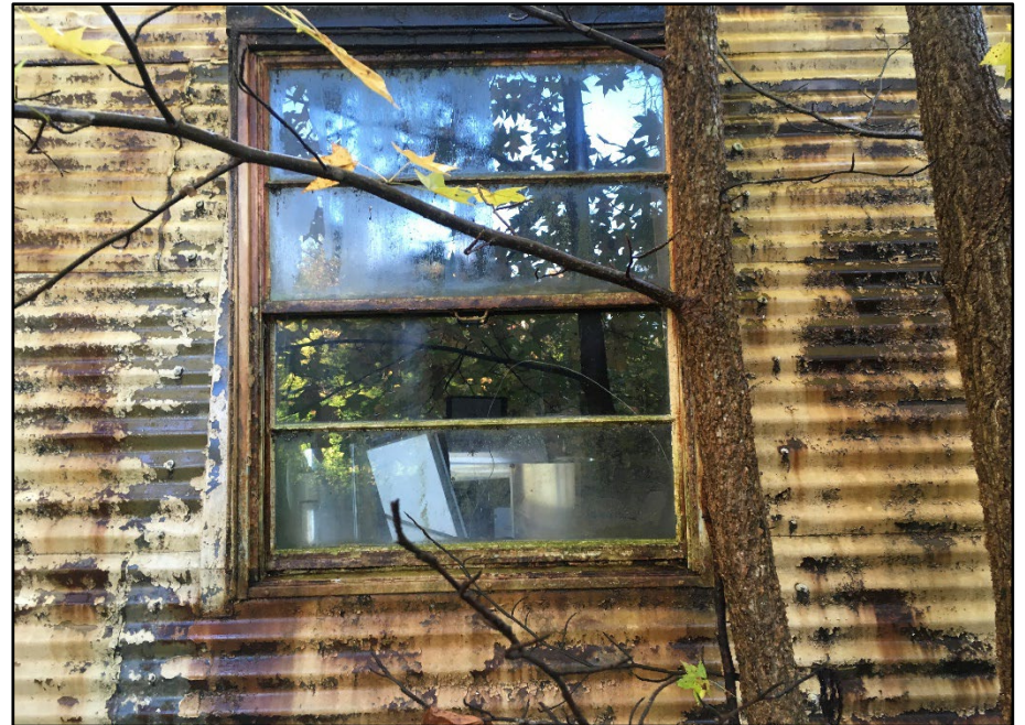
Photo 284: Building 0488, window detail
