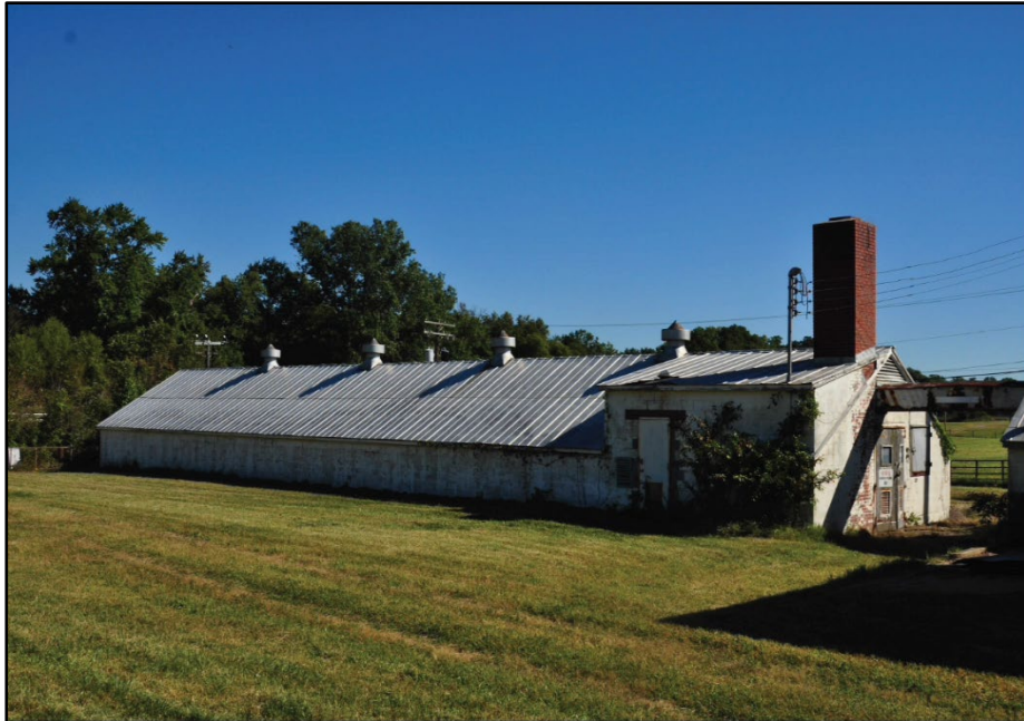
Photo 421: Building 1425, west and south elevations; photograph courtesy of Brian Clevin, 2017
