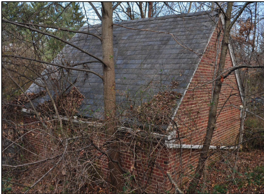
Photo 349: Building 1071, west and south elevations; photograph courtesy of Brian Cleven, 2017
