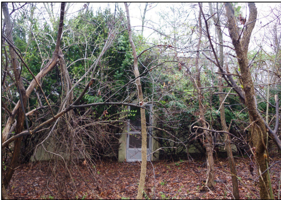
Photo 179: Building 0357, north elevation
