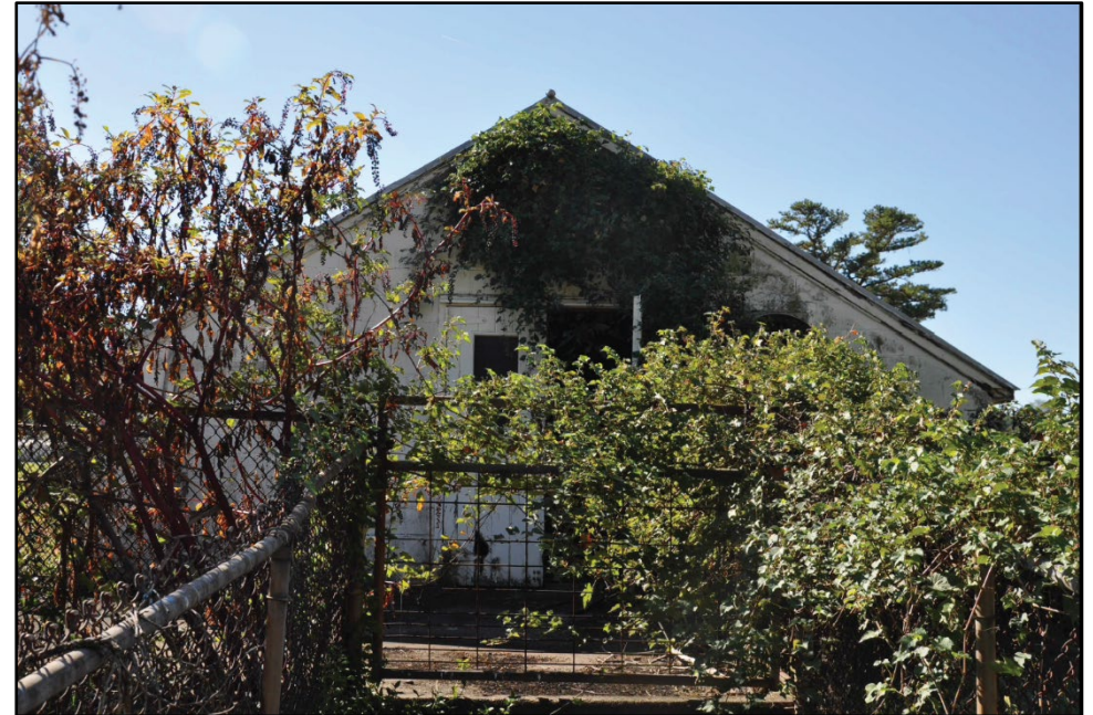
Photo 422: Building 1425, north elevation; photograph courtesy of Brian Clevin, 2017
