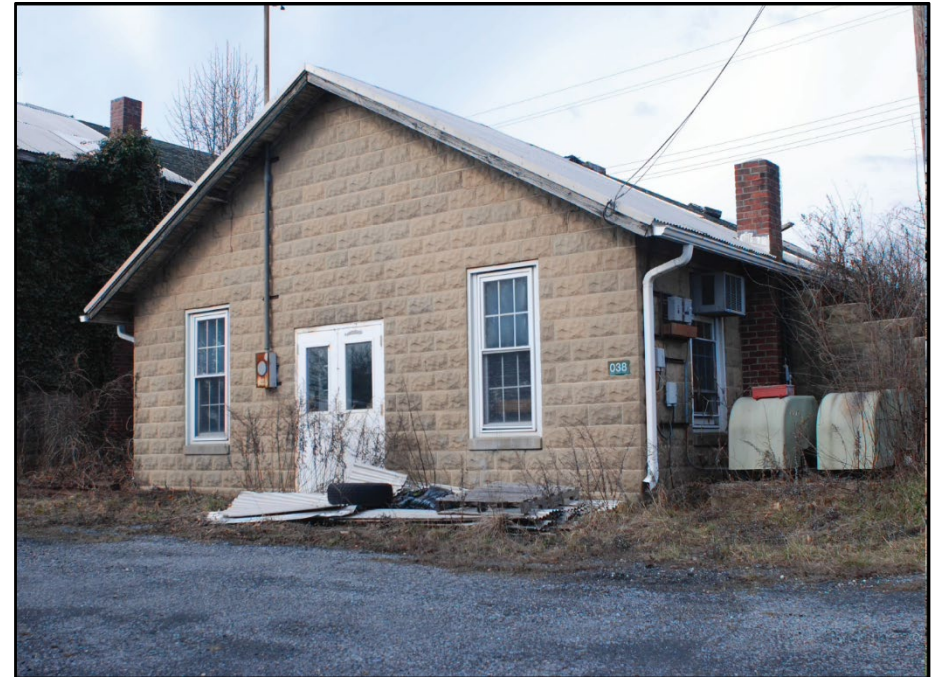
Photo 10: Building 0038, east elevation; photograph courtesy of Mark Edwards and Brian Clevon, 2016
