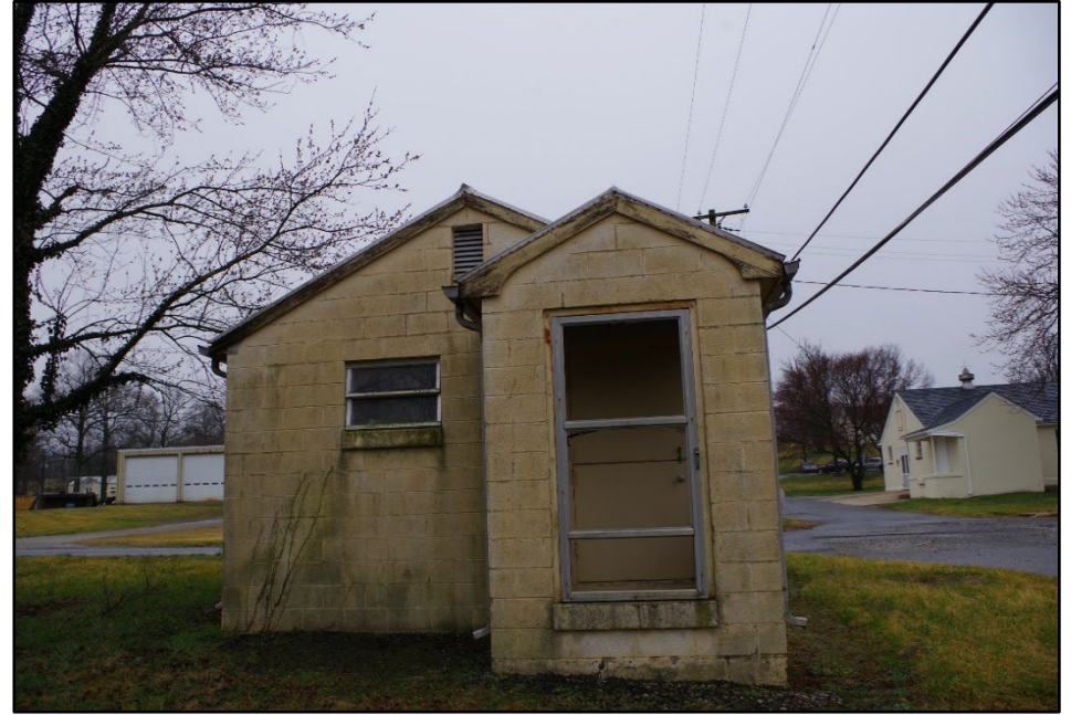
Photo 412: Building 1390, north elevation
