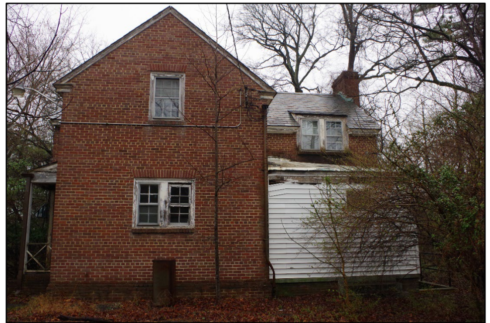
Photo 354: Building 1072, south elevation
