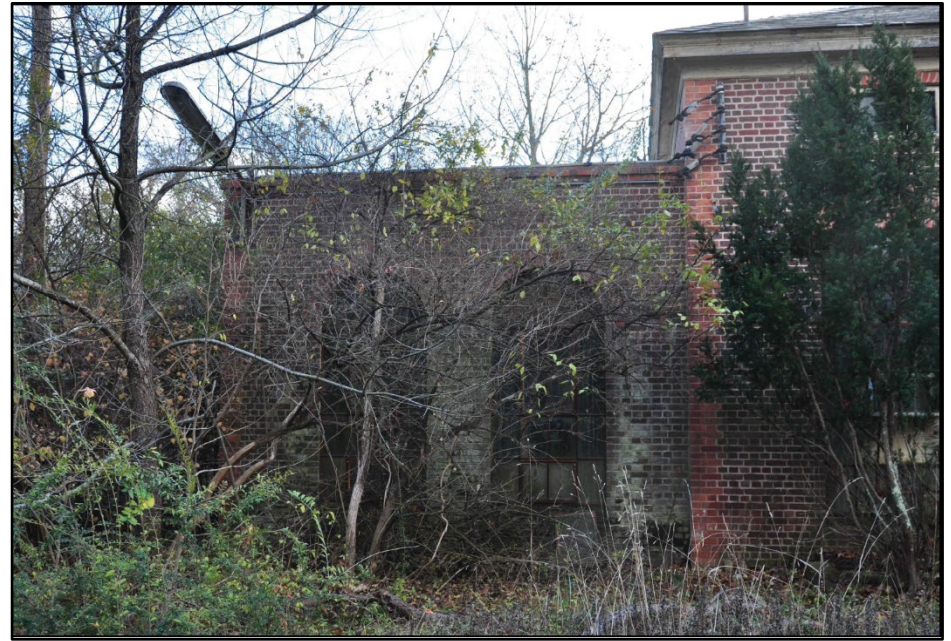
Photo 243: Building 0470, north elevation; photograph courtesy of Brian Clevin, 2017.
