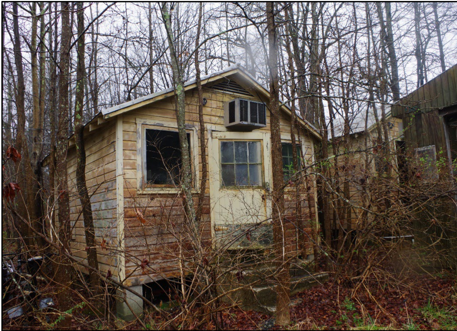
Photo 200: Building 0372, north elevation
