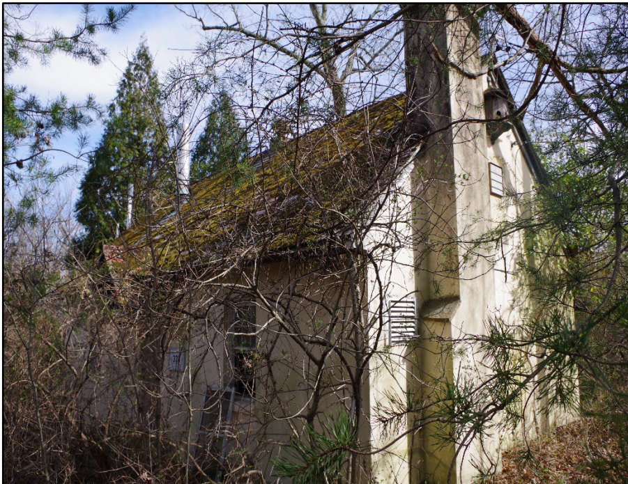
Photo 100: Building 0328, west and north elevations
