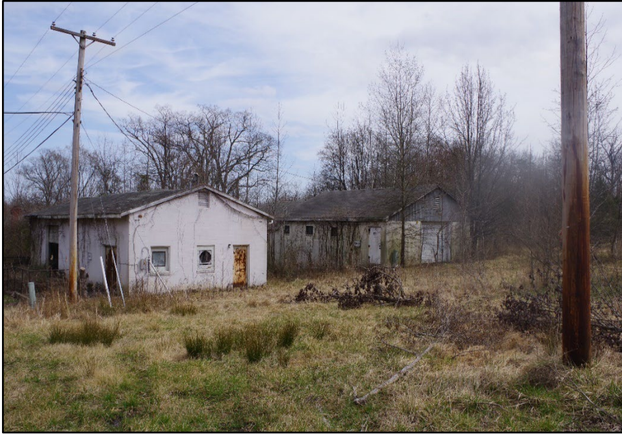
Photo 144: Building 0338A and 0338B, overview
