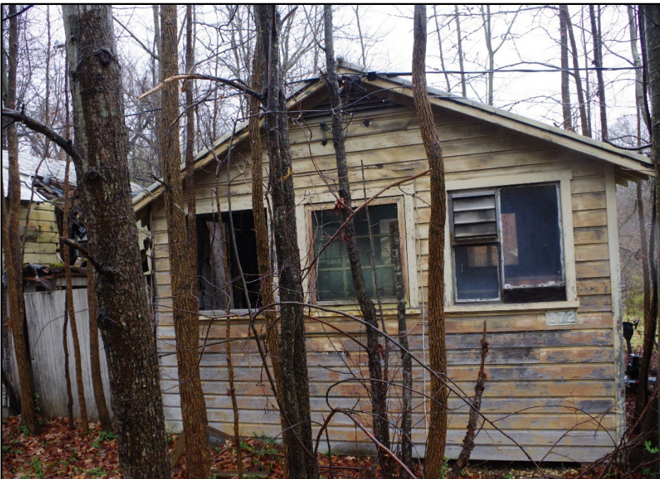
Photo 202: Building 0372, south elevation
