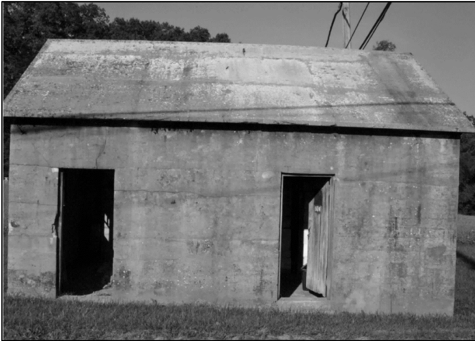
Photo 289: Building 0524, east elevation; photograph courtesy of Brian Clevon, 2017
