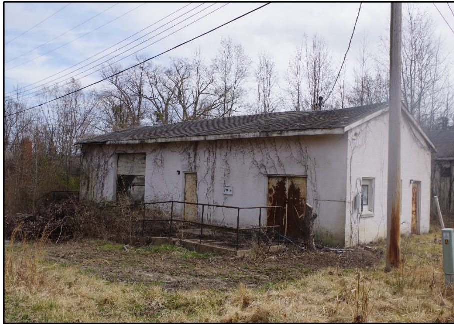
Photo 146: Building 0338A, north elevation
