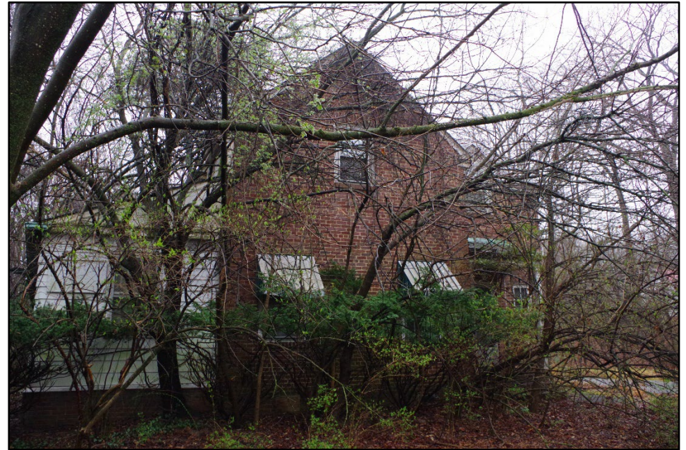
Photo 352: Building 1072, west elevation
