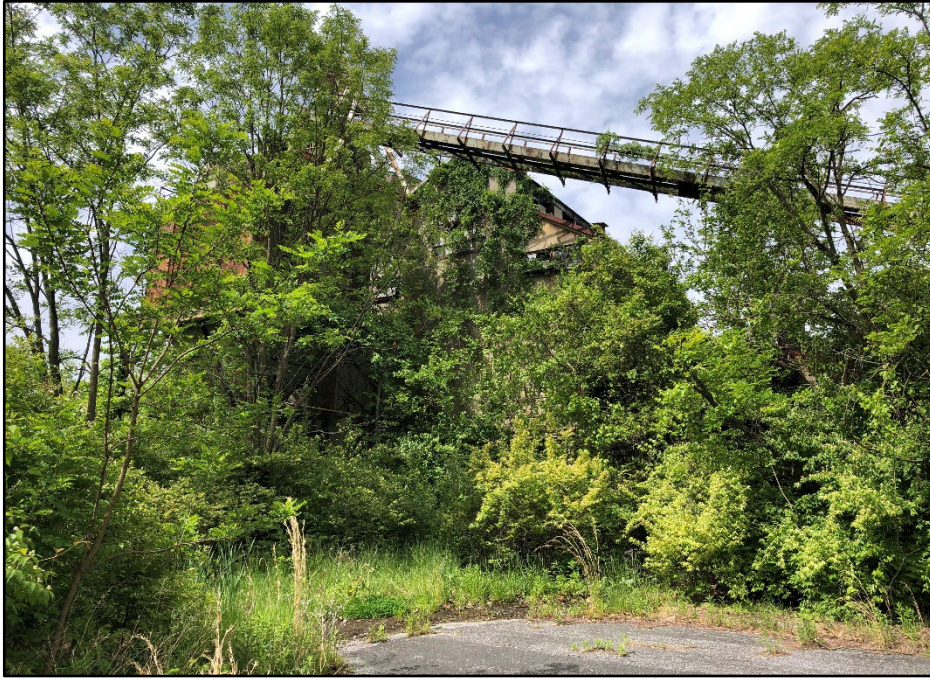
Photo 36: Building 0085, east elevation
