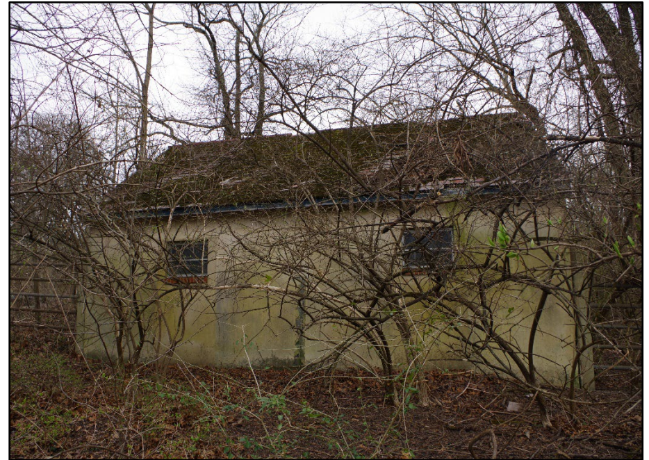
Photo 86: Building 0323, north elevation
