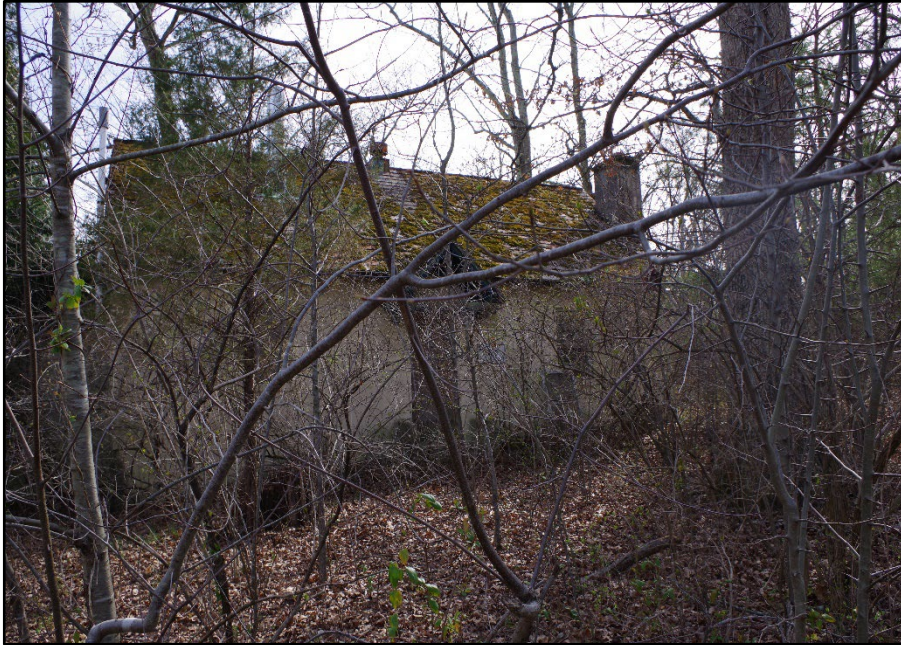
Photo 98: Building 0328, north elevation
