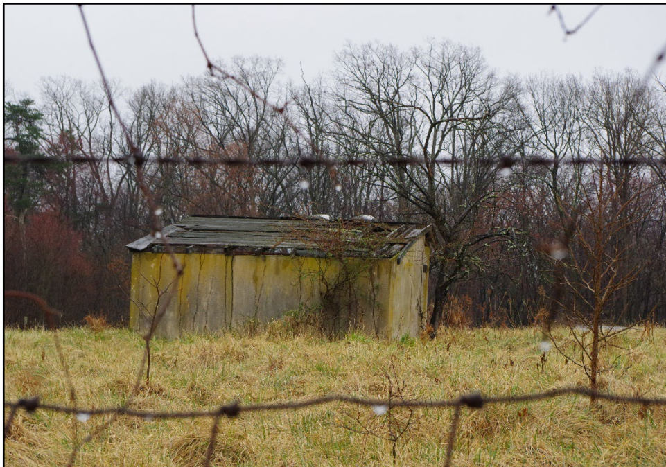
Photo 130: Building 0336C, north elevation
