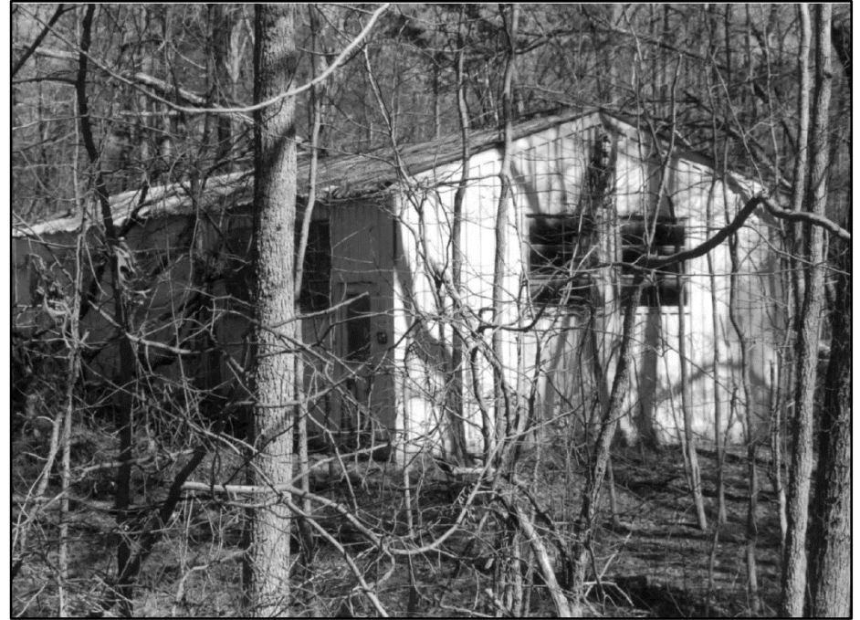
Photo 255: Building 0472, west and south elevations; photograph courtesy of Brian Clevon, 2017.
