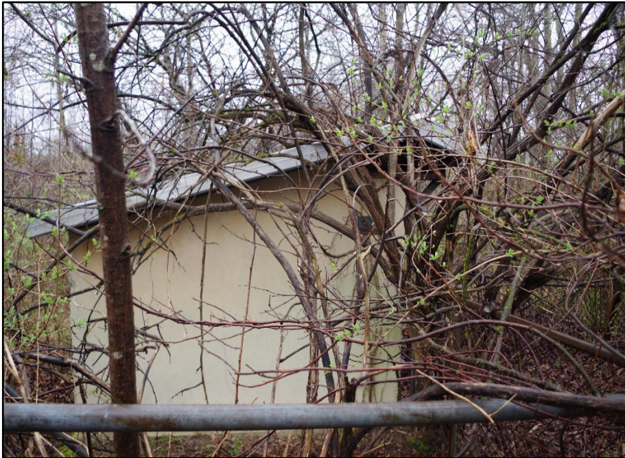
Photo 163: Building 0342, west elevation
