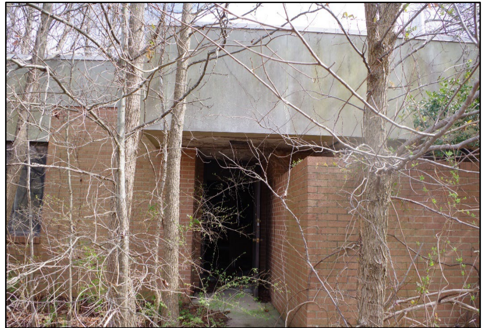
Photo 157: Building 339F, entrance
