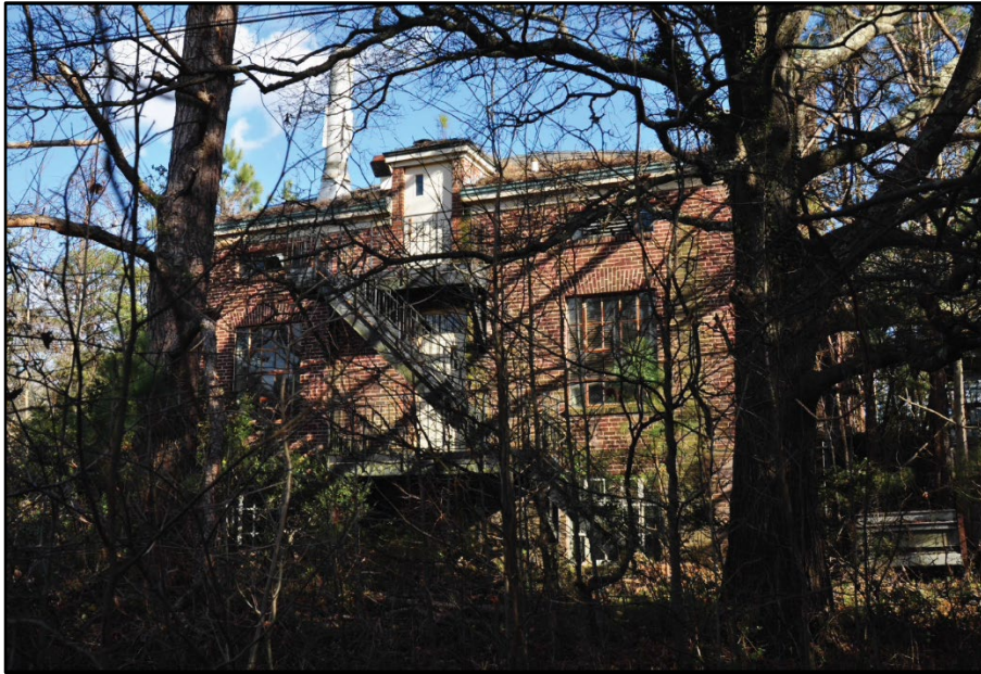
Photo 229: Building 0467, west elevation; photograph courtesy of Brian Clevon, 2017
