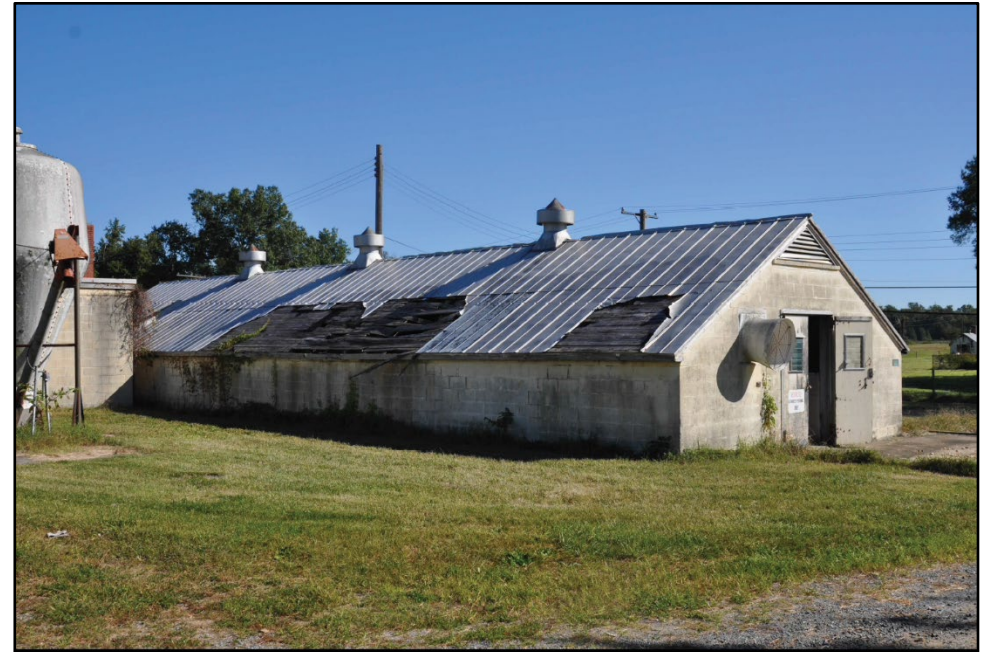
Photo 416: Building 1422, west and south elevations; photograph courtesy of Brian Clevin, 2017
