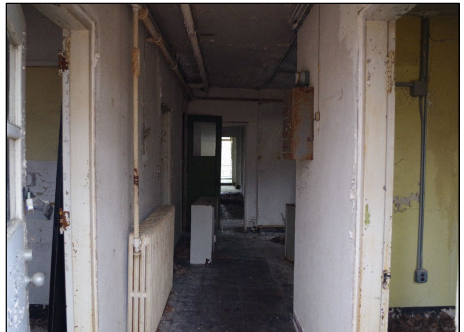
Photo 117: Building 0334, interior view
