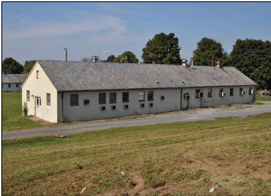
Photo 365: Building 1100, south and east elevations; photograph courtesy of Brian Clevon, 2017
