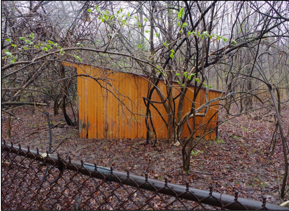
Photo 162: Building 0341R, obstructed overview
