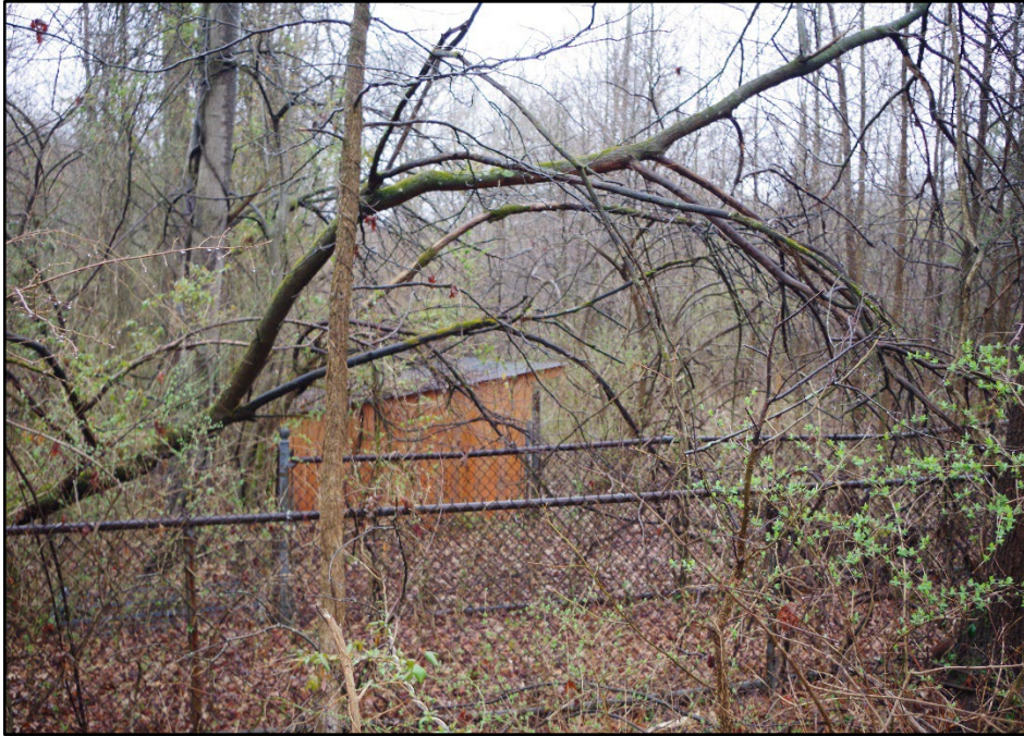
Photo 169: Building 0342C, obstructed overview
