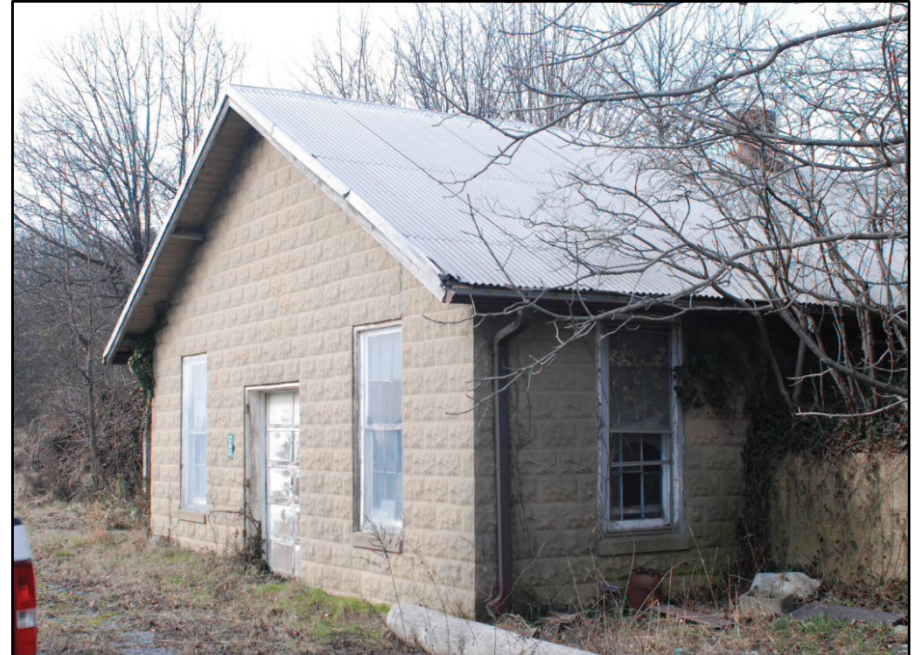
Photo 18: Building 0040, east and west elevations; photograph courtesy of Mark Edwards and Brian Clevon, 2016
