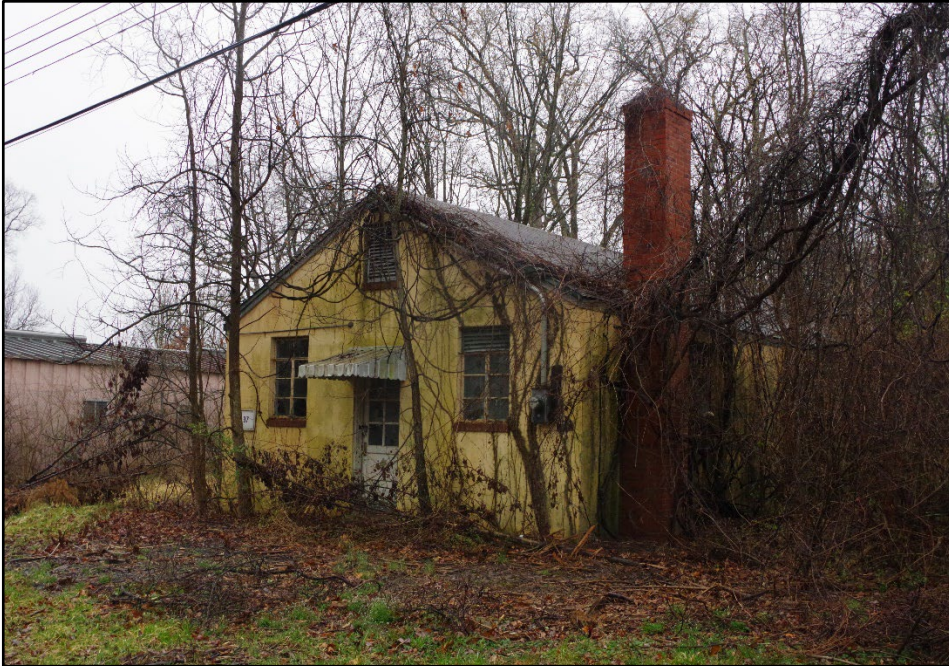
Photo 131: Building 0337, north elevation
