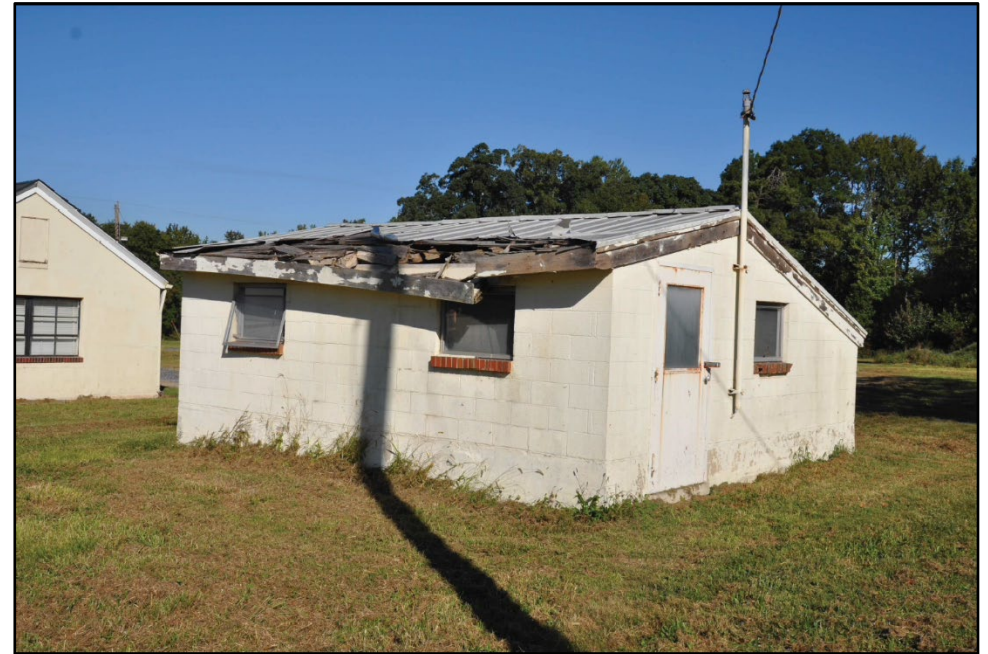
Photo 400: Building 1328, south and east elevations; photograph courtesy of Brian Clevon, 2017
