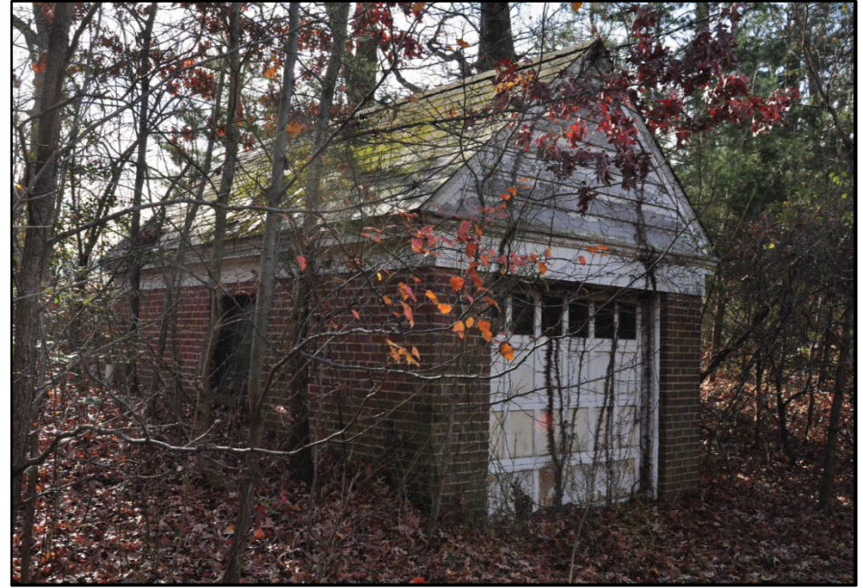
Photo 356: Building 1073, east and north elevations; photograph courtesy of Brian Clevon, 2017
