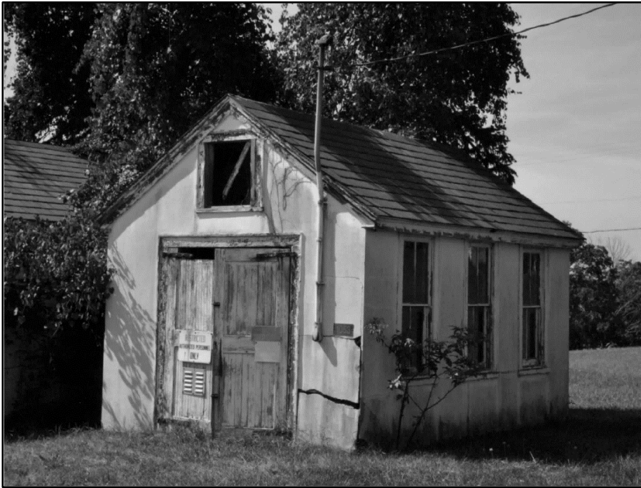
Photo 321: Building 1053, east and north elevations; photograph courtesy of Mark Edwards and Brian Clevon, 2016
