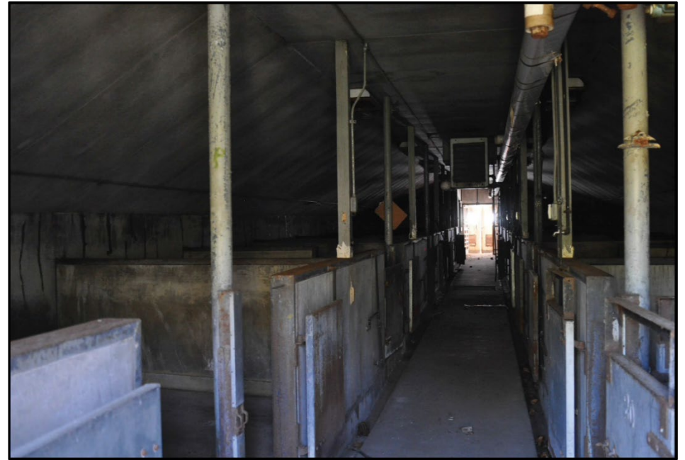
Photo 424: Building 1425; photograph courtesy of Brian Clevon, 2017
