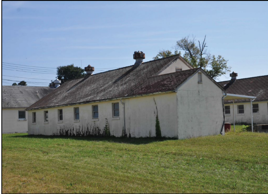
Photo 315: Building 1005, north and west elevations; photograph courtesy of Brian Clevon, 2017
