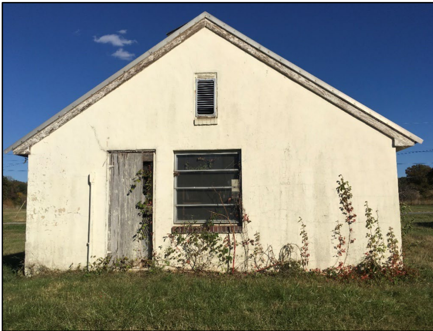
Photo 393: Building 1289, west elevation
