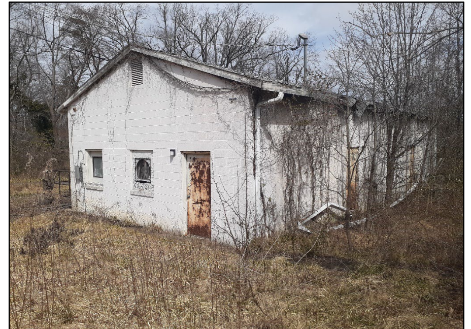
Photo 147: Building 0338A, north elevation
