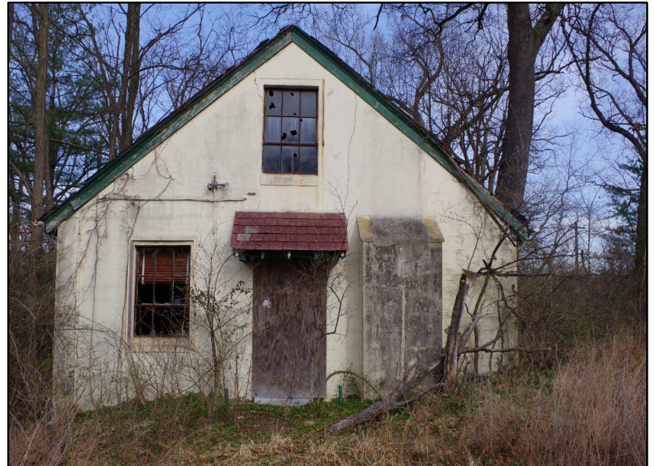
Photo 68: Building 0321, west elevation
