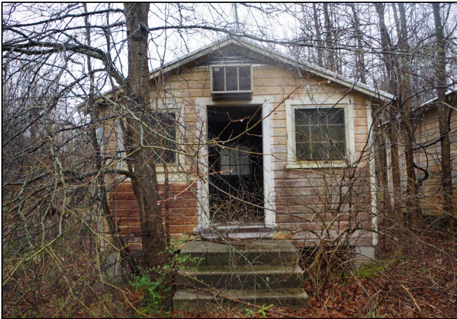
Photo 194: Building 0370, north elevation
