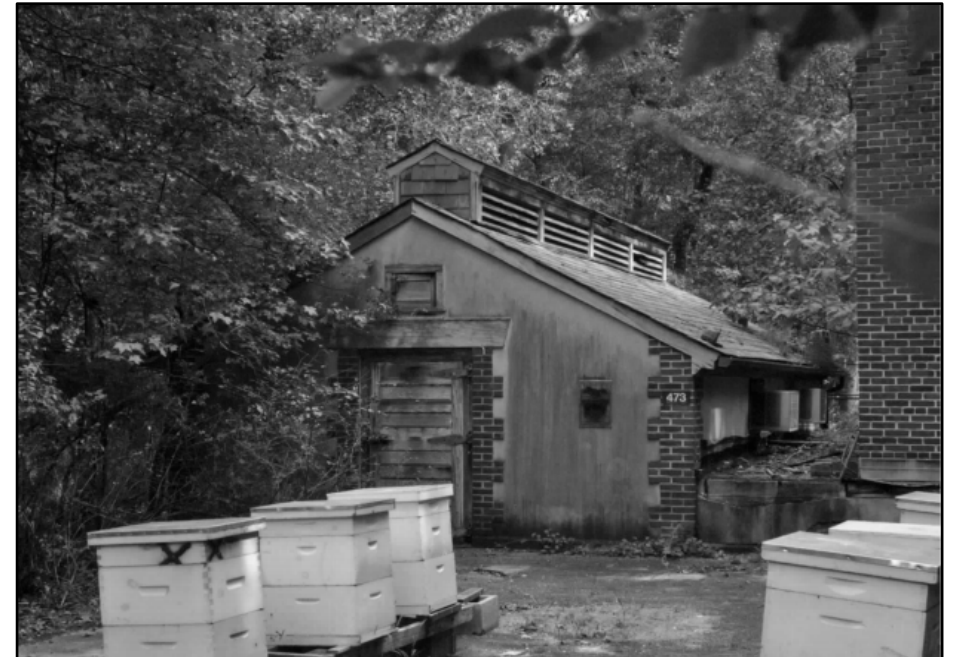
Photo 261: Building 0473, west and south elevations; photograph courtesy of Mark Edwards and Brian Clevon, 2016
