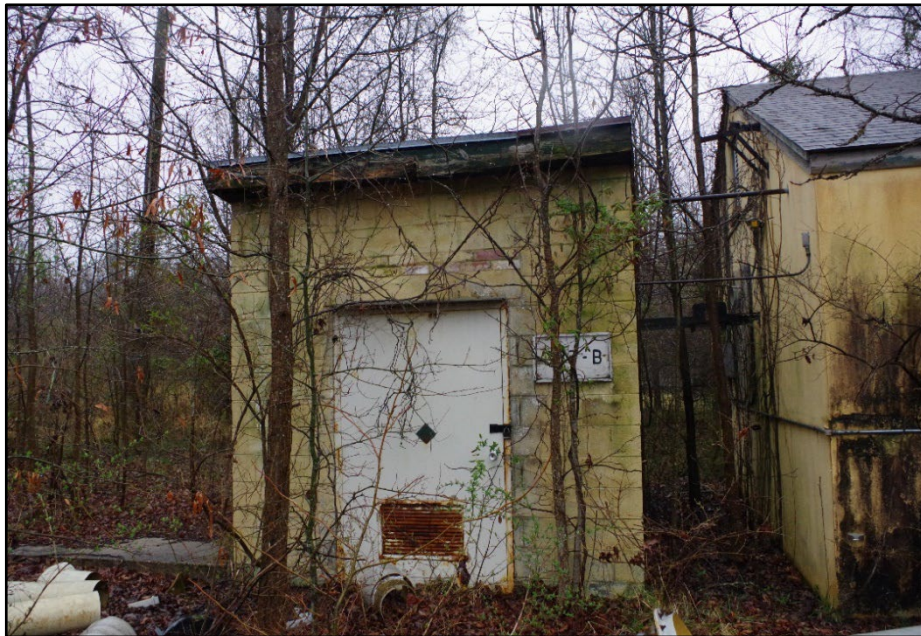
Photo 139: Building 0337B, east elevation
