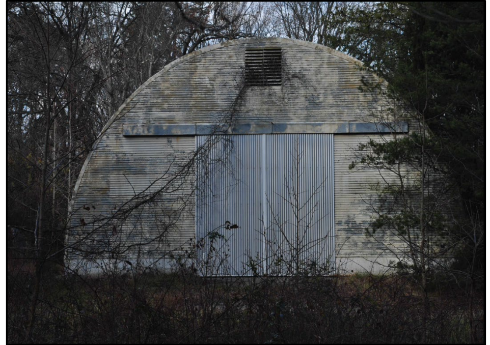
Photo 251: Building 0470B, south elevation; photograph courtesy of Brian Clevon, 2017.
