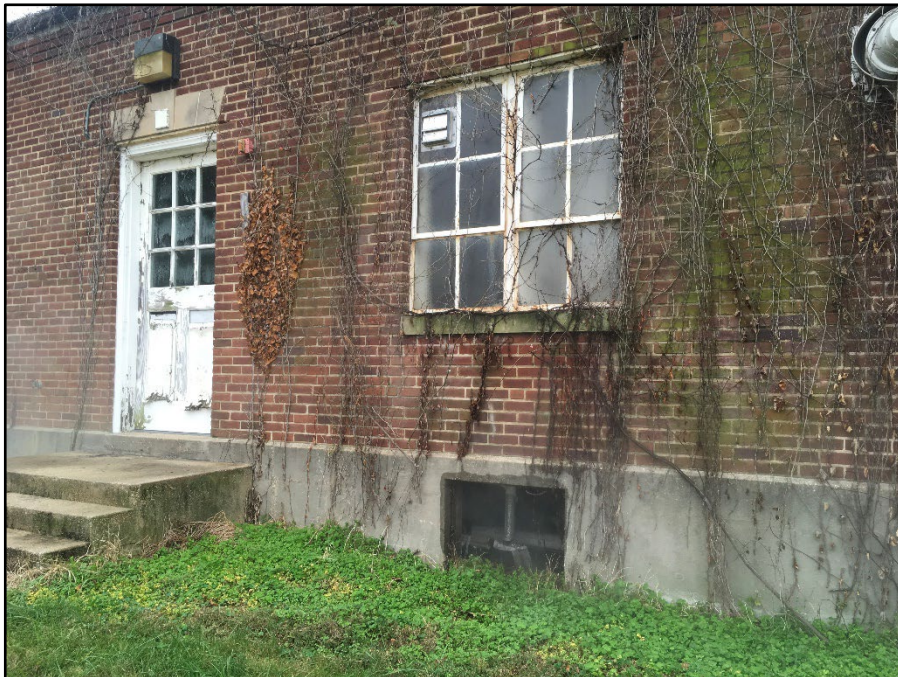
Photo 03: District Building 0009, entrance and window on northwest elevation
