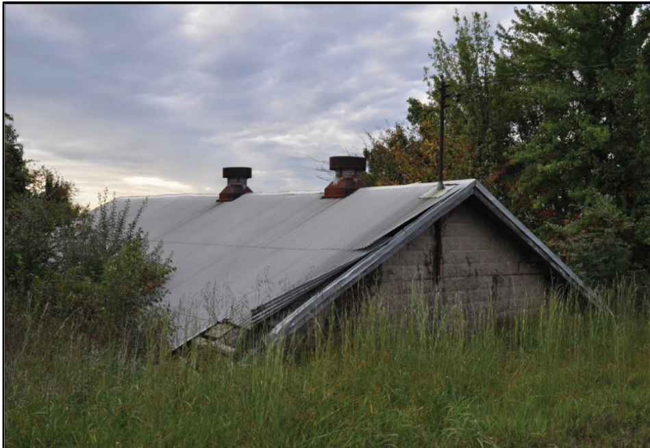
Photo 19: Building 0040, east and west elevations; photograph courtesy of Mark Edwards and Brian Clevon, 2016
