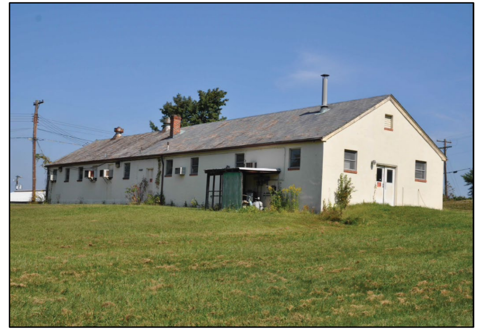
Photo 366: Building 1100, west and south elevations; photograph courtesy of Brian Clevon, 2017
