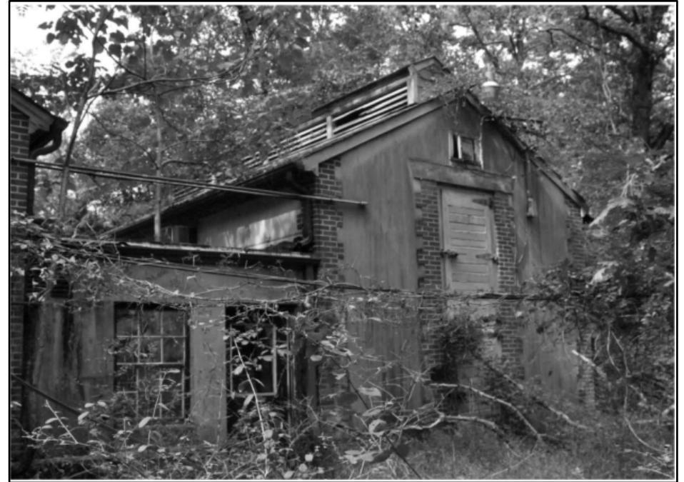
Photo 259: Building 0473, east elevation; photograph courtesy of Mark Edwards and Brian Clevon, 2016
