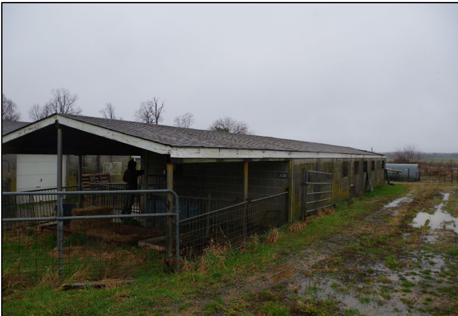
Photo 51: Building 0203B, northern elevation
