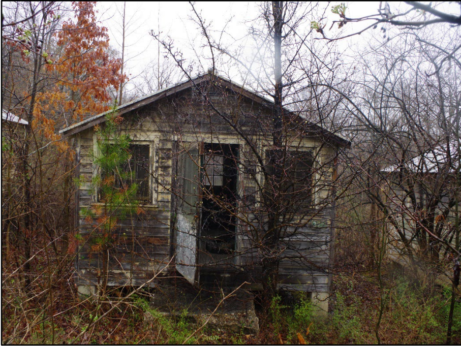
Photo 207: Building 0375, south elevation
