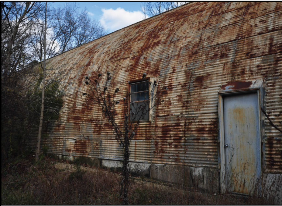
Photo 252: Building 0470B, west elevation; photograph courtesy of Brian Clevon, 2017.
