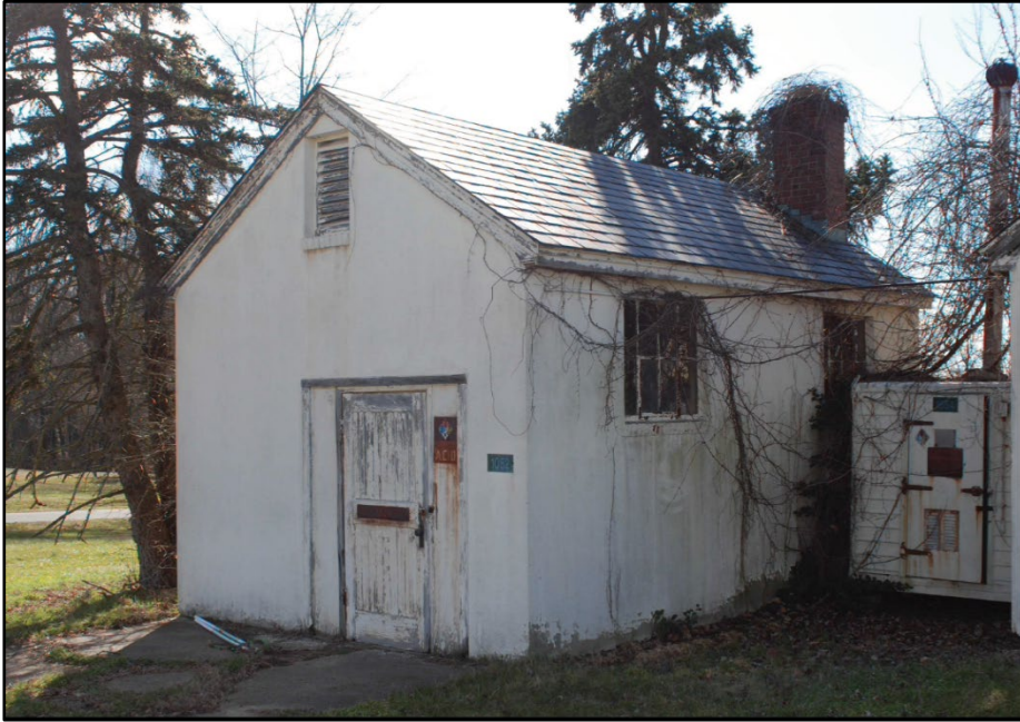
Photo 317: Building 01052, east and north elevations; photograph courtesy of Mark Edwards and Brian Clevon, 2016
