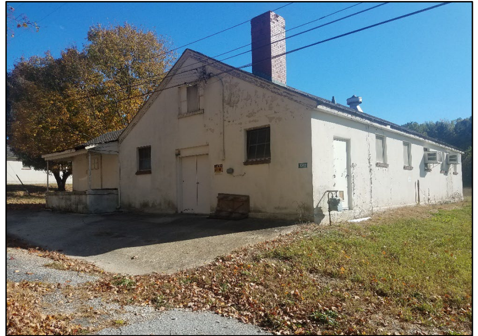
Photo 328: Building 1062, north and west elevations
