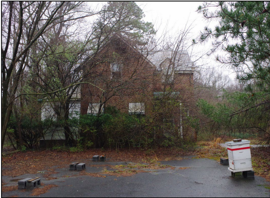
Photo 351: Building 1072, west elevation and beehives
