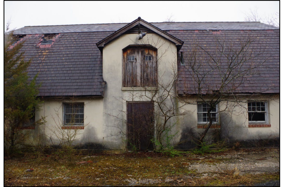
Photo 159: Building 0340, west elevation
