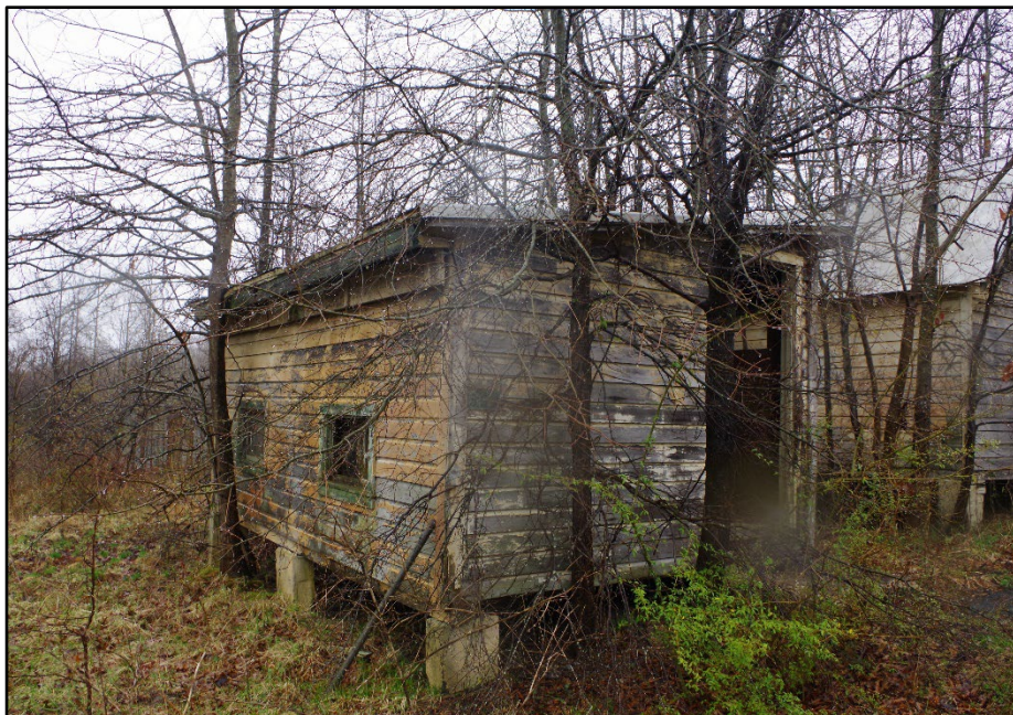
Photo 187: Building 0364, west elevation
