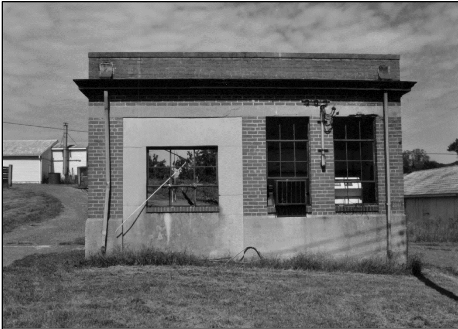
Photo 53: Building 0204A, south elevation; photograph courtesy of Brian Clevon, 2017
