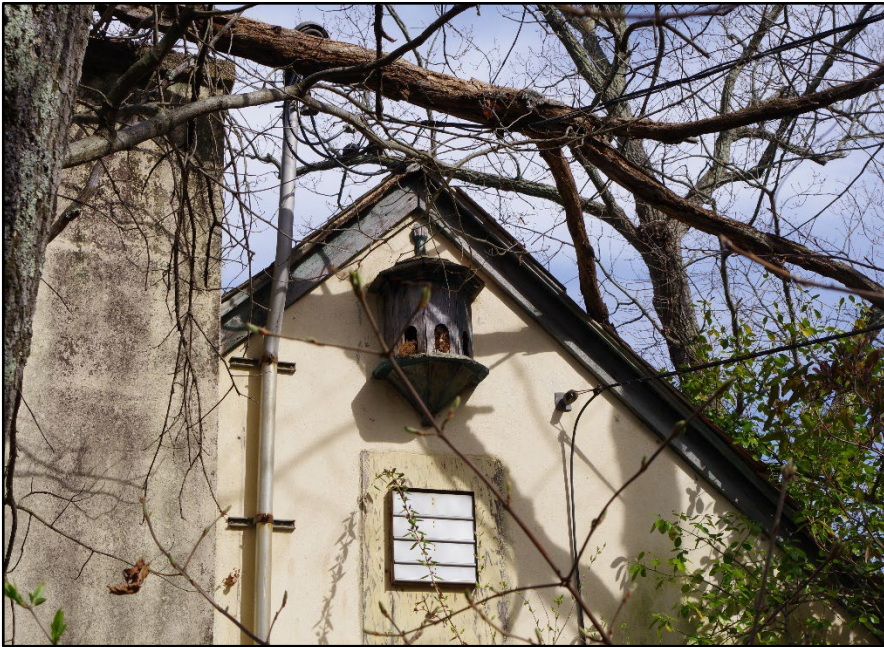
Photo 102: Building 0328, birdhouse dormer on west elevation
