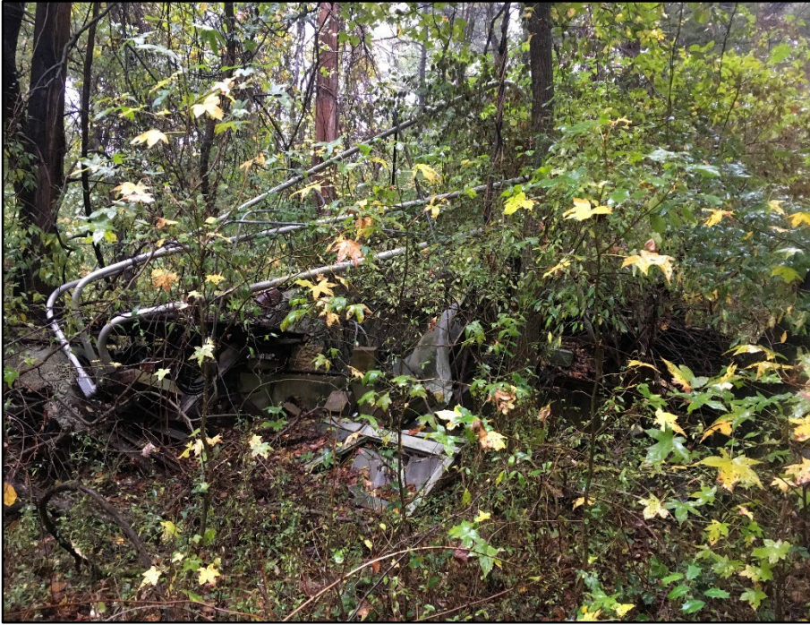
Photo 223: Building 0452, west elevation
