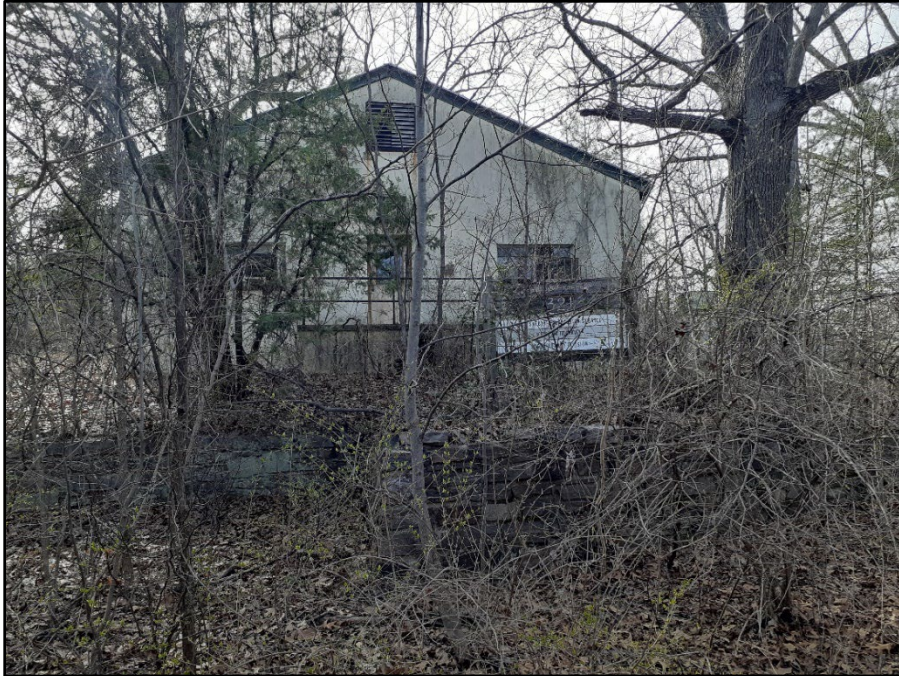
Photo 65: Building 0321, overview of east elevation
