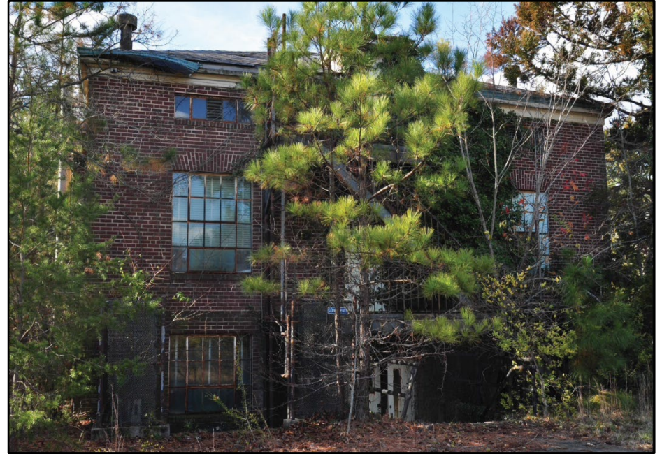
Photo 232: Building 0467, east elevation; photograph courtesy of Brian Clevon, 2017
