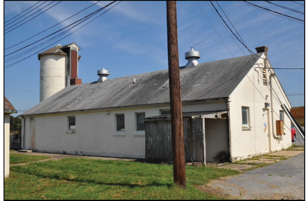
Photo 310: Building 1002, west and south elevations; photograph courtesy of Brian Clevin, 2017
