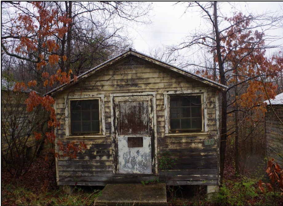
Photo 209: Building 0376, south elevation
