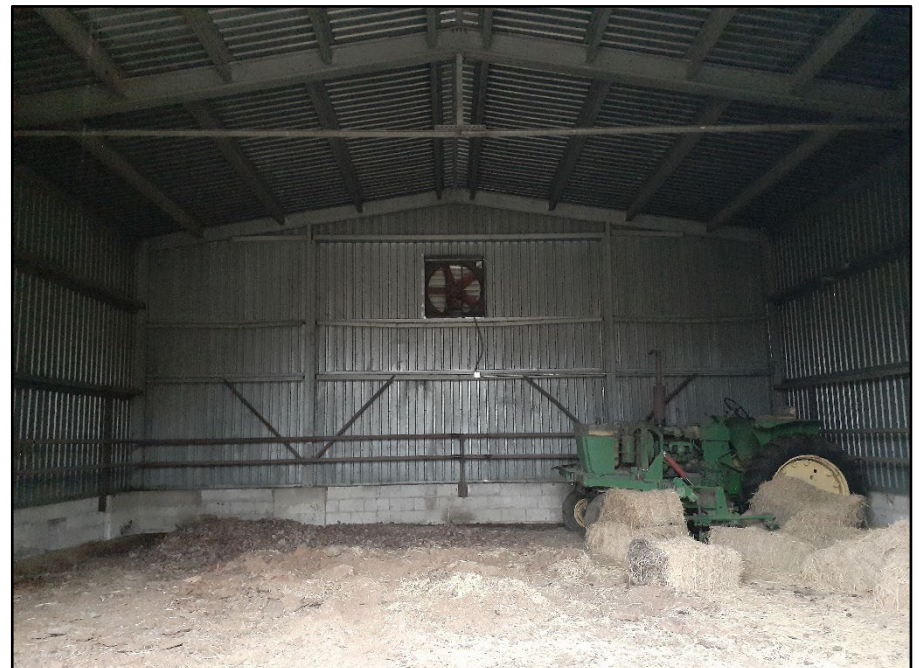
Photo 127: Building 0335B, interior
