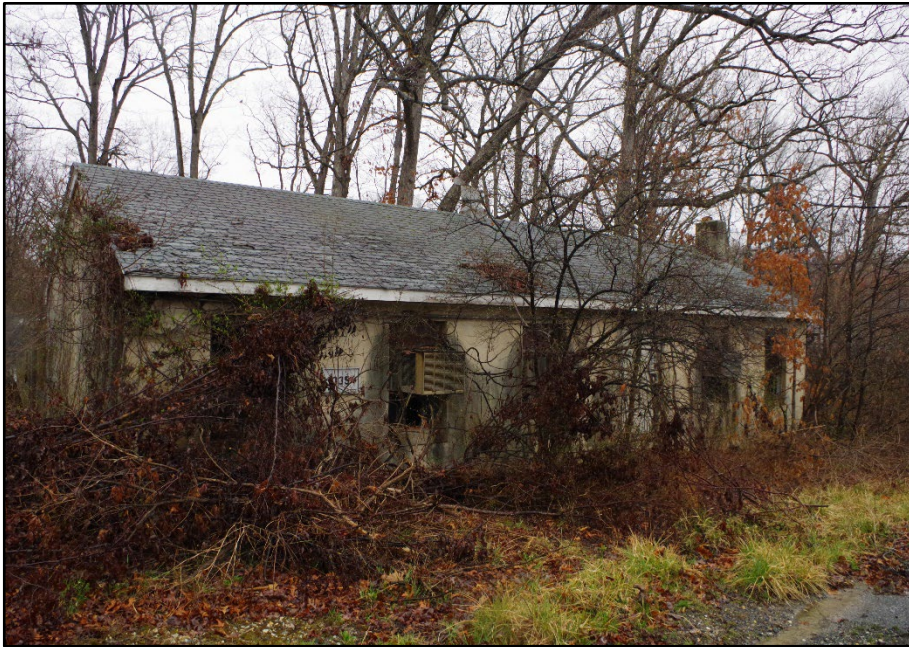
Photo 118: Building 0335, south elevation
