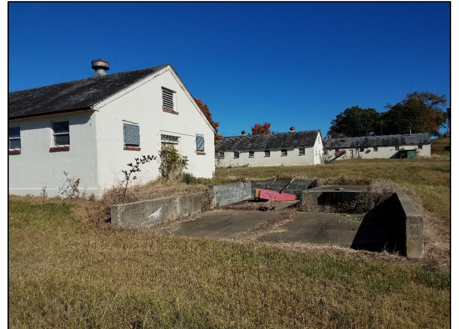
Photo 338: Building 1064, camera facing east; photograph courtesy of Brian Clevon, 2017
