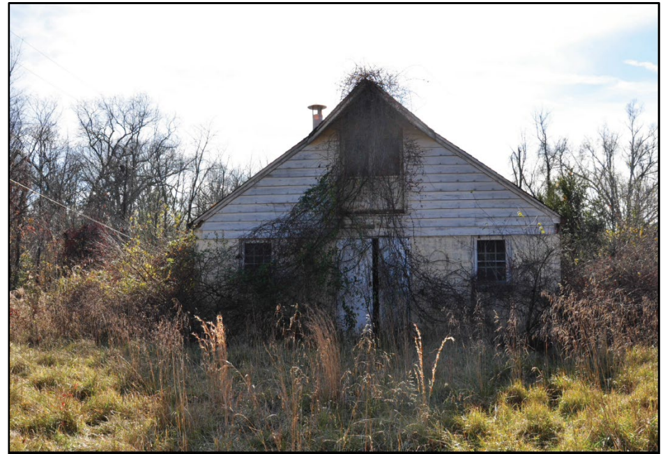
Photo 304: Building 0543, north elevation; photograph courtesy of Mark Edwards and Brian Clevon, 2016
