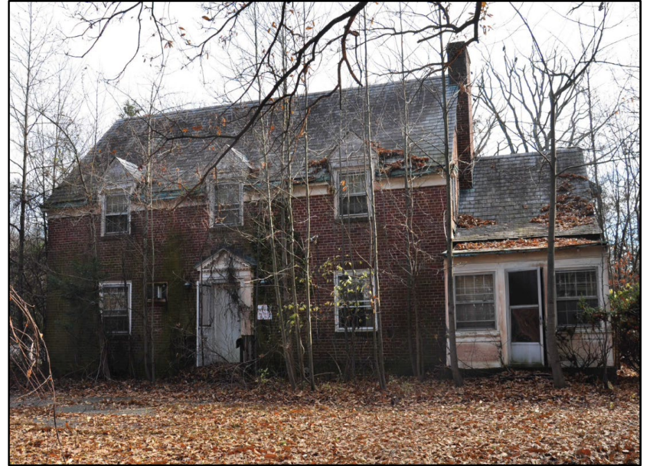
Photo 340: Building 1070, north elevation; photograph courtesy of Brian Clevon, 2017
