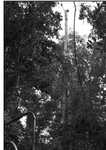
Photo 226: Building 0452, view of radio tower; photograph courtesy of Brian Clevon, 2017
