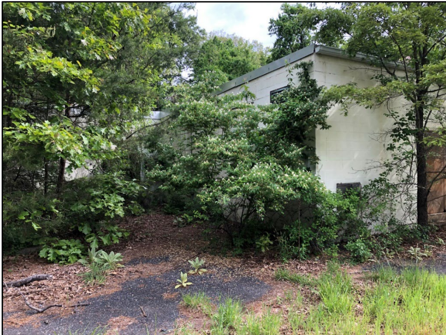
Photo 63: Building 0288, south elevation; photograph courtesy of the USDA
