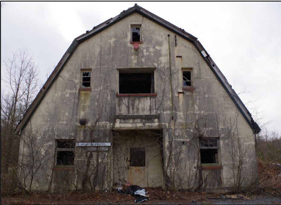
Photo 83: Building 0322, east elevation
