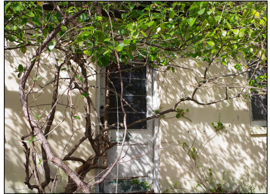
Photo 103: Building 0328, entrance on south elevation
