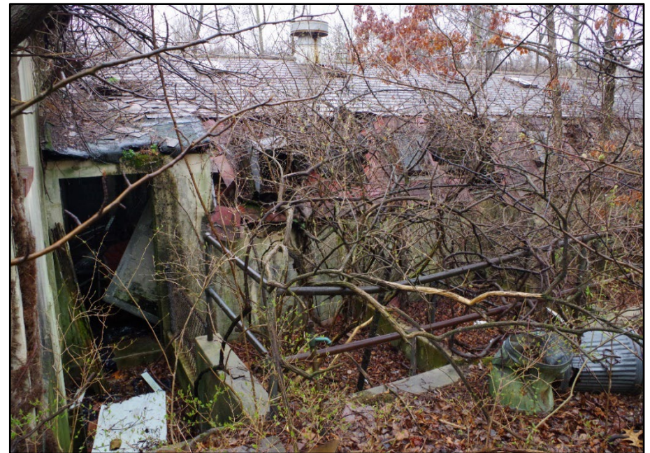
Photo 161: Building 0340, rear wing
