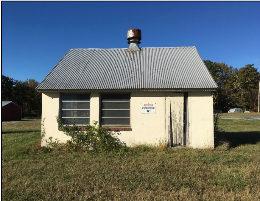
Photo 391: Building 1289, south elevation
