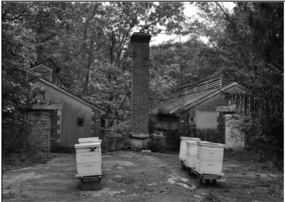
Photo 260: Building 0473, west elevation; photograph courtesy of Mark Edwards and Brian Clevon, 2016
