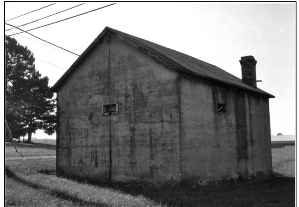
Photo 292: Building 0524, north and west elevations; photograph courtesy of Brian Clevon, 2017
