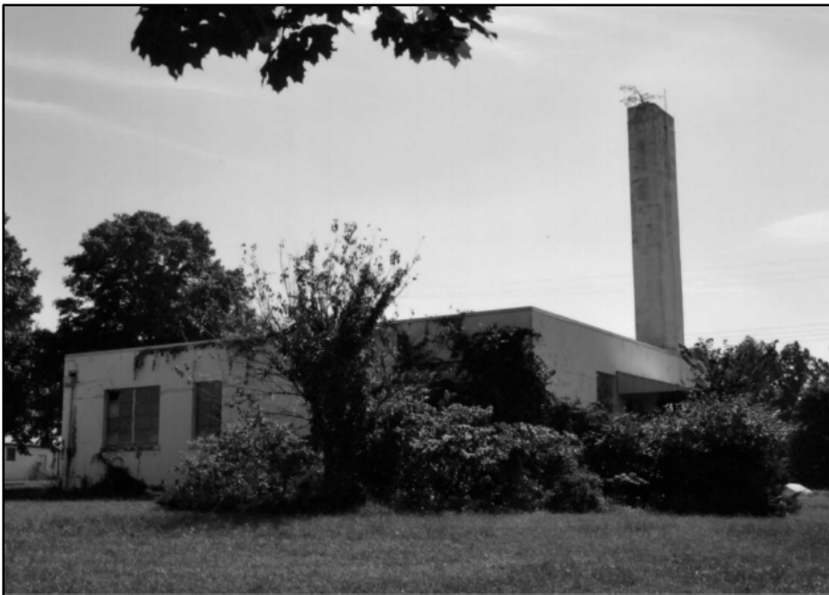
Photo 373: Building 1120, north and west elevations; photograph courtesy of Brian Clevin, 2017
