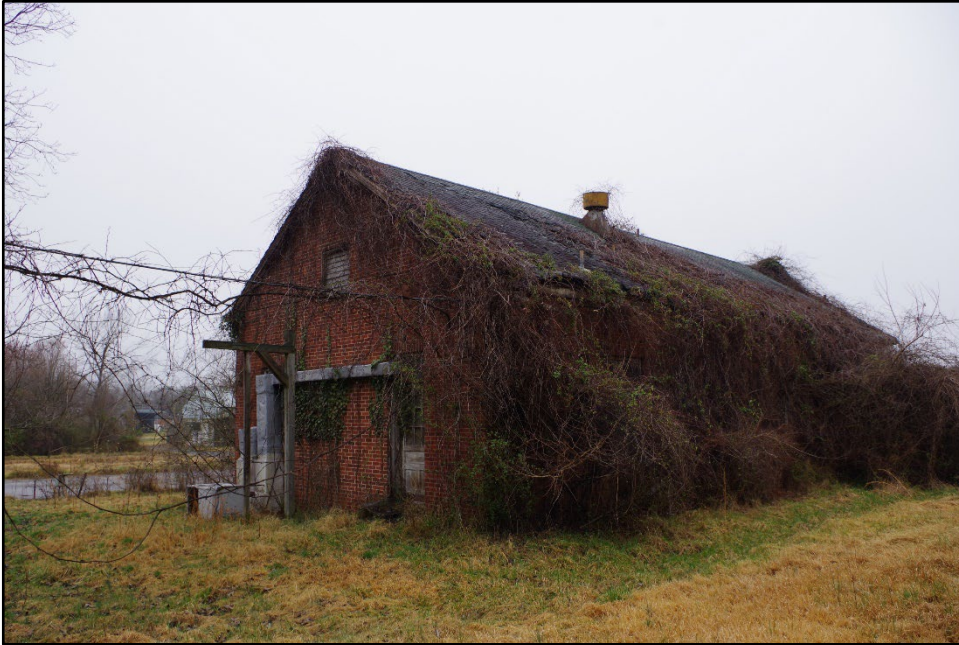
Photo 24: Building 0044, oblique southwest elevation
