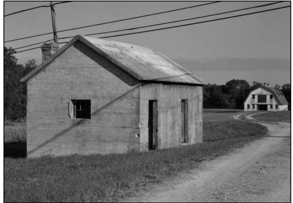
Photo 290: Building 0524, south and east elevations; photograph courtesy of Brian Clevon, 2017
