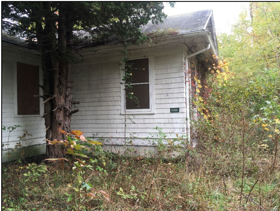
Photo 07: Building 0018, building number
