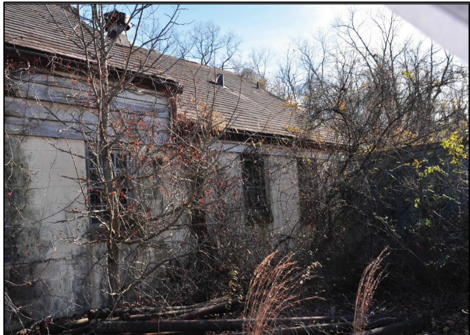
Photo 303: Building 0543, west elevation; photograph courtesy of Mark Edwards and Brian Clevon, 2016
