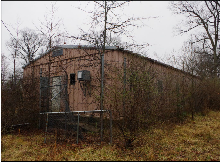
Photo 135: Building 0337A, north elevation
