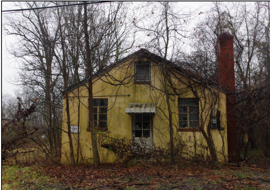
Photo 133: Building 0337, north elevation
