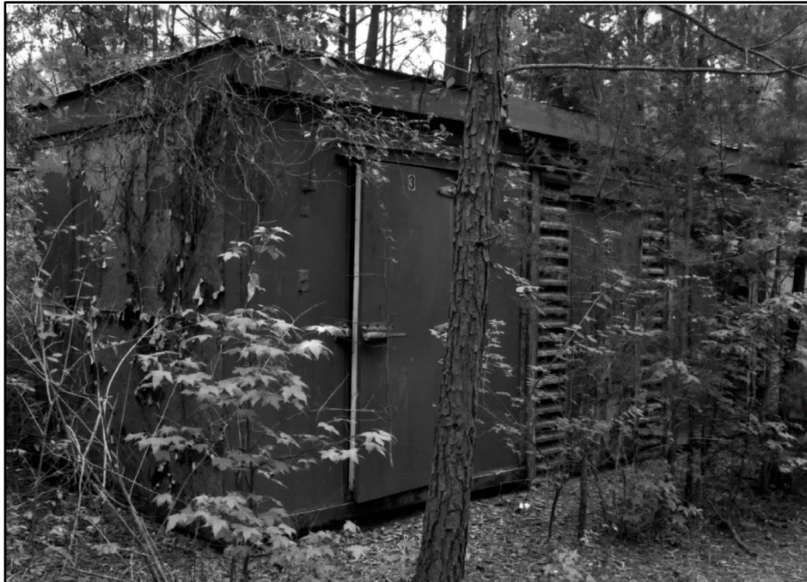
Photo 279: Building 0487-2, north and west elevations; photograph courtesy of Brian Clevon, 2017
