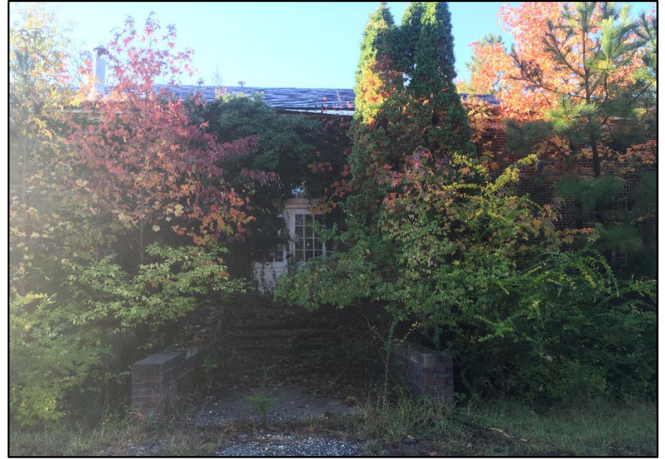
Photo 228: Building 0467, north elevation
