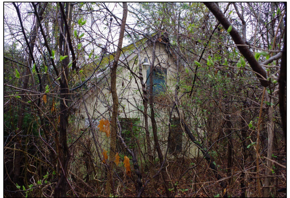
Photo 180: Building 0357, west elevation
