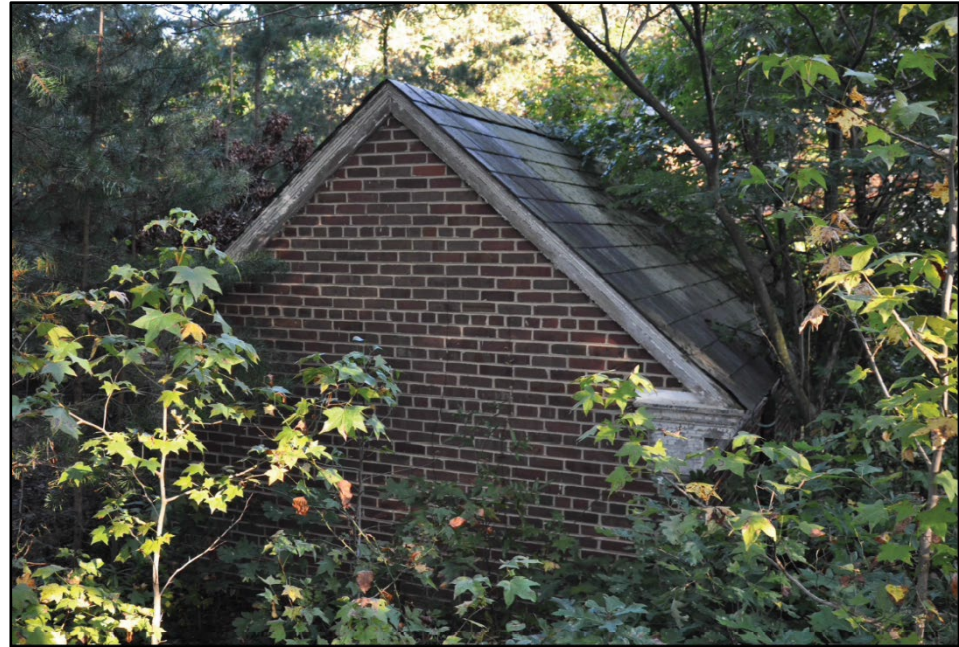
Photo 358: Building 1073, south elevation; photograph courtesy of Brian Clevon, 2017
