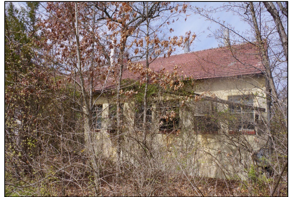
Photo 143: Building 0338, south elevation
