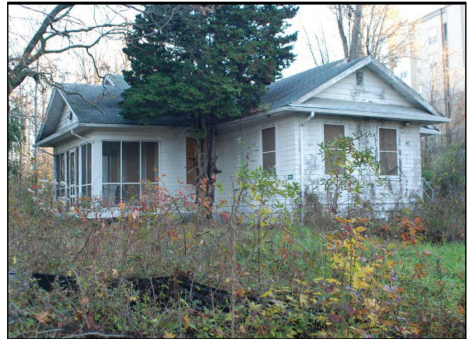
Photo 08: Building 0018, west and south elevations; photograph courtesy of AECOM, 2017
