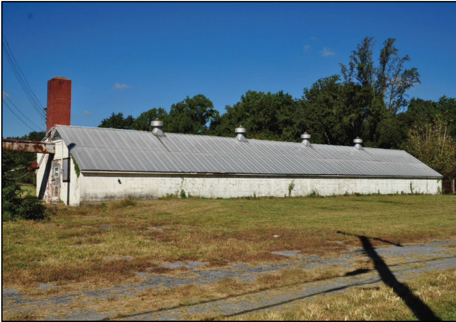
Photo 419: Building 1425, south and east elevations; photograph courtesy of Brian Clevin, 2017
