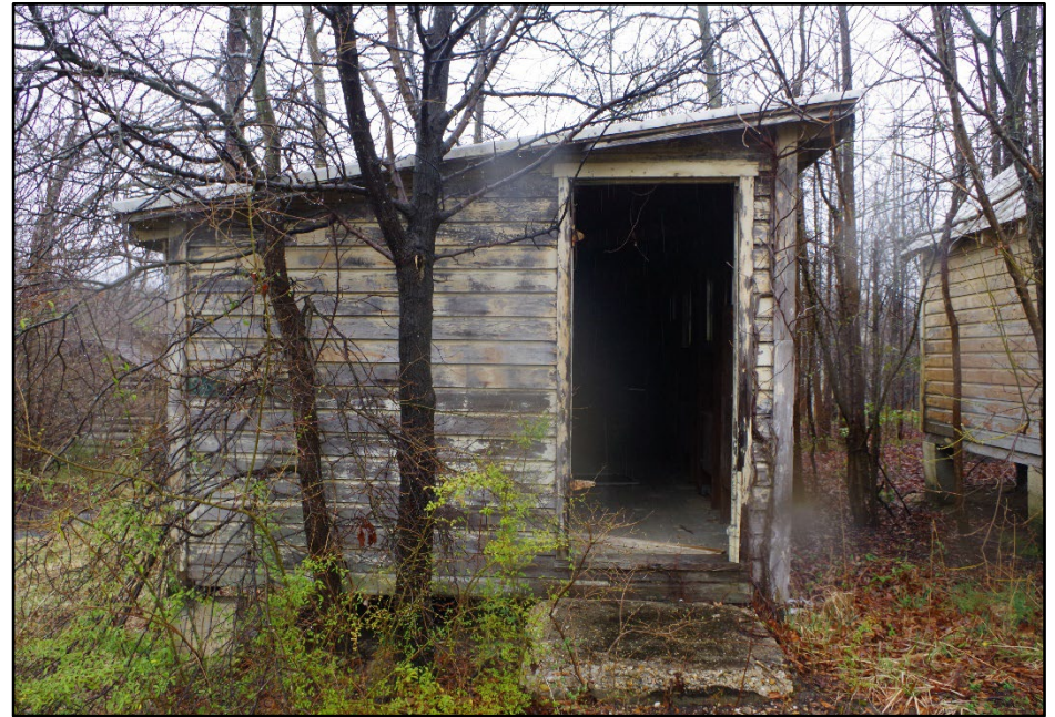
Photo 186: Building 0364, west elevation
