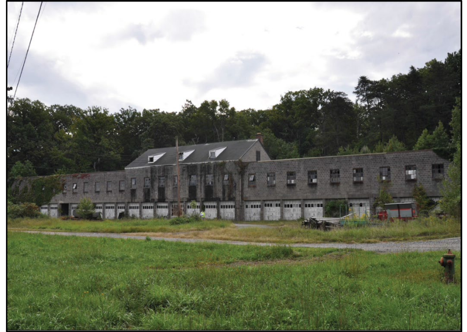
Photo 33: Building 0060, north elevation; photograph courtesy of Mark Edwards and Brian Clevon, 2016
