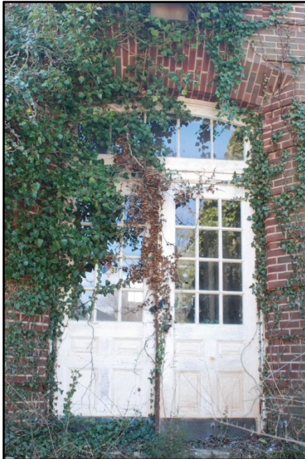
Photo 233: Building 0467, detail of main entrance; photograph courtesy of Brian Clevon, 2017
