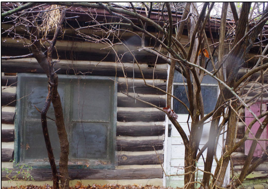
Photo 191: Building 0369, window detail
