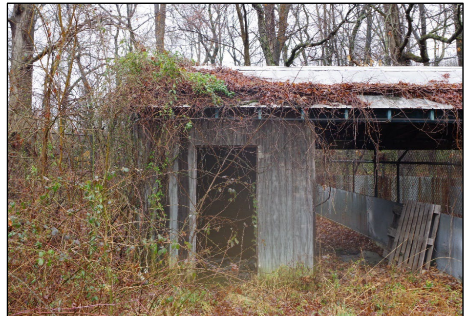
Photo 222: Building 0391, animal stalls, entrance
