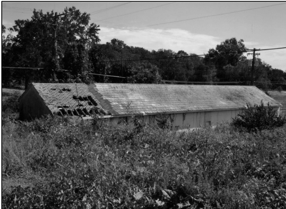
Photo 59: Building 0205, north and west elevations; photograph courtesy of Brian Clevon, 2017
