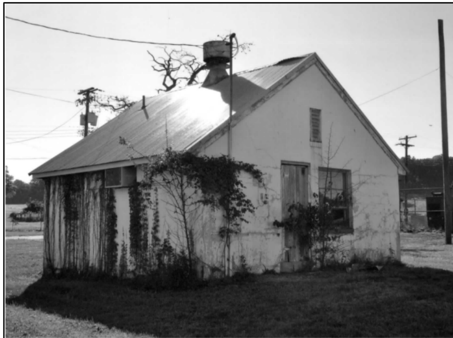
Photo 385: Building 1287, north and west elevations; photograph courtesy of Brian Clevon, 2017
