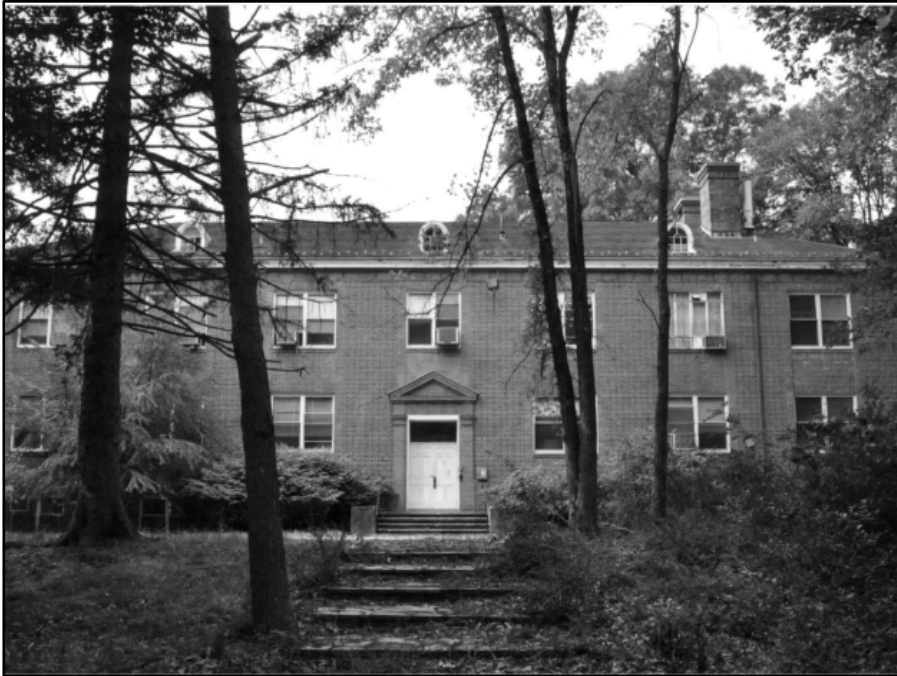
Photo 270: Building 0476, east elevation; photograph courtesy of Brian Clevon, 2017
