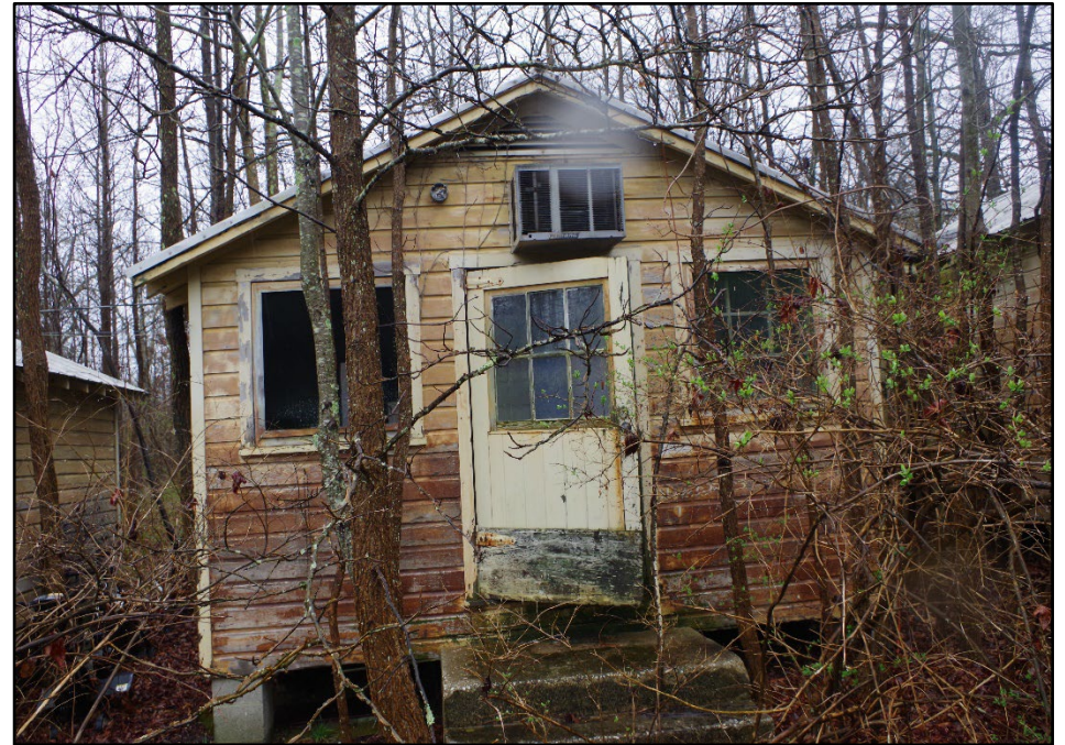
Photo 201: Building 0372, north elevation
