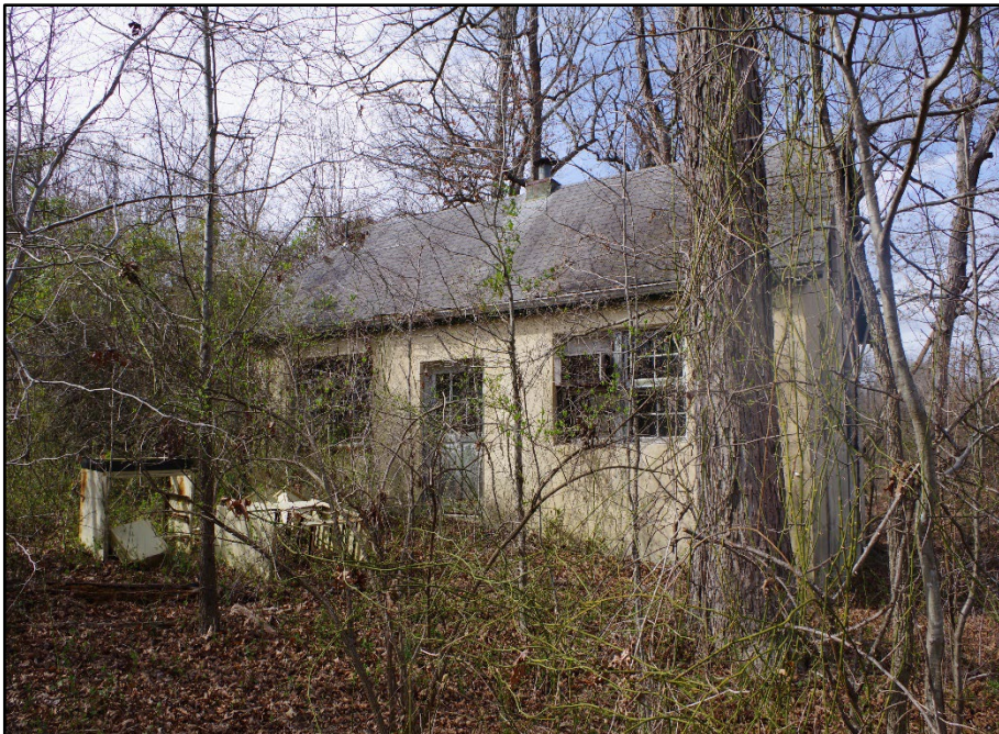
Photo 108: Building 0333, south elevation
