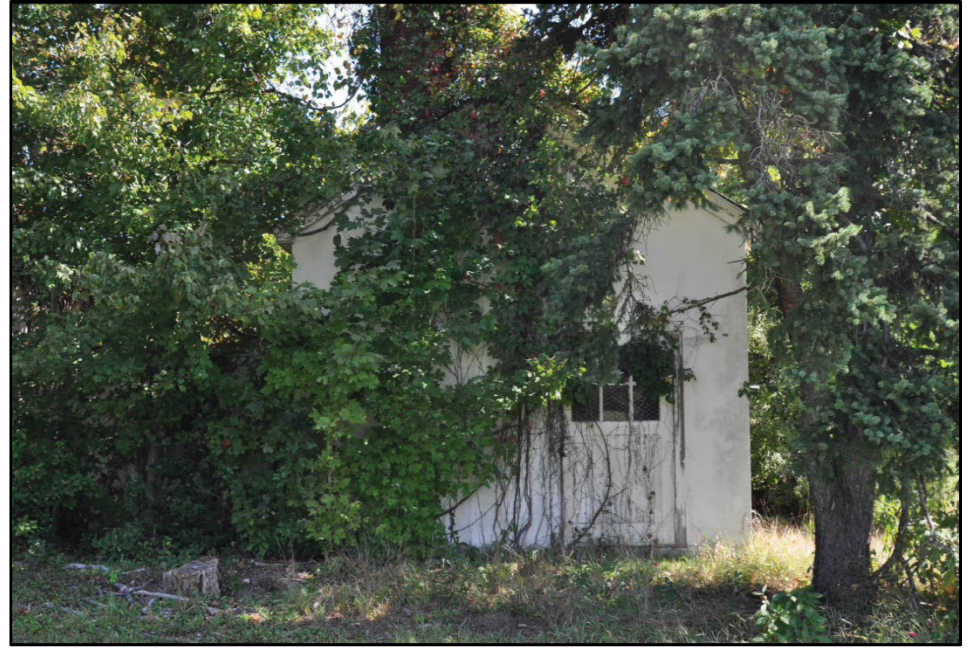
Photo 318: Building 1052, west elevation; photograph courtesy of Mark Edwards and Brian Clevon, 2016
