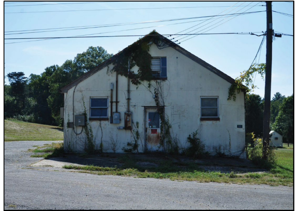
Photo 364: Building 1100, north elevation; photograph courtesy of Brian Clevon, 2017
