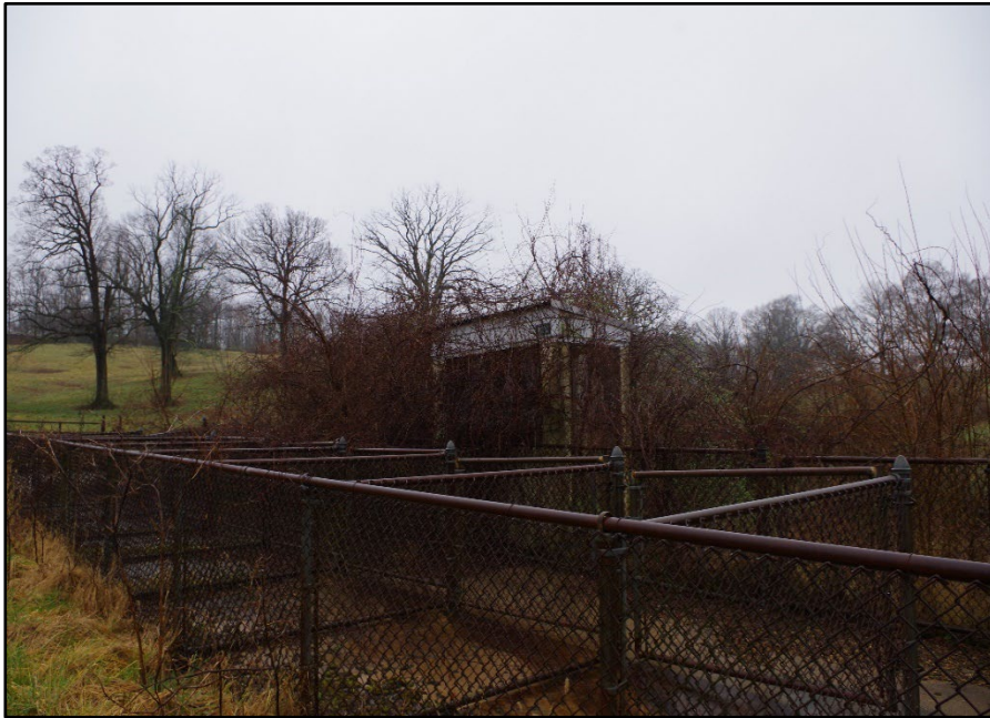
Photo 359: Building 1092, view of building and pen
