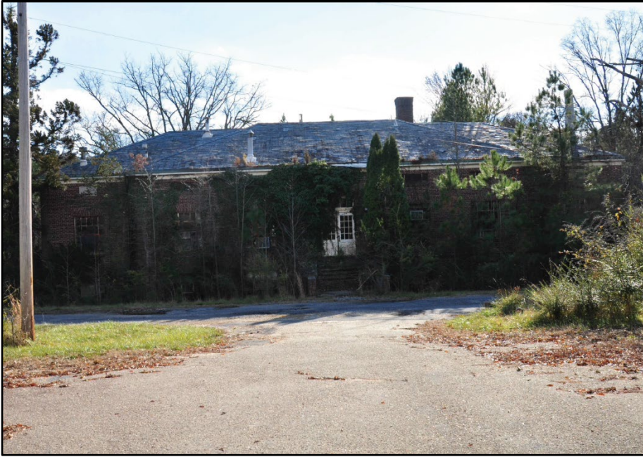
Photo 227: Building 0467, north elevation; photograph courtesy of Brian Clevon, 2017
