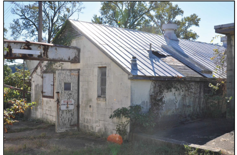
Photo 418: Building 1422, north elevation; photograph courtesy of Brian Clevin, 2017
