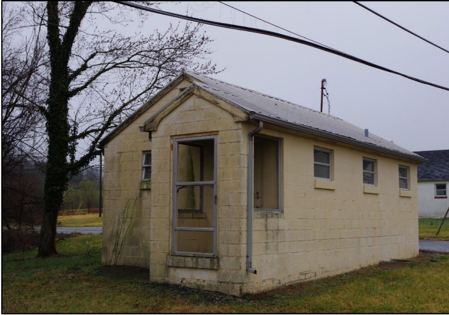
Photo 411: Building 1390, north elevation
