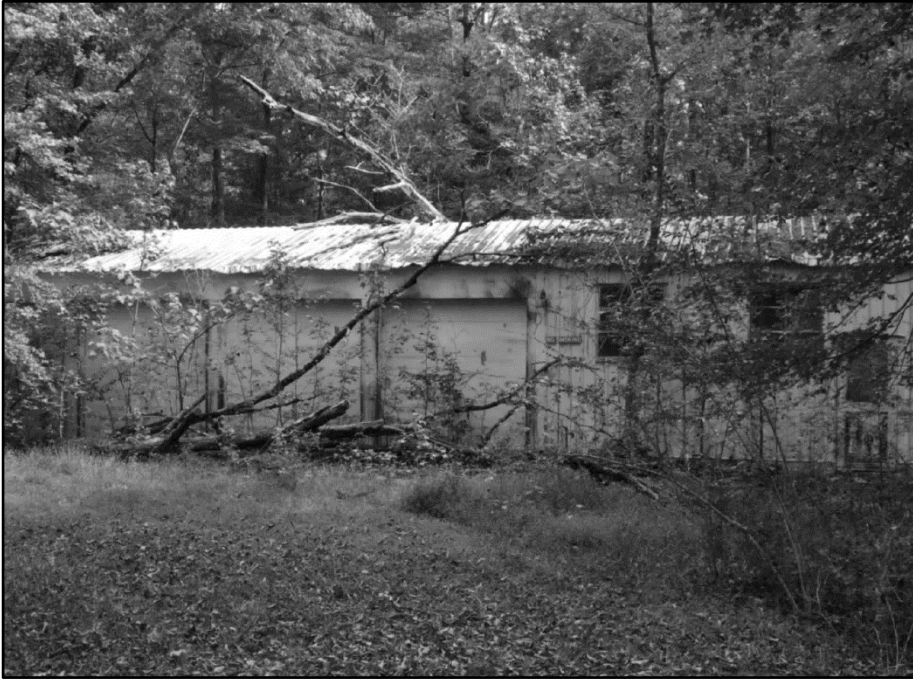
Photo 254: Building 0472, west elevation; photograph courtesy of Brian Clevon, 2017.
