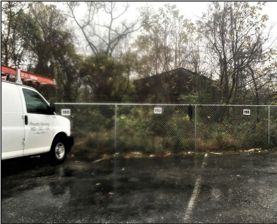
Photo 44: Building 0085B, east (front) and south sides
