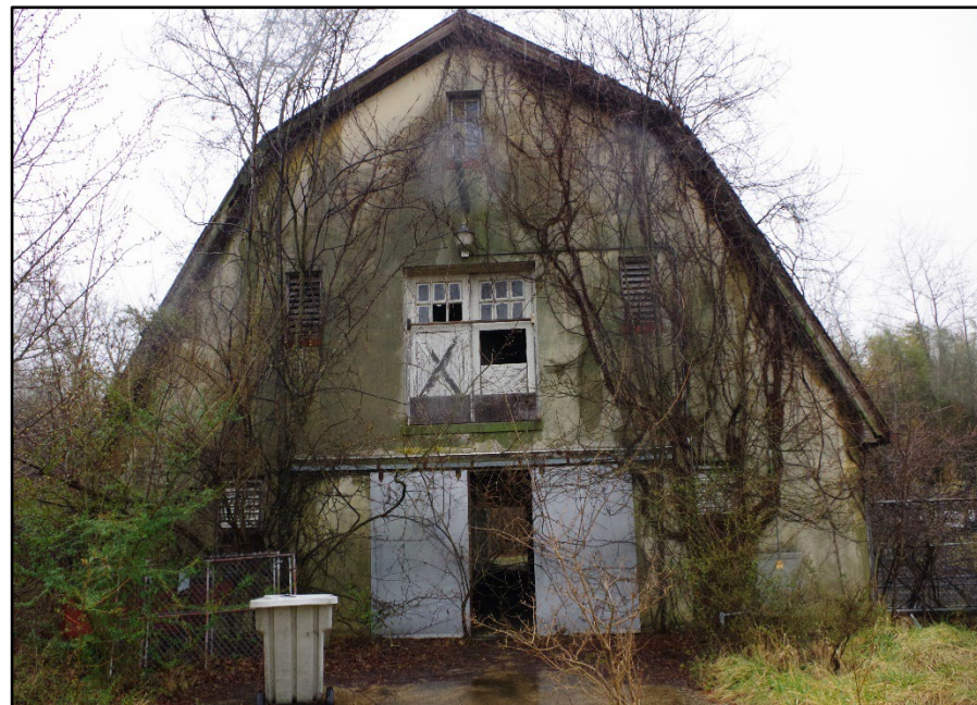
Photo 175: Building 0344, east elevation
