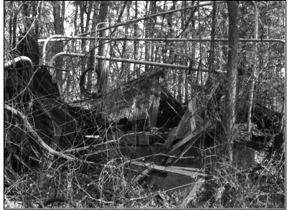
Photo 224: Building 0452, west elevation; photograph courtesy of Brian Clevon, 2017
