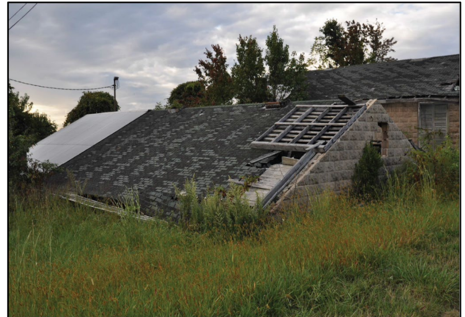
Photo 12: Building 0038, west elevation; photograph courtesy of Mark Edwards and Brian Clevon, 2016
