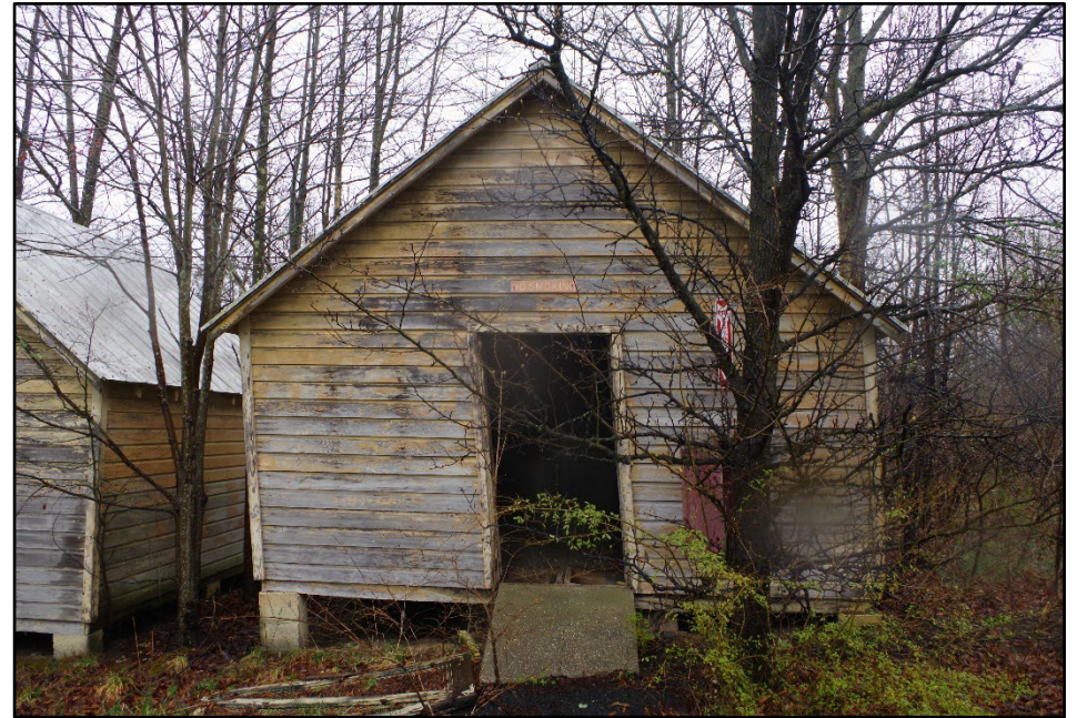
Photo 182: Building 0362, west elevation
