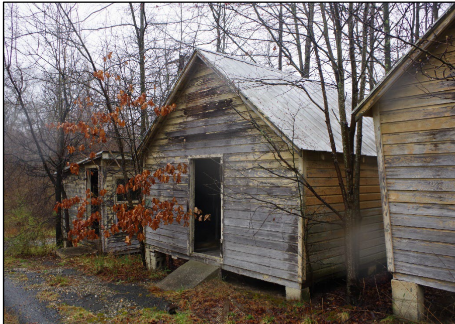
Photo 183: Building 0363, obstructed overview
