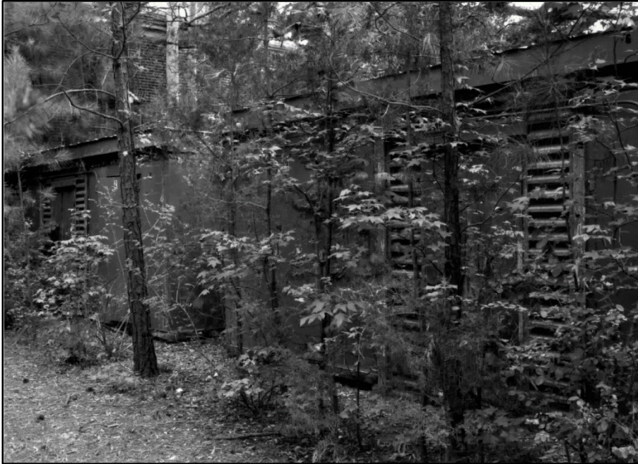
Photo 277: Building 0487-1 and Building 0487-2, west elevation; photograph courtesy of Brian Clevon, 2017
