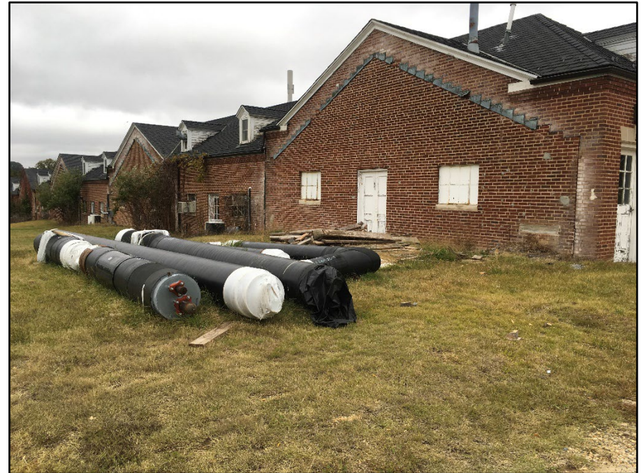
Photo 02: Building 0009, southwest elevation
