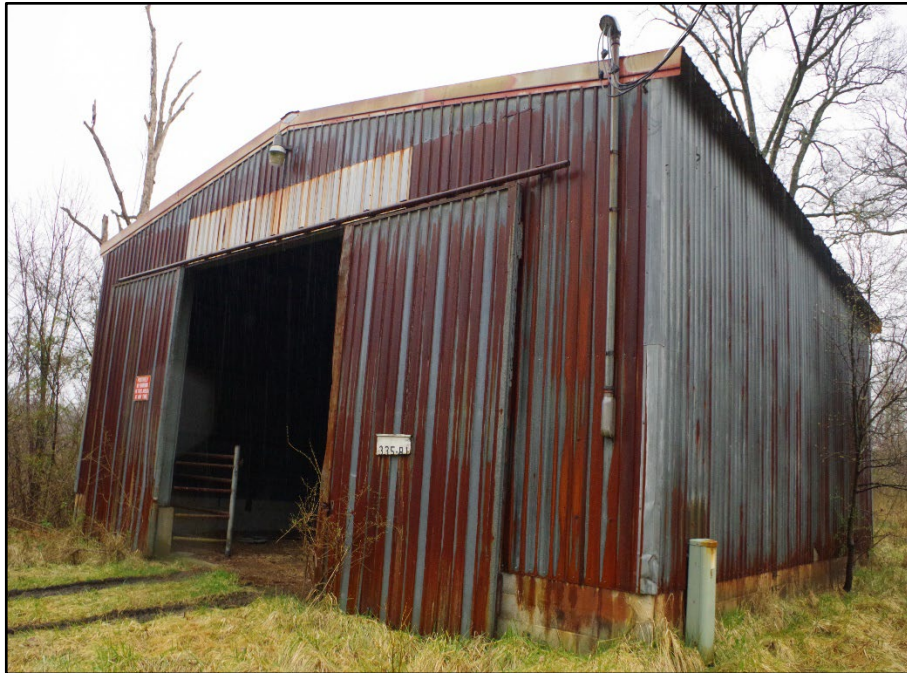
Photo 124: Building 0335B, north elevation
