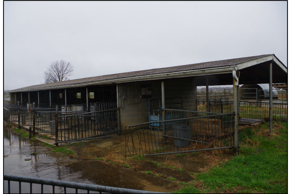
Photo 50: Building 0203B, southern elevation
