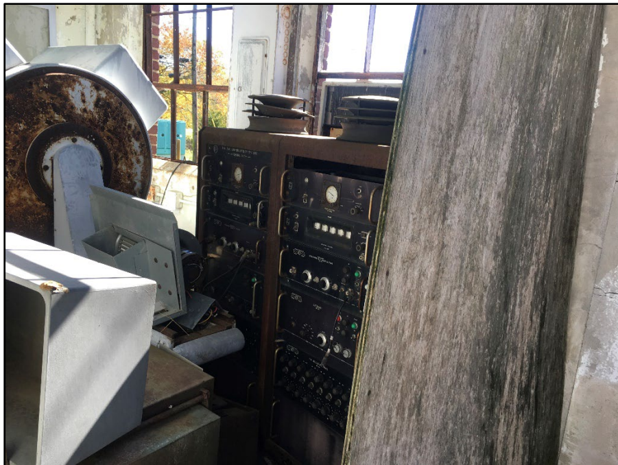
Photo 55: Building 0204A, interior
