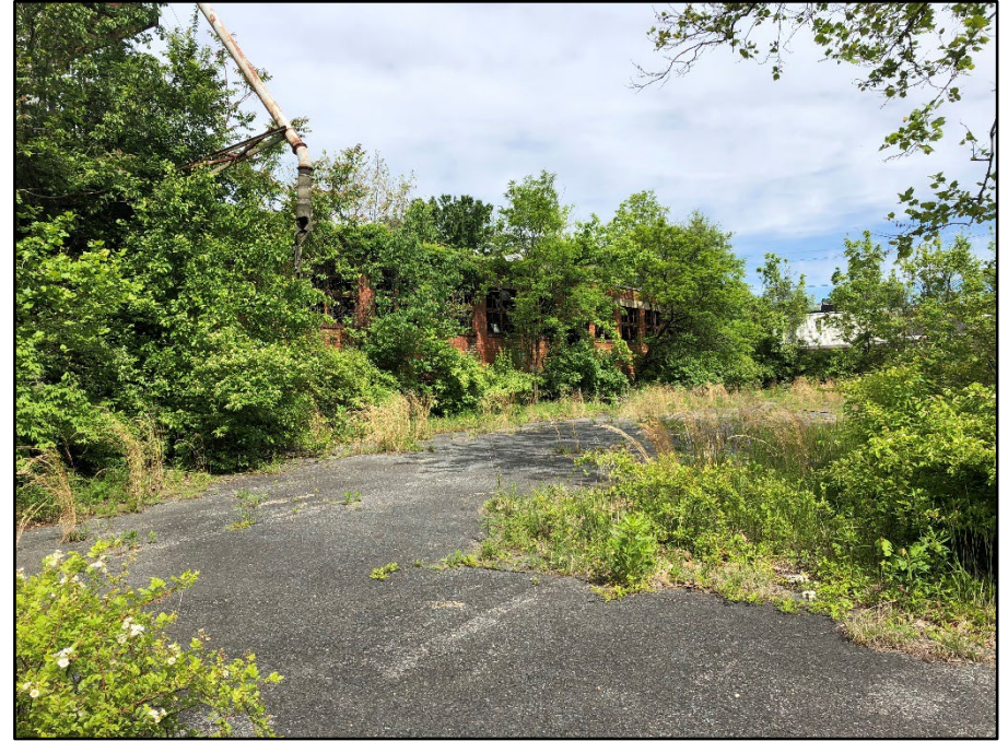
Photo 37: Building 0085, east elevation, camera facing northwest
