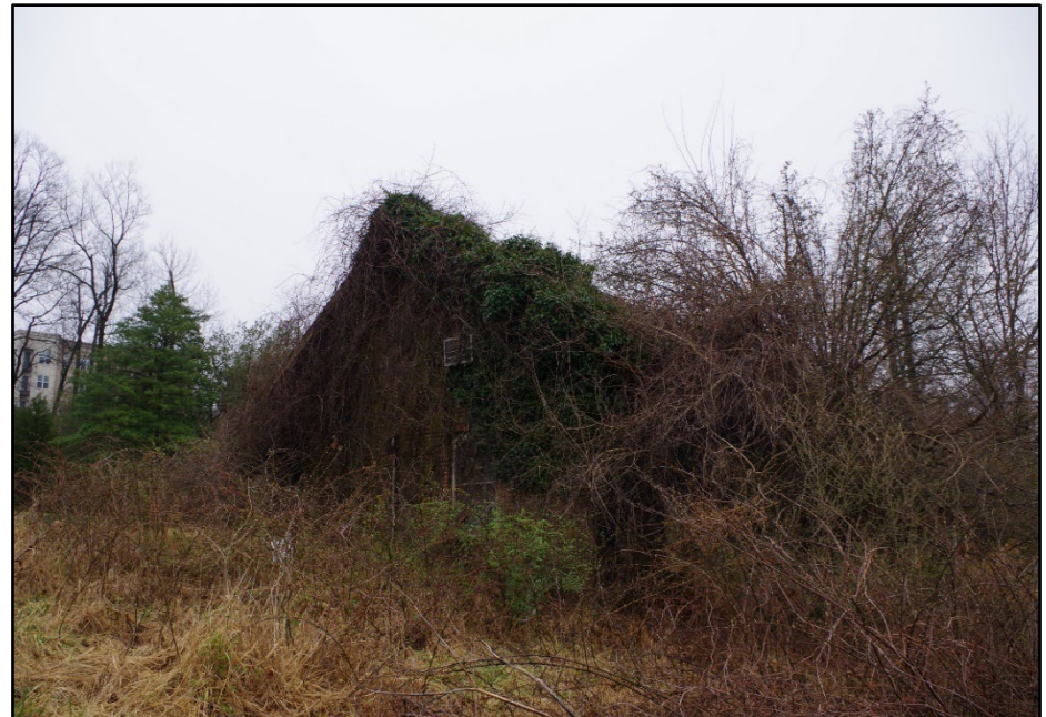
Photo 27: Building 0044, obstructed oblique northeast elevation
