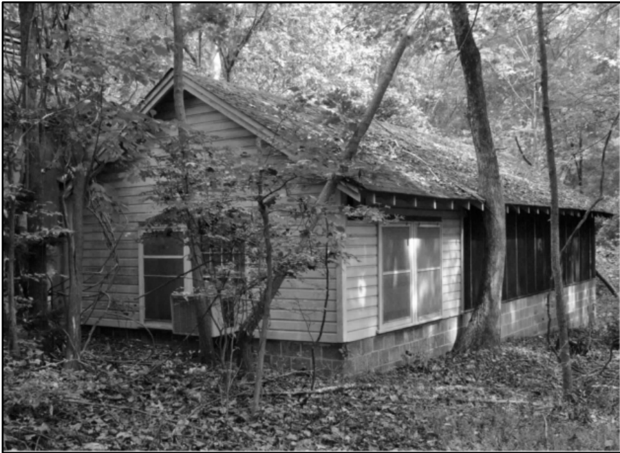
Photo 266: Building 0475, west and south elevations; photograph courtesy of Brian Clevon, 2017
