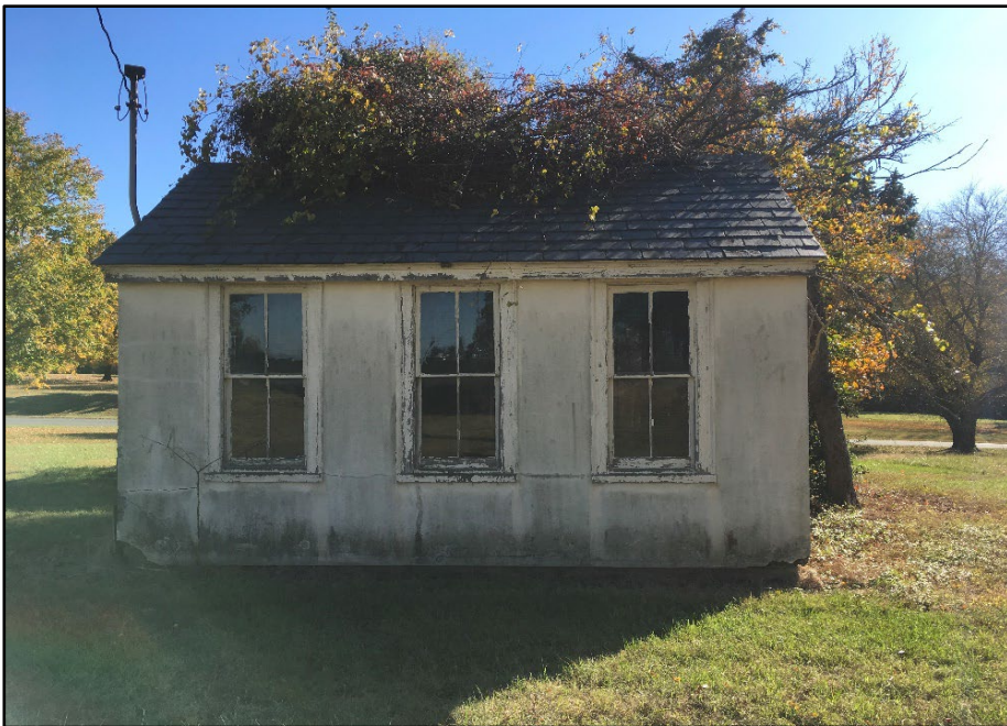
Photo 323: Building 1053, west and north elevations; photograph courtesy of Mark Edwards and Brian Clevon, 2016
