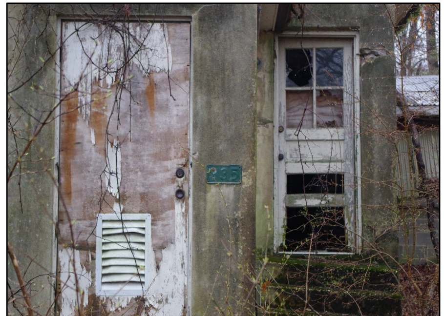
Photo 121: Building 0335, entrance on east elevation
