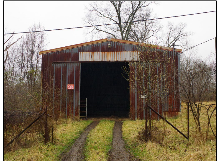
Photo 125: Building 0335B, north elevation
