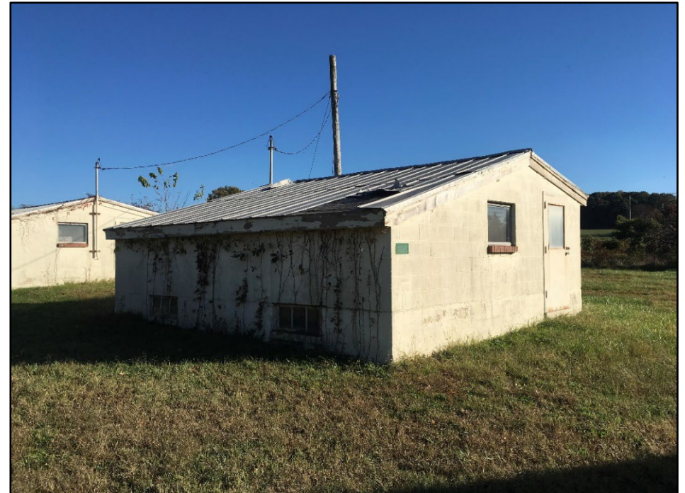
Photo 402: Building 1328, north and west elevations; photograph courtesy of Brian Clevon, 2017
