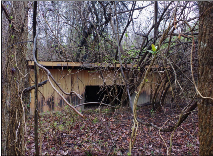
Photo 165: Building 0342A, overview
