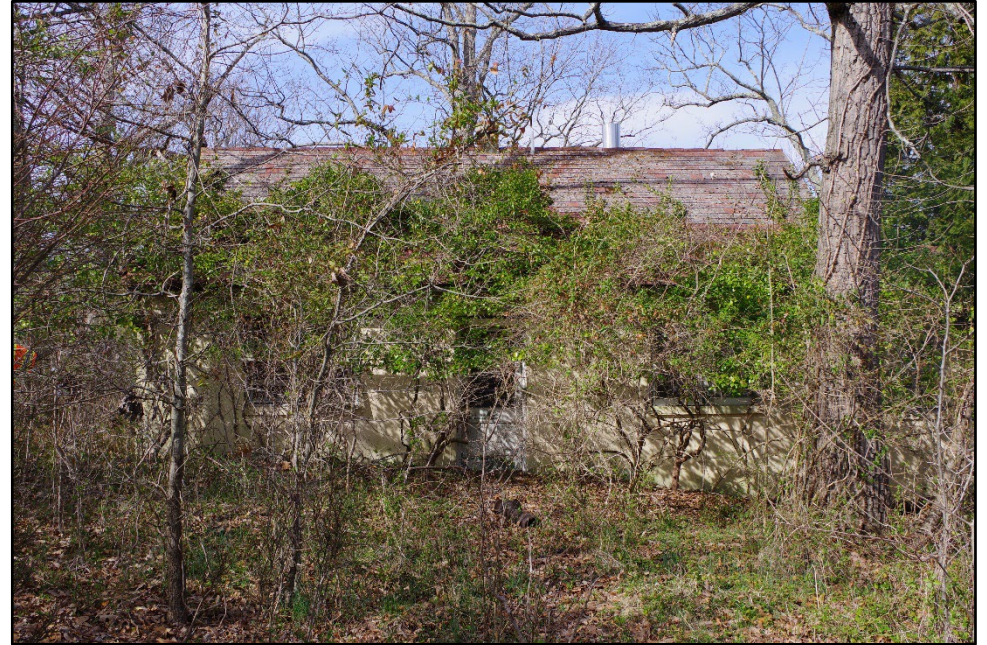
Photo 99: Building 0328, south elevation
