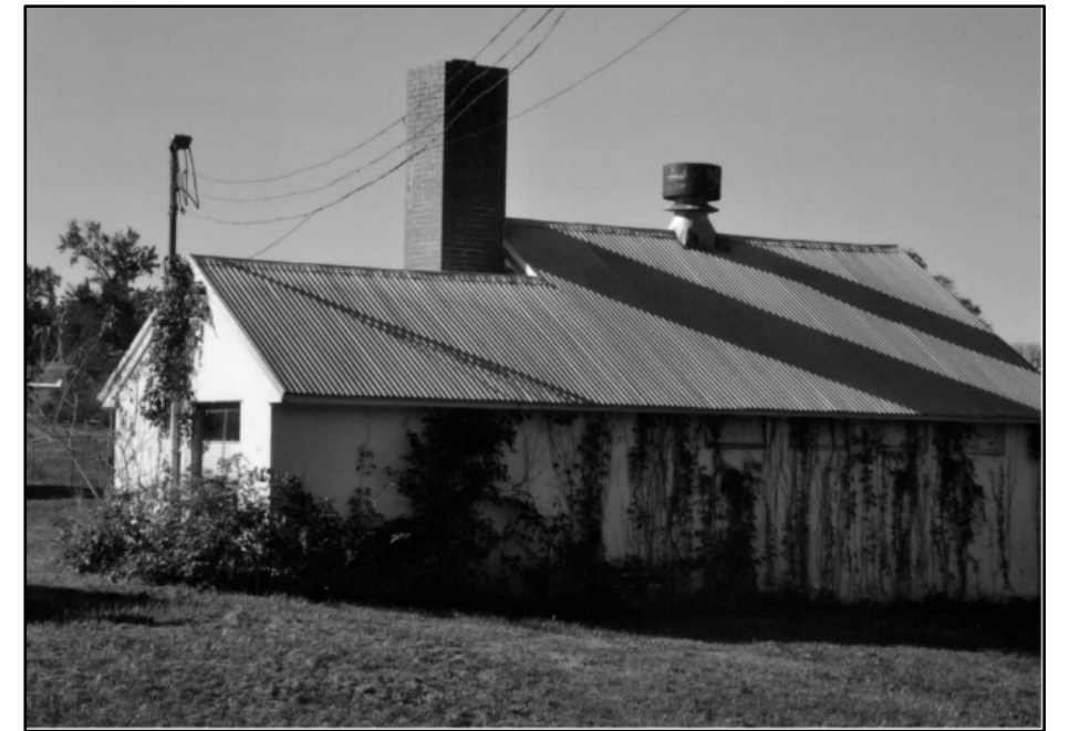
Photo 398: Building 1292, east and north elevations; photograph courtesy of Brian Clevon, 2017
