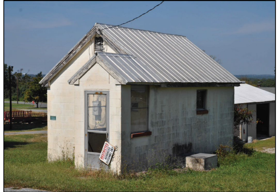
Photo 368: Building 1104, south and east elevations; photograph courtesy of Brian Clevin, 2017
