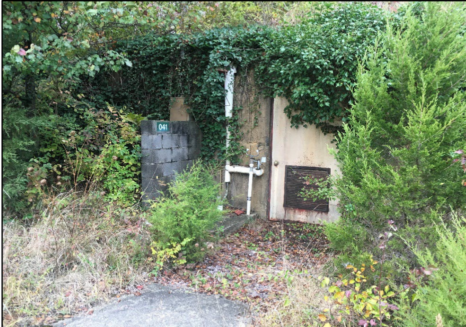
Photo 21: Building 0041, east elevation
