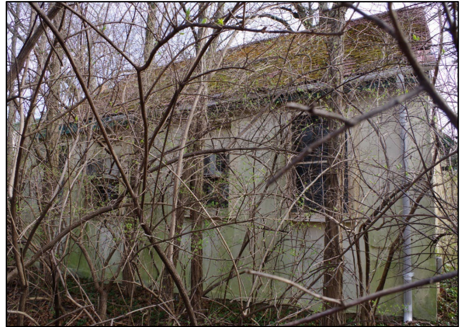
Photo 70: Building 0321, rear wing detail
