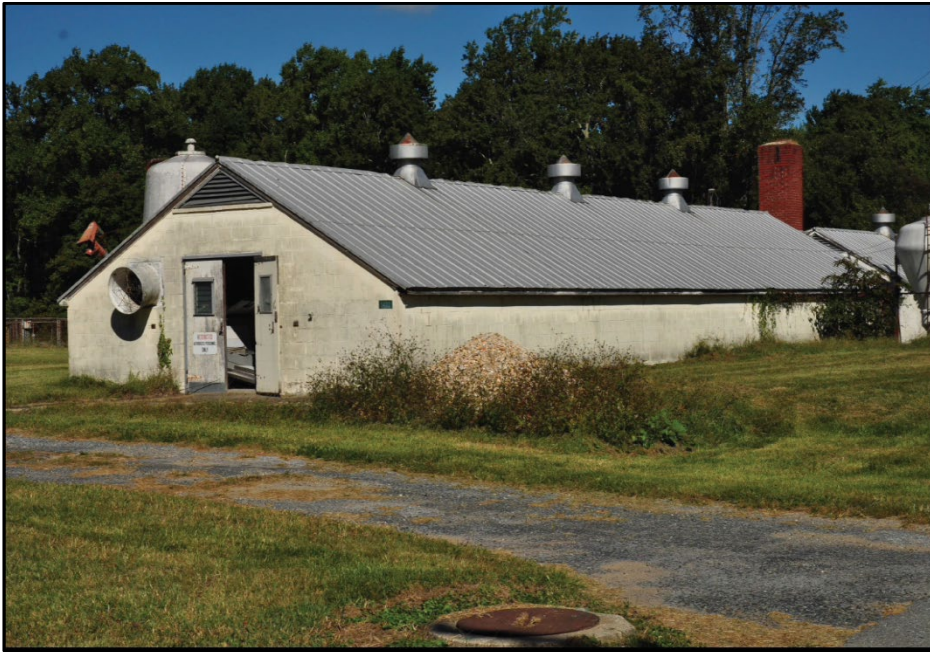
Photo 415: Building 1422, south and east elevations; photograph courtesy of Brian Clevin, 2017
