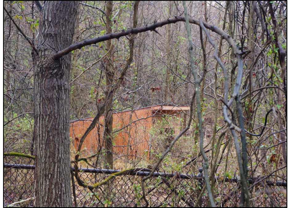
Photo 170: Building 0342C, obstructed overview
