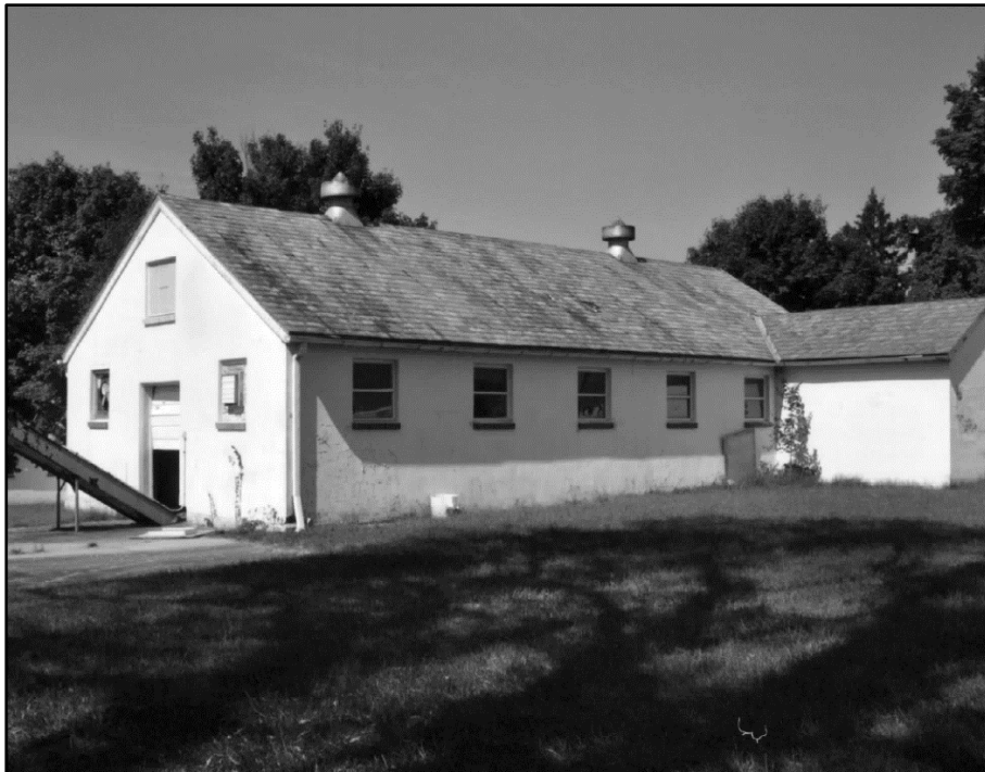
Photo 333: Building 1063, south and east elevations; photograph courtesy of Brian Clevon, 2017
