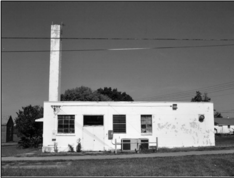
Photo 371: Building 1120, south elevation, camera facing north; photograph courtesy of Brian Clevin, 2017
