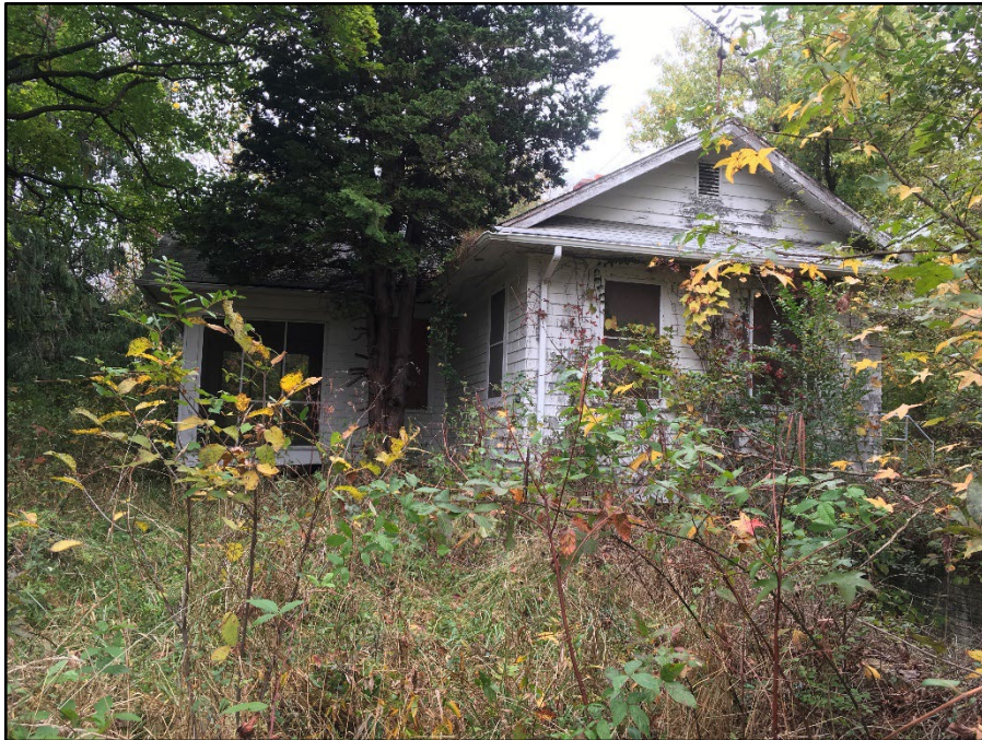
Photo 05: Building 0018, west and south elevations
