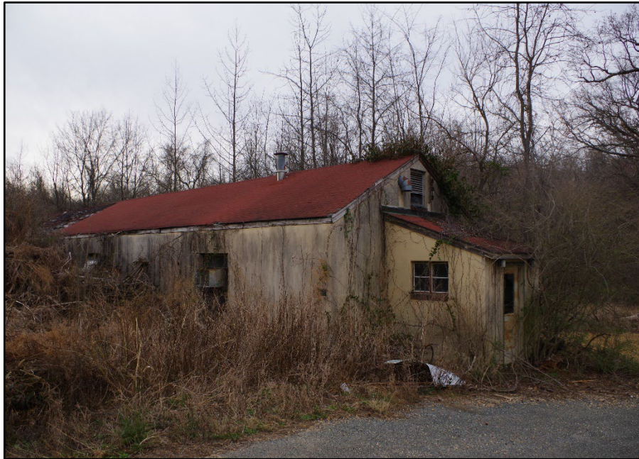
Photo 94: Building 0327, south elevation
