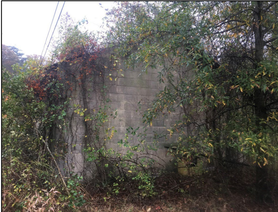
Photo 307: Building 0543A, east elevation
