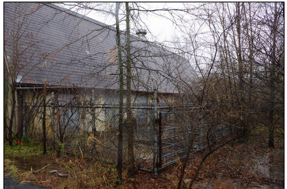
Photo 176: Building 0344, pens attached to south elevation
