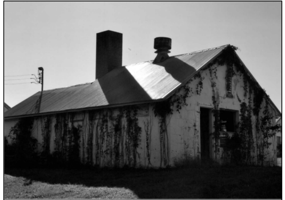
Photo 396: Building 1292, north and west elevations; photograph courtesy of Brian Clevon, 2017
