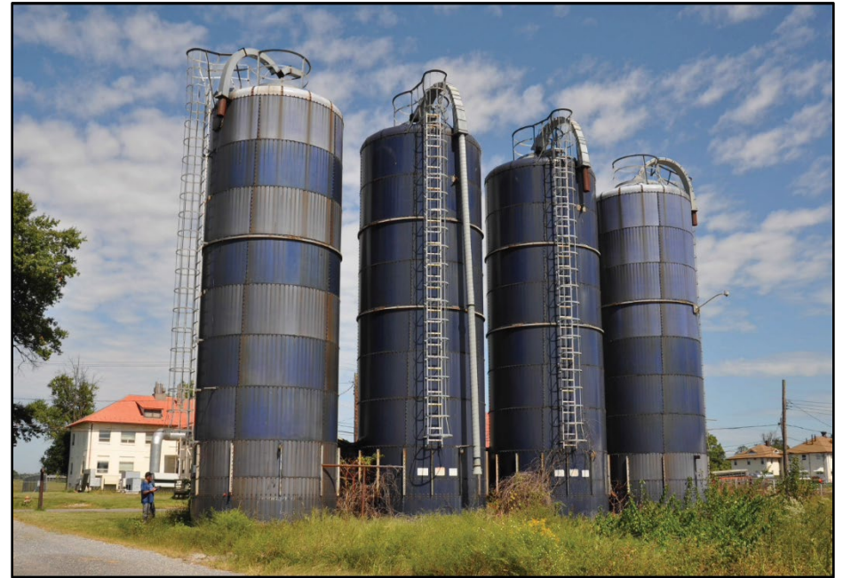
Photo 46: Building 0166A, south elevation; photograph courtesy of Mark Edwards and Brian Clevin, 2016
