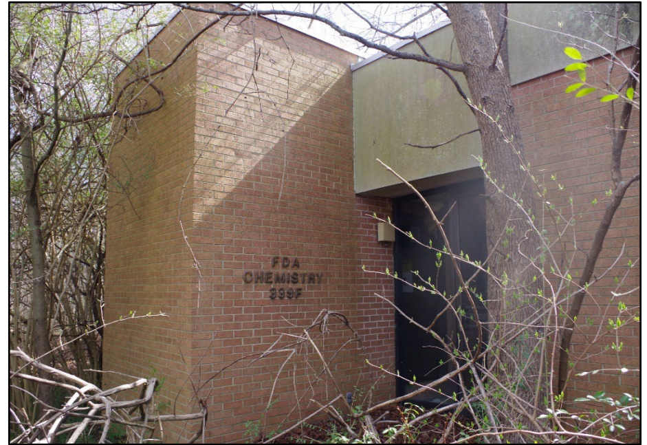
Photo 155: Building 0339F, northwest elevation
