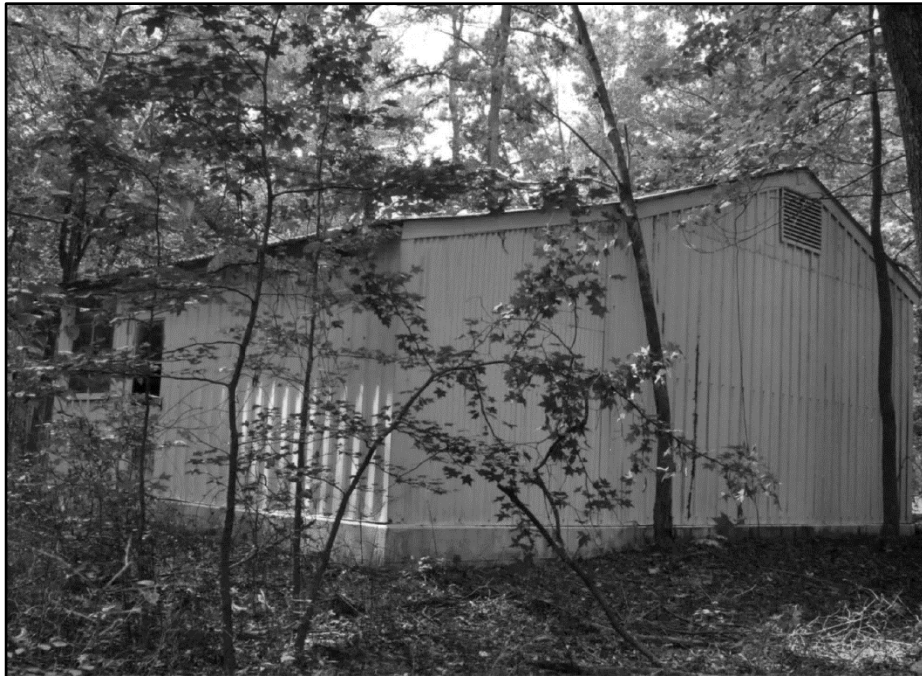
Photo 256: Building 0472, east and north elevations; photograph courtesy of Brian Clevon, 2017.
