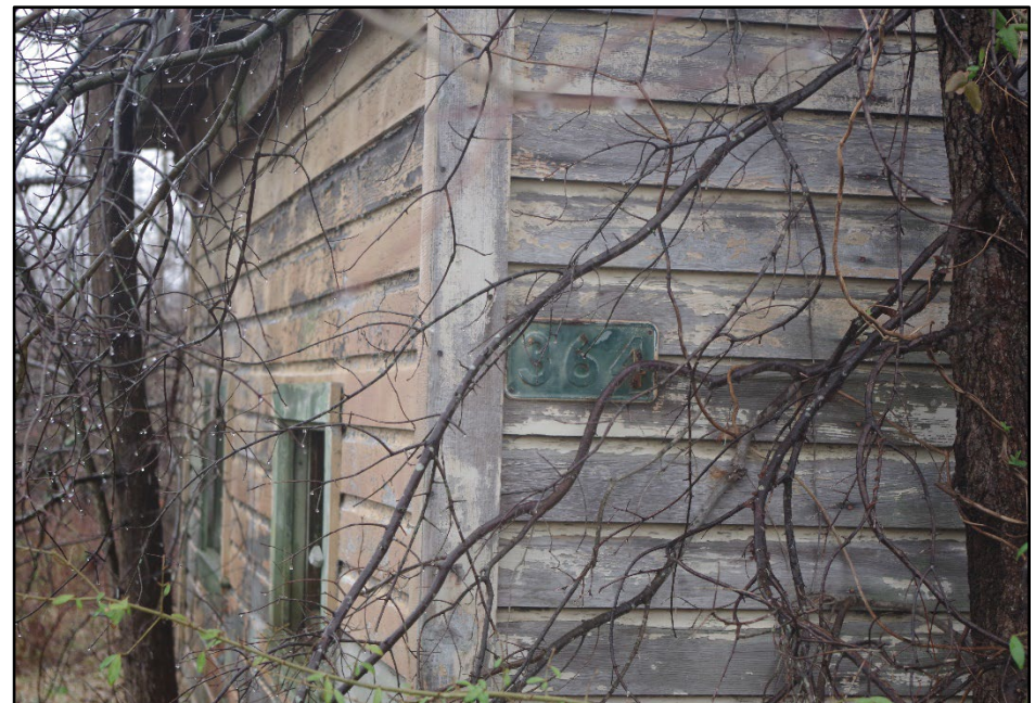
Photo 188: Building 364, view of building number on west elevation
