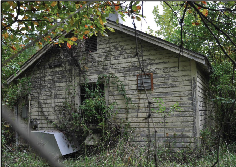
Photo 237: Building 0468, west elevation; photograph courtesy of Brian Clevon, 2017
