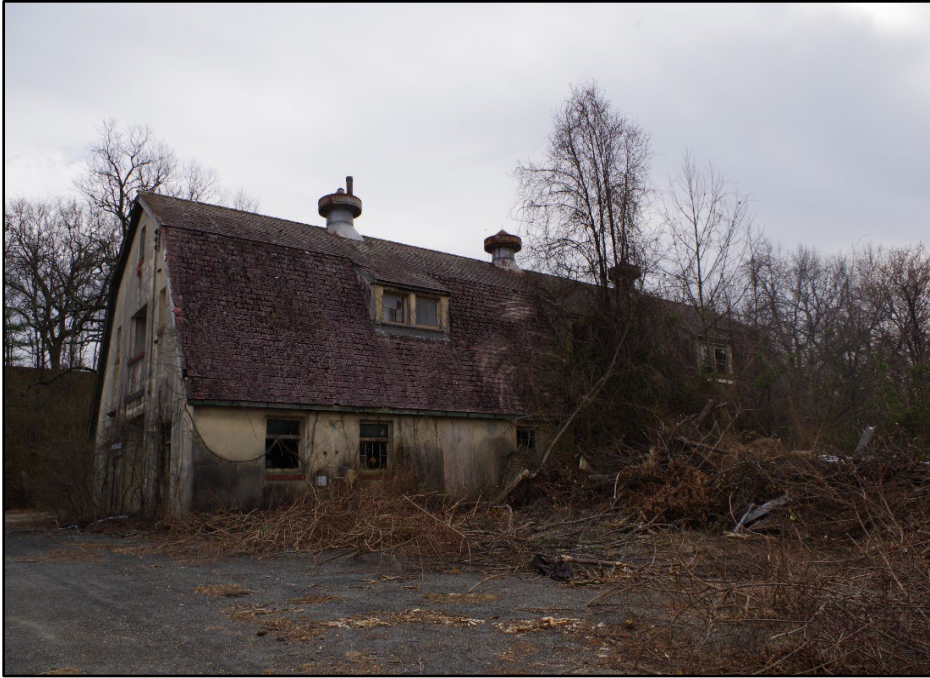
Photo 81: Building 0322, north elevation
