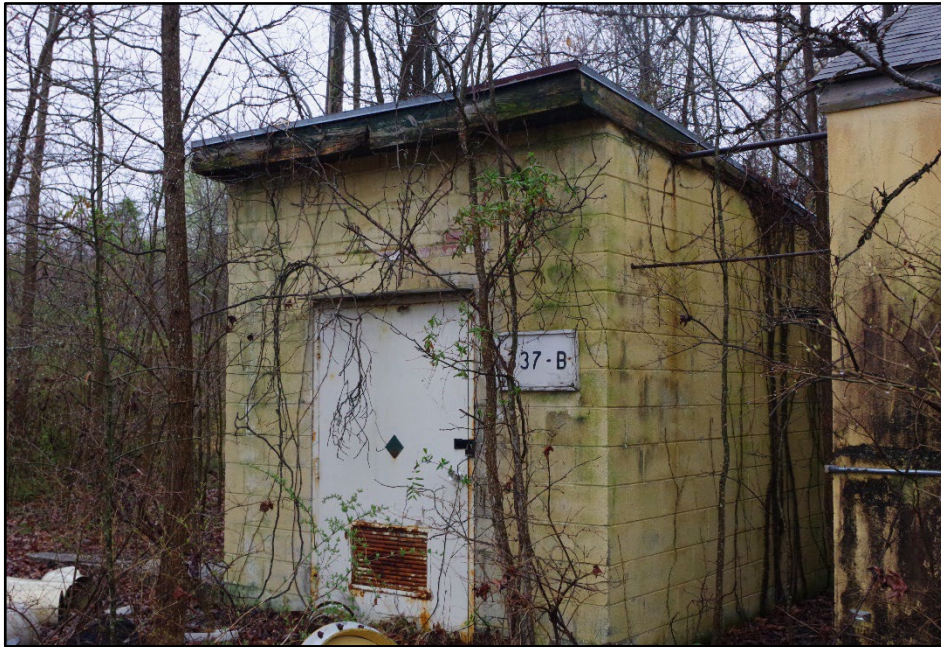
Photo 137: Building 0337B, camera facing southwest
