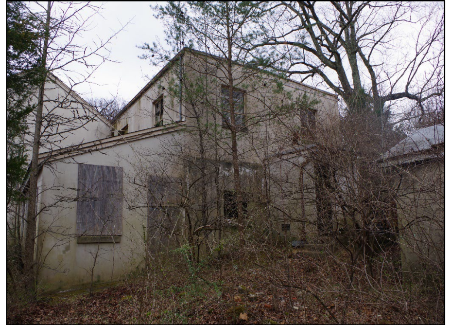
Photo 94: Building 0324B, west elevation
