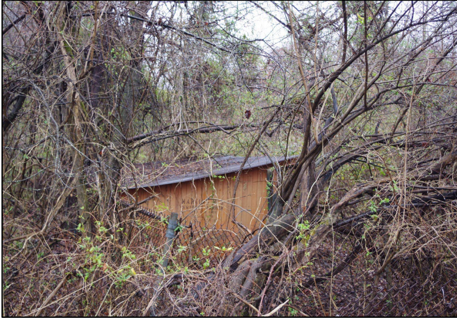
Photo 171: Building 0342D, obstructed west elevation
