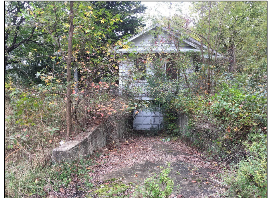
Photo 06: Building 0018, south elevation
