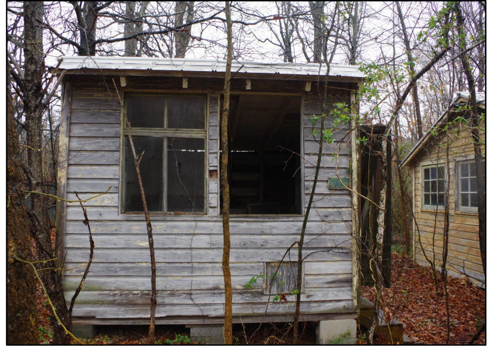
Photo 214: Building 0378, east elevation
