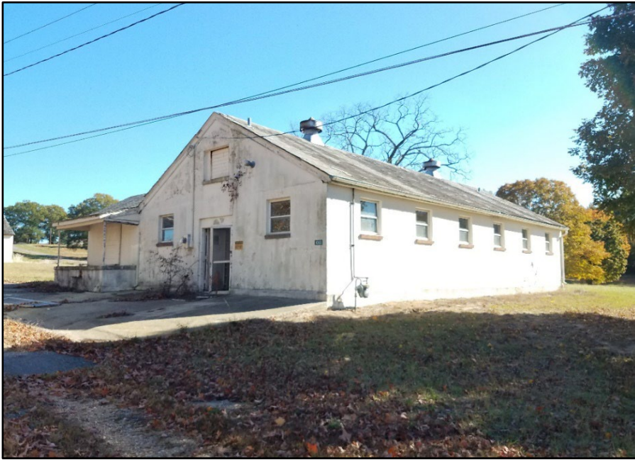
Photo 331: Building 1063, north and west elevations
