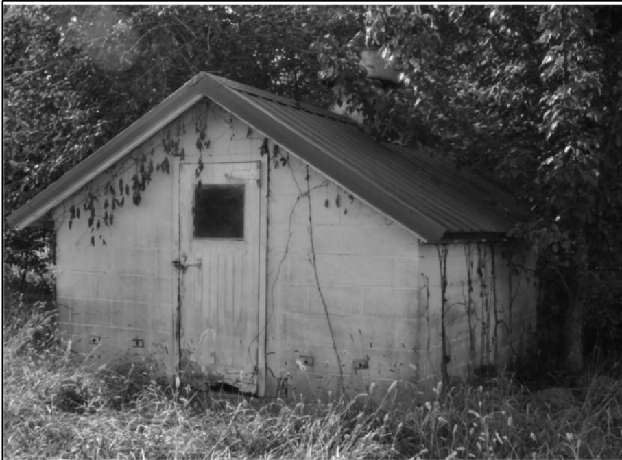
Photo 295: Building 04541C, north and west elevations; photograph courtesy of Mark Edwards and Brian Clevon, 2016
