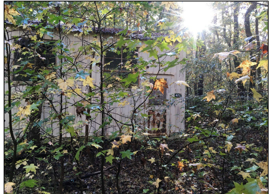
Photo 257: Building 0472, west elevation
