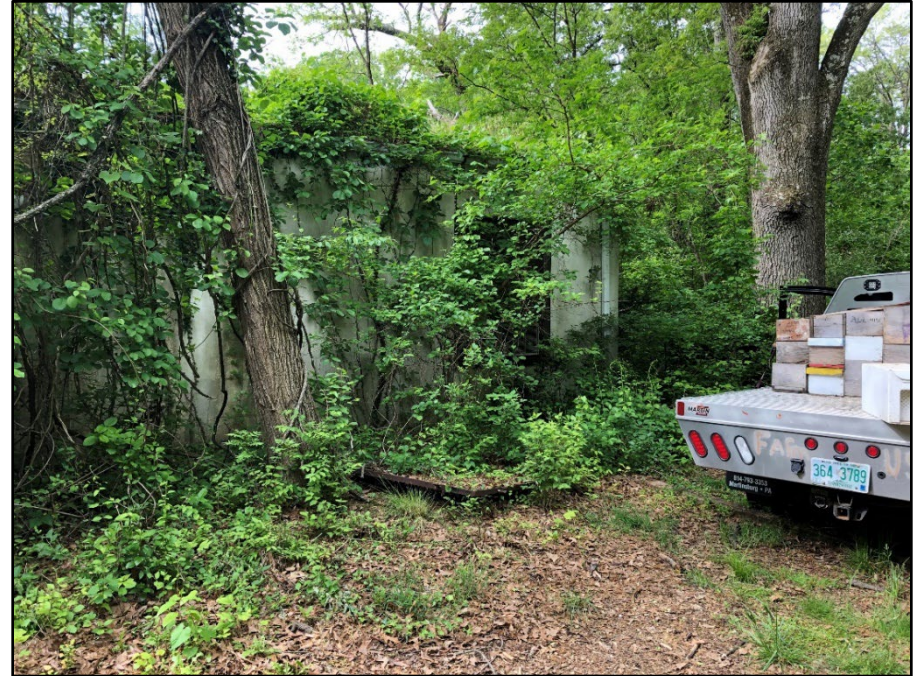
Photo 62: Building 0288, eastern elevation; photograph courtesy of the USDA
