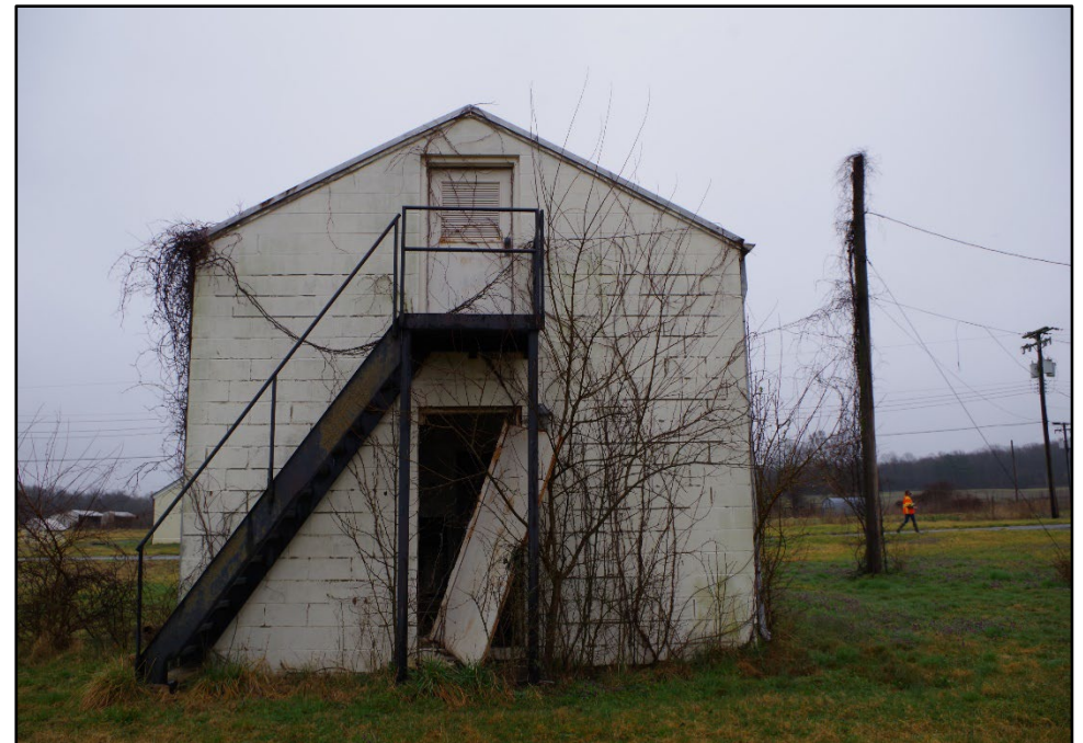
Photo 390: Building 1288, west elevation
