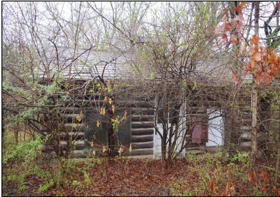
Photo 189: Building 0369, south elevation
