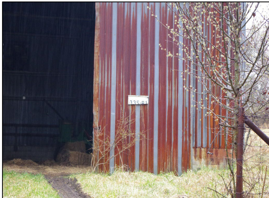
Photo 126: Building 0335B, building number detail
