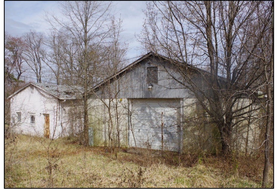
Photo 145: Building 0338A and 0338B, west elevations
