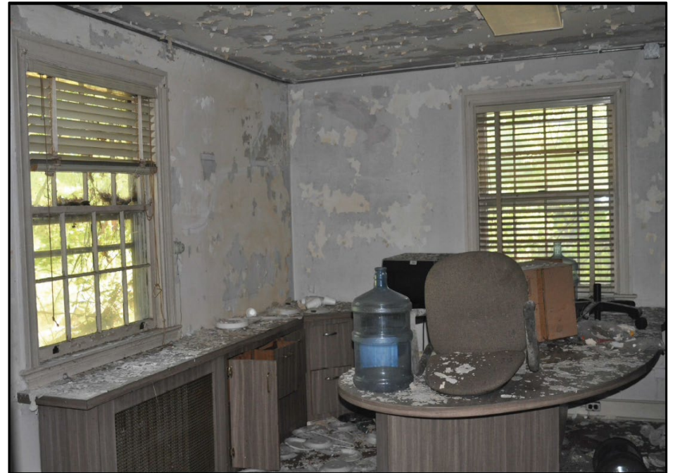
Photo 346: Building 1070, interior view; photograph courtesy of Brian Clevon, 2017
