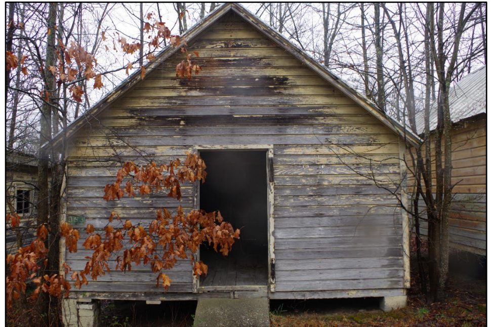
Photo 184: Building 0363, west elevation
