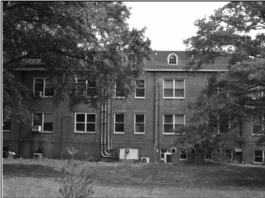
Photo 272: Building 0476, west elevation; photograph courtesy of Brian Clevon, 2017
