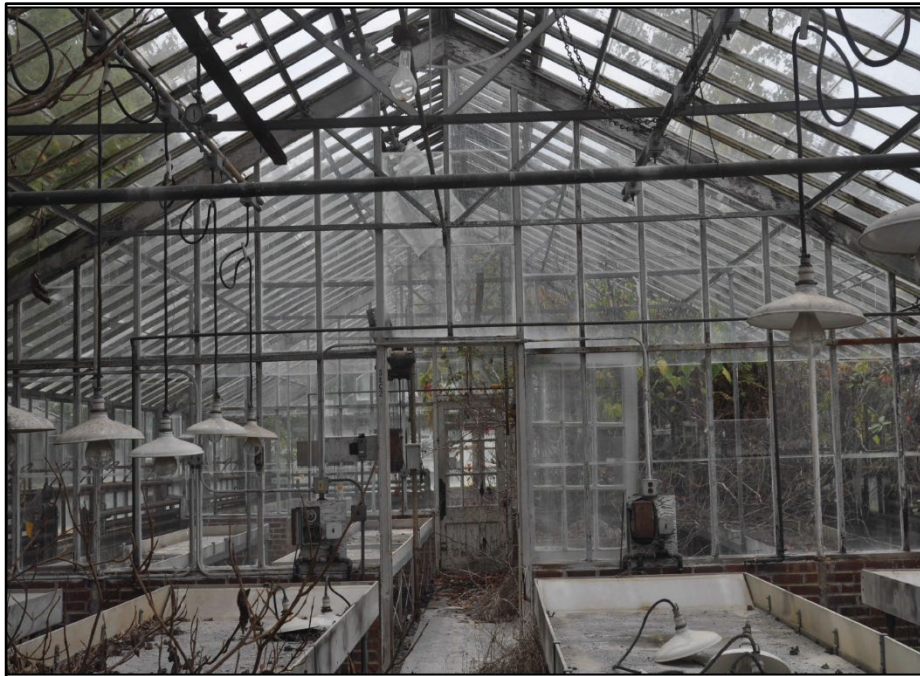
Photo 248: Building 0470, view of interior; photograph courtesy of Brian Clevon, 2017.
