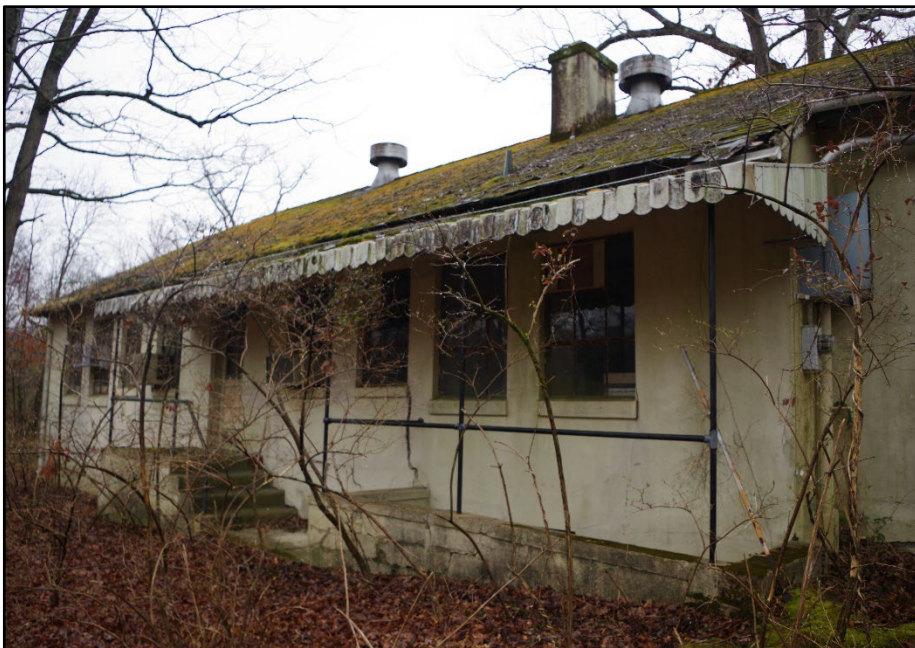
Photo 116: Building 0334, north elevation
