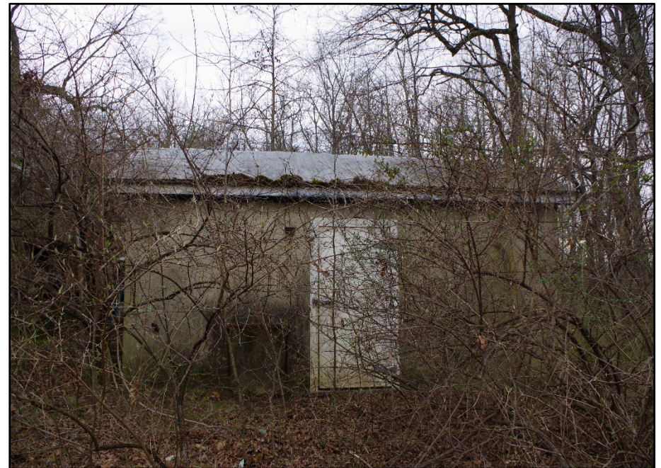
Photo 92: Building 0324A, north elevation
