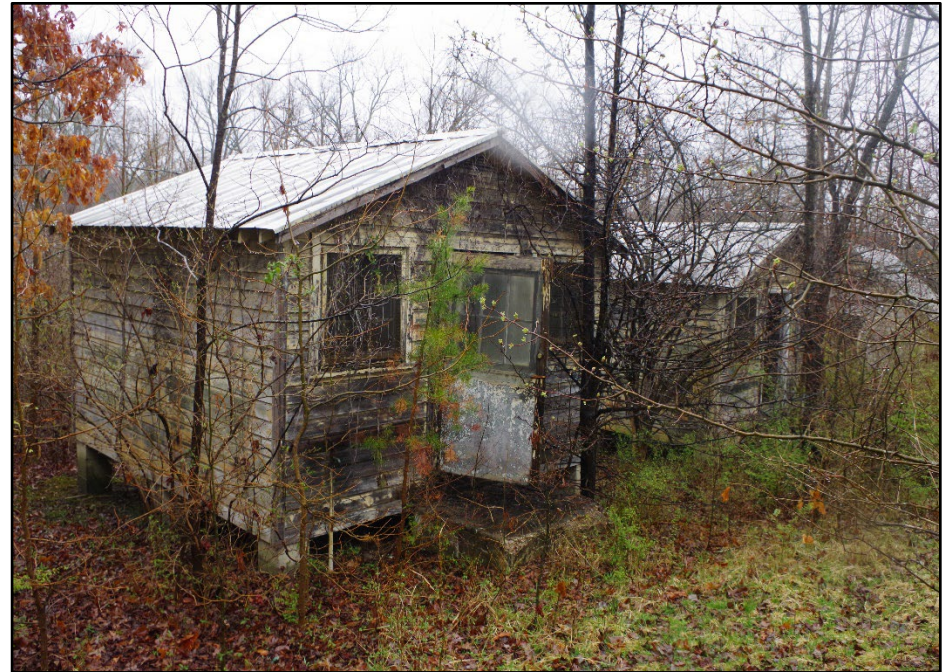
Photo 210: Building 0376, south elevation
