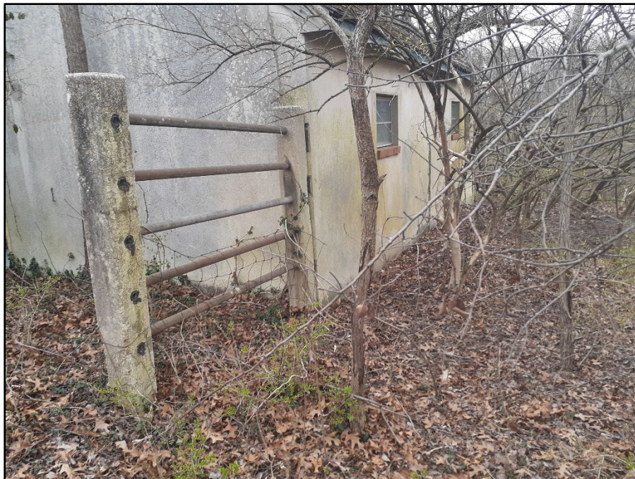
Photo 87: Building 0323, fence on east elevation
