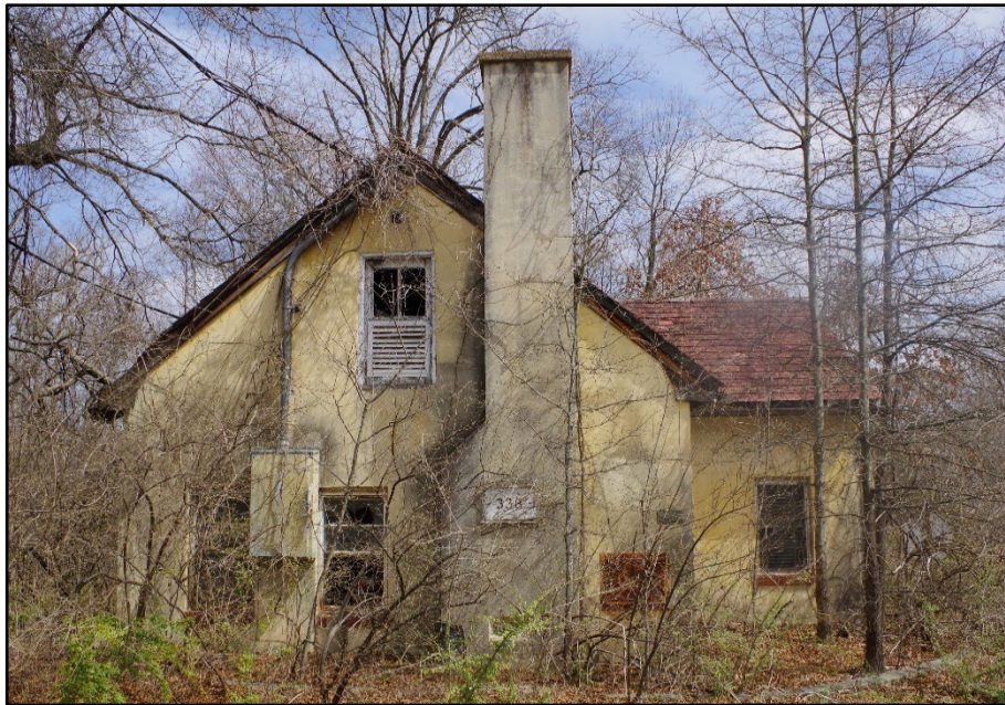
Photo 142: Building 0338, west elevation
