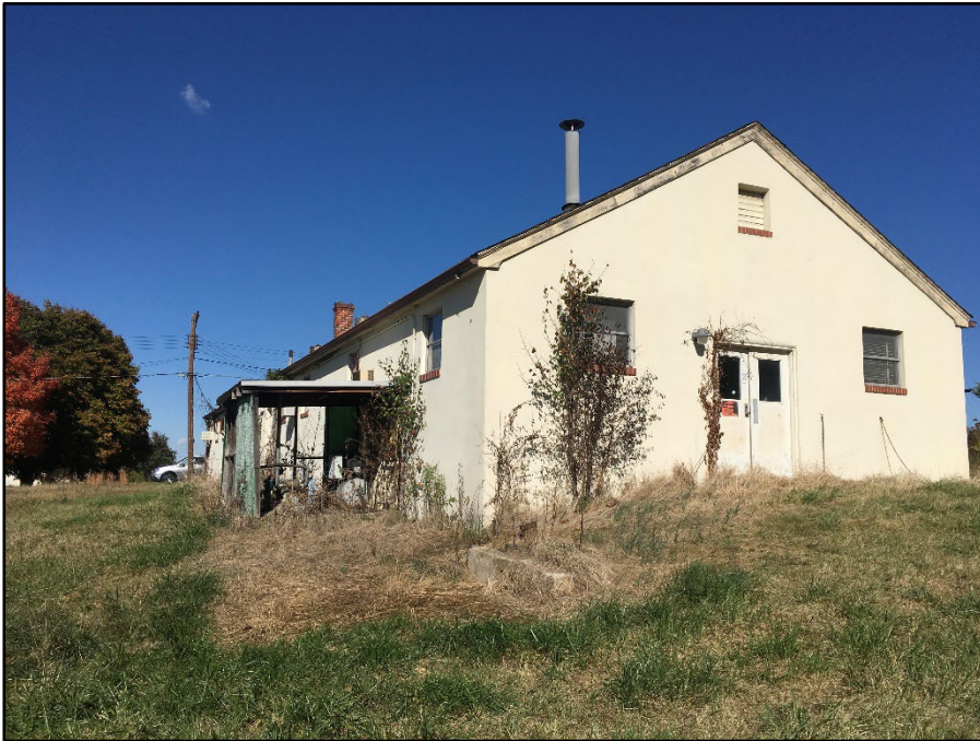
Photo 363: Building 1100, south and west elevations
