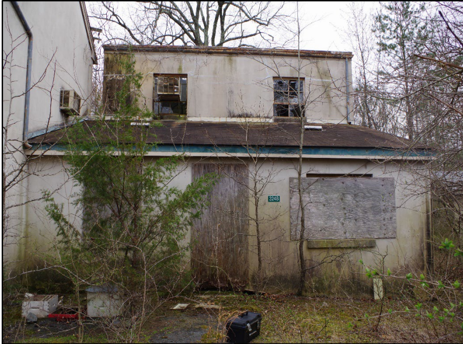
Photo 93: Building 0324B, north elevation
