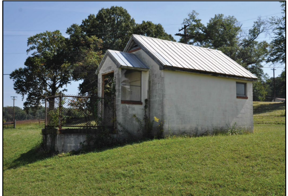
Photo 370: Building 1104, north and west elevations; photograph courtesy of Brian Clevin, 2017
