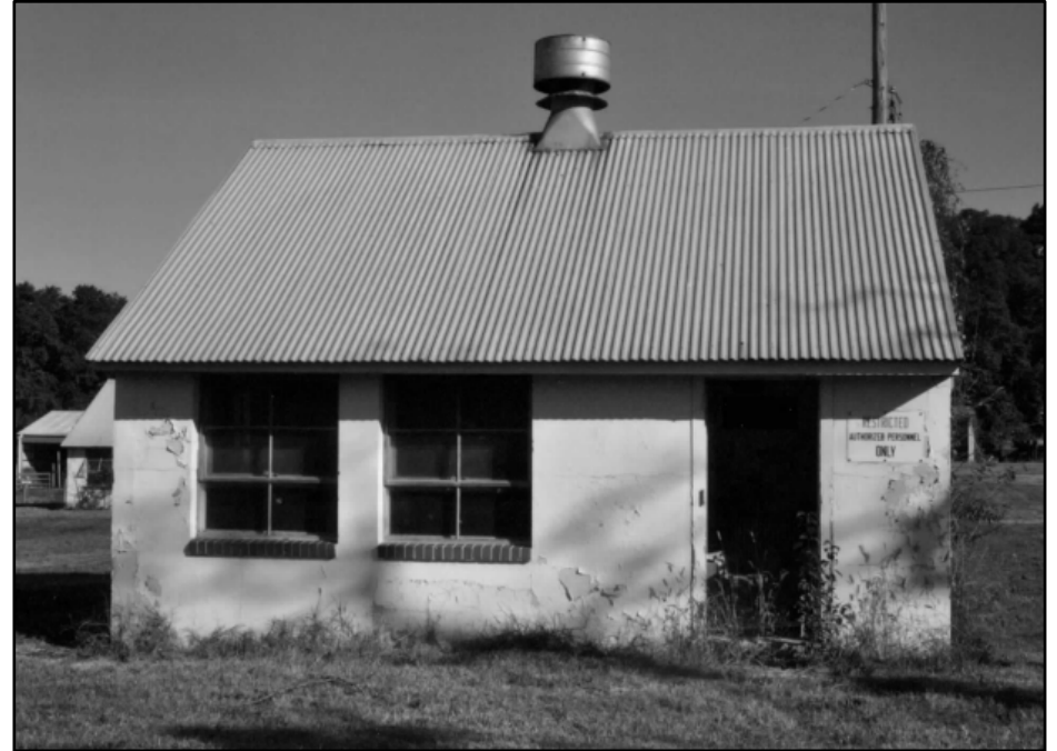
Photo 384: Building 1287, south elevation; photograph courtesy of Brian Clevon, 2017
