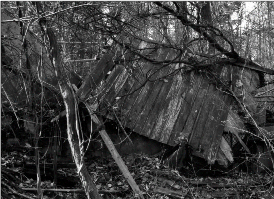
Photo 225: Building 0452, east elevation; photograph courtesy of Brian Clevon, 2017
