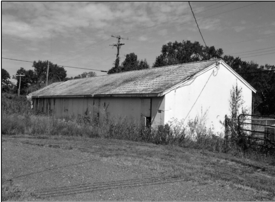
Photo 57: Building 0205, west and south elevations; photograph courtesy of Brian Clevon, 2017
