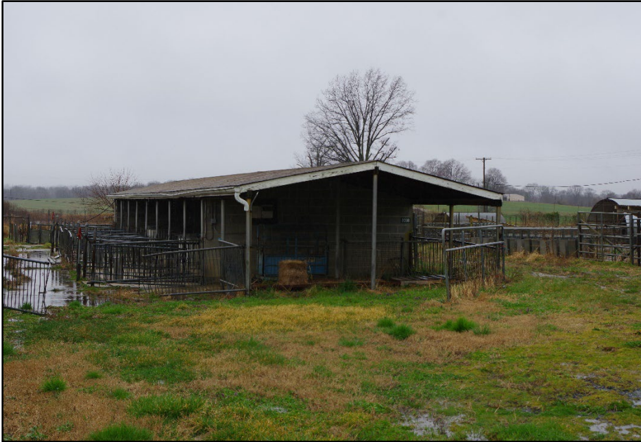
Photo 49: Building 0203B, overview
