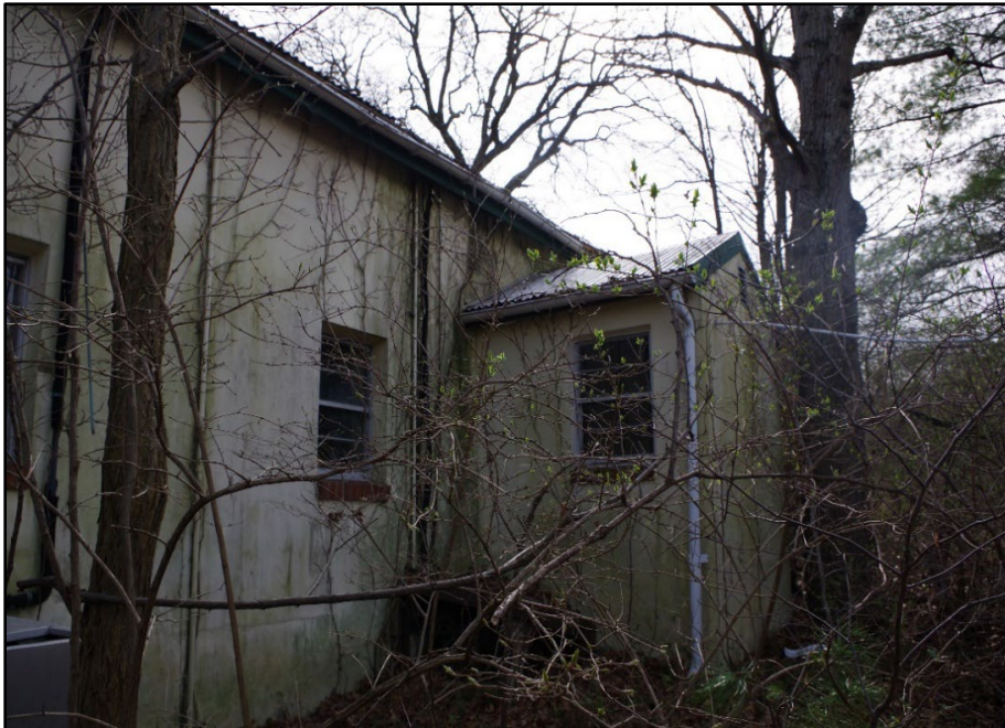
Photo 67: Building 0321, north elevation
