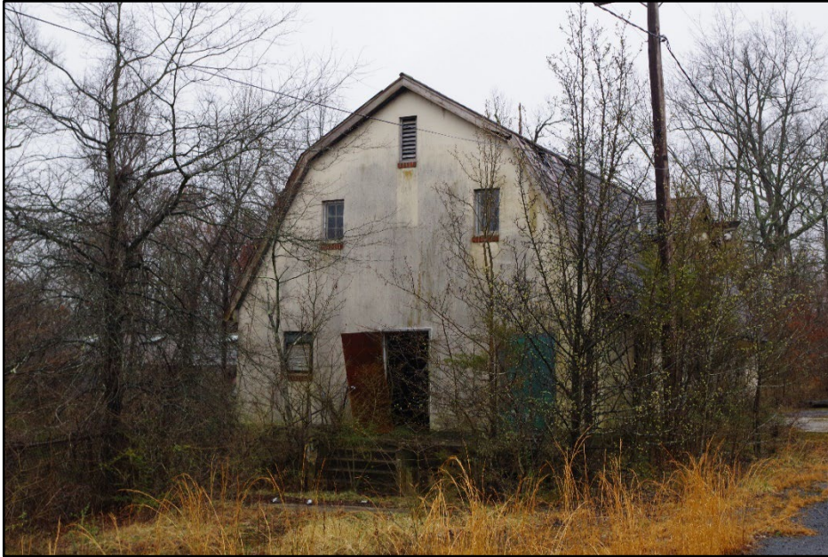
Photo 158: Building 0340, north elevation
