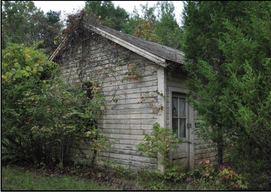
Photo 235: Building 0468, east and north elevations; photograph courtesy of Brian Clevon, 2017
