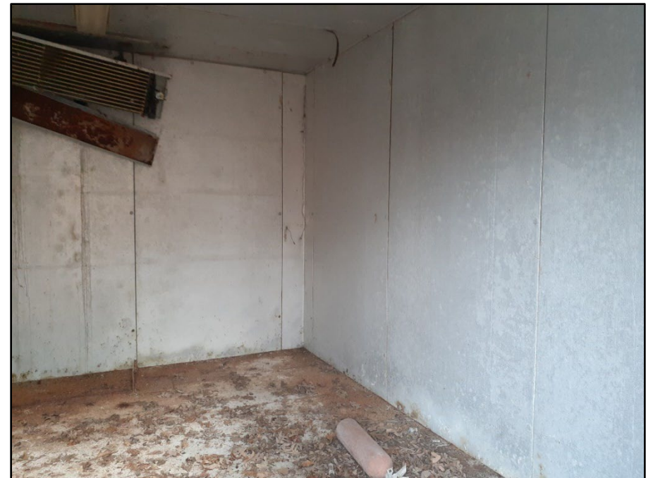
Photo 80: Building 0321B, interior
