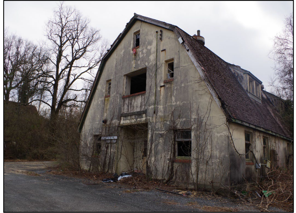
Photo 82: Building 0322, east elevation
