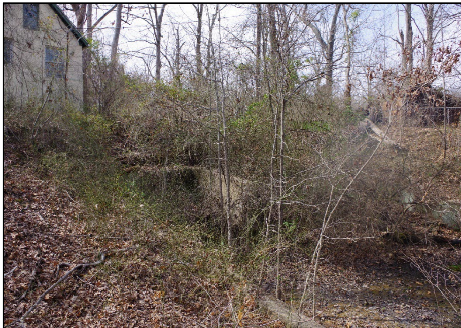
Photo 112: Building 0333, culvert near Building 0333
