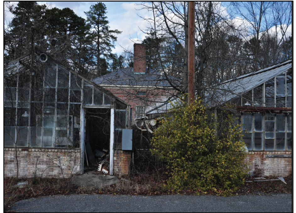
Photo 247: Building 0470, south elevation; photograph courtesy of Brian Clevon, 2017.
