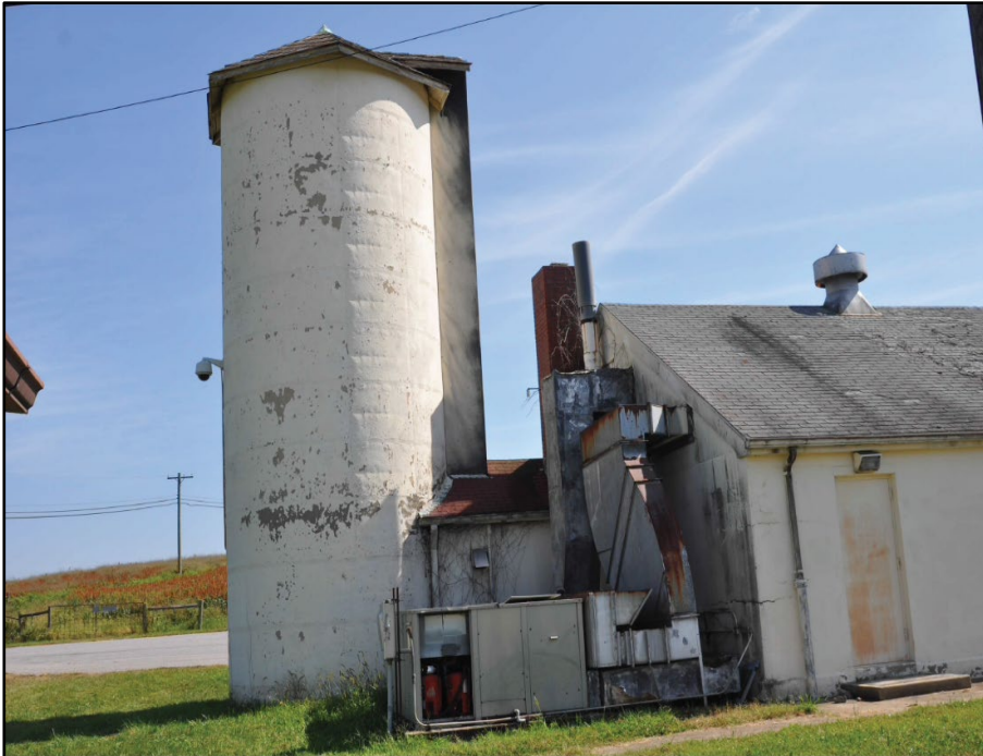
Photo 311: Building 1002, north and west elevations; photograph courtesy of Brian Clevin, 2017
