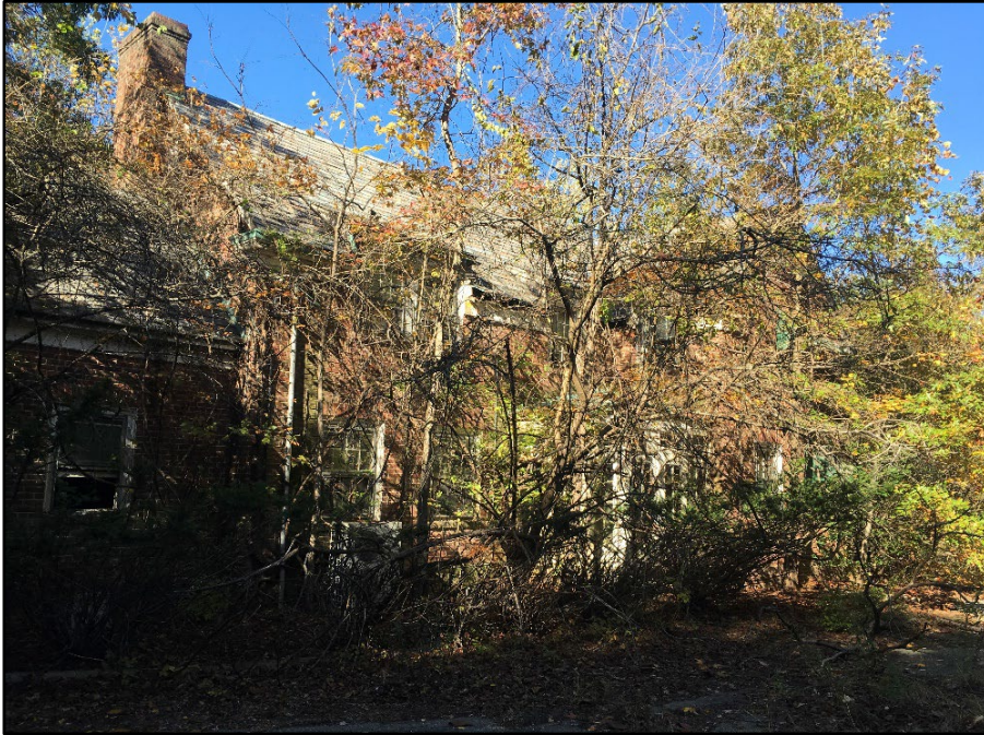
Photo 339: Building 1070, north elevation
