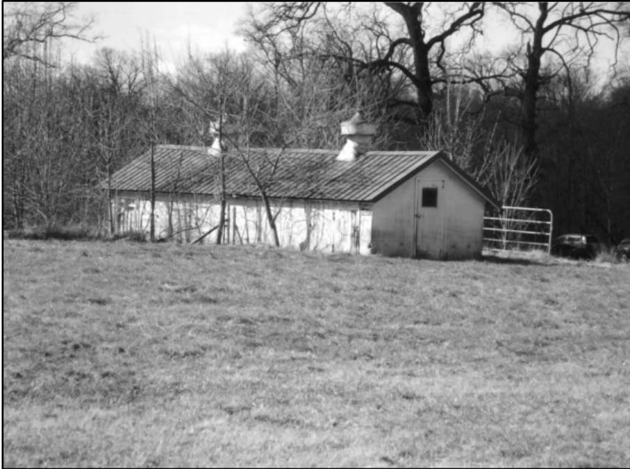
Photo 293: Building 04541C, east and north elevations; photograph courtesy of Mark Edwards and Brian Clevon, 2016
