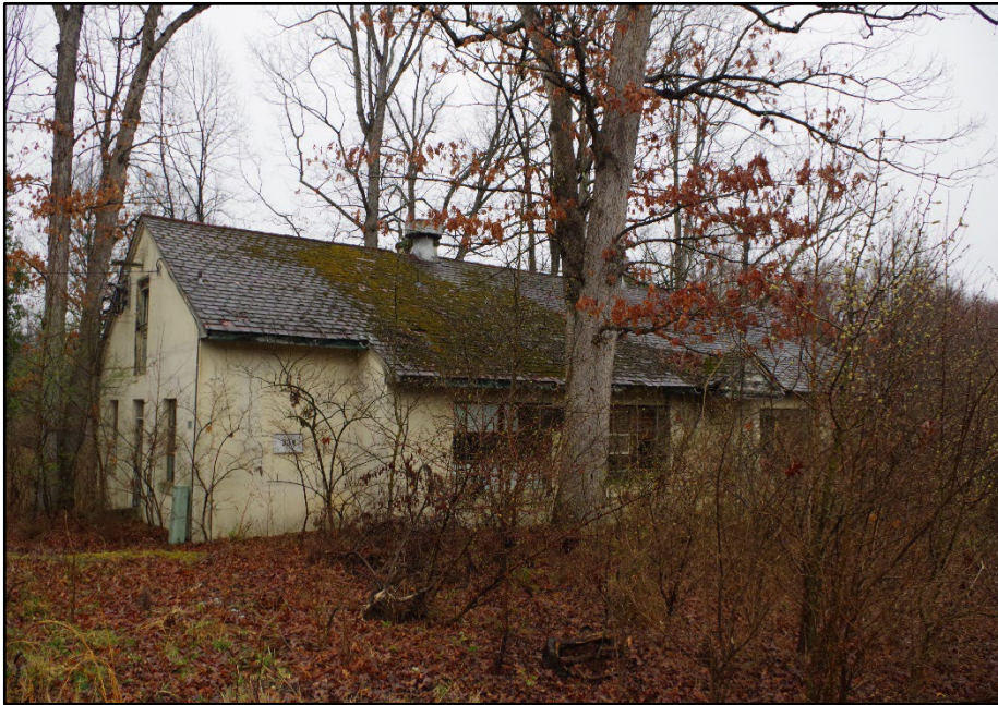
Photo 114: Building 0334, west and south elevations
