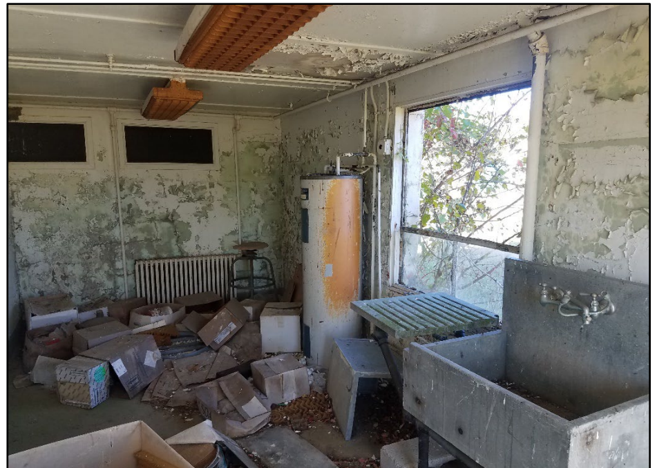
Photo 386: Building 1287, interior view
