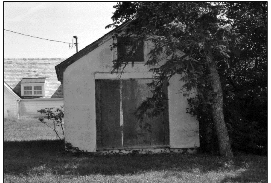
Photo 324: Building 1053, west elevation; photograph courtesy of Mark Edwards and Brian Clevon, 2016
