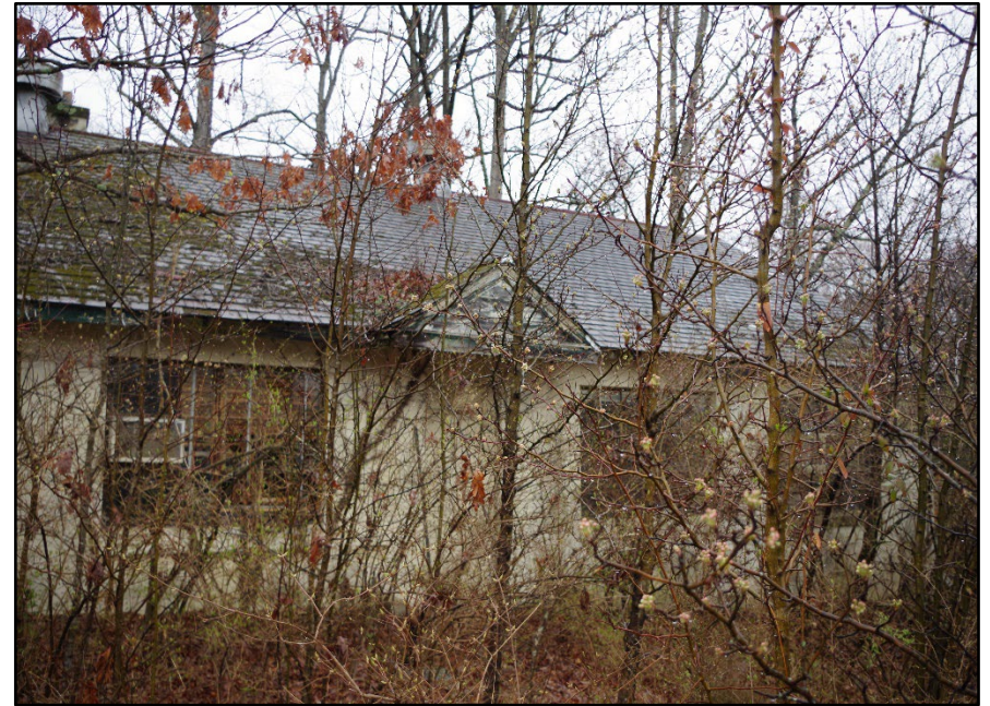
Photo 115: Building 0334, south elevation
