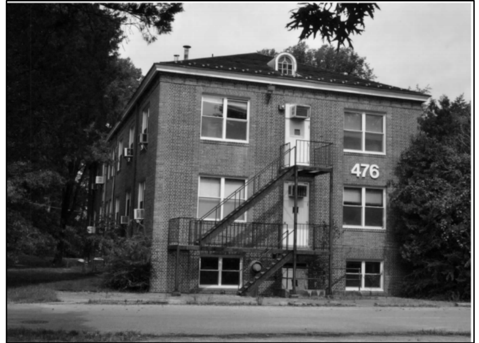
Photo 271: Building 0476, west and south elevations; photograph courtesy of Brian Clevon, 2017
