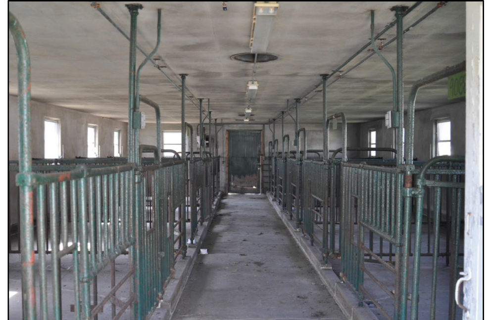
Photo 316: Building 1005, view of interior; photograph courtesy of Brian Clevon, 2017
