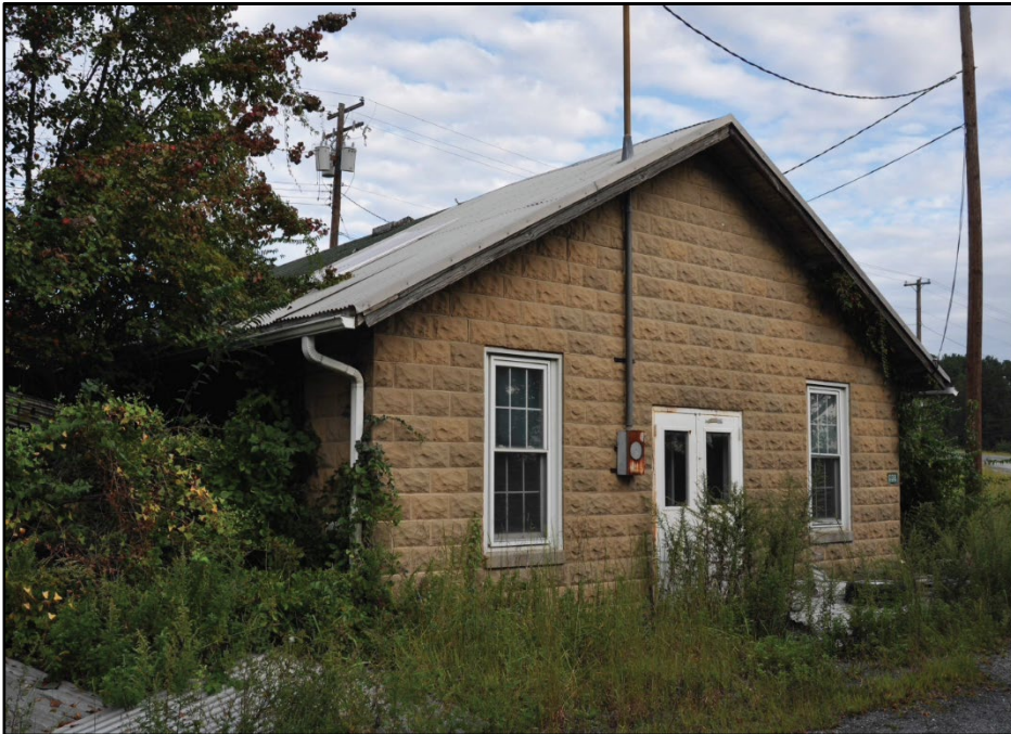
Photo 09: District Building 0038, east elevation; photograph courtesy of Mark Edwards and Brian Clevon, 2016
