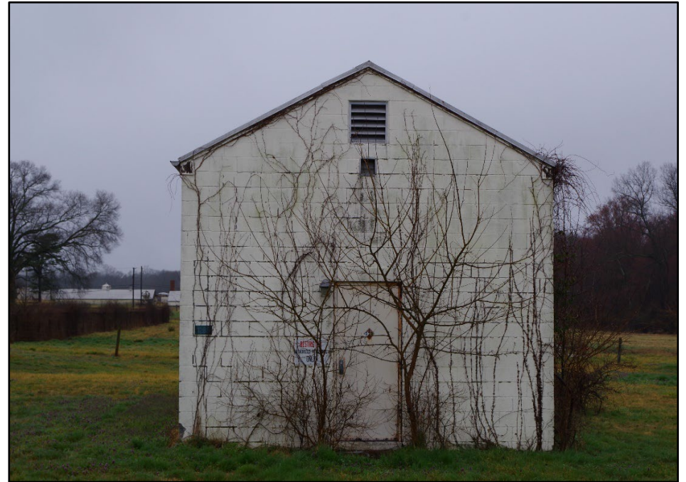
Photo 388: Building 1288, east elevation
