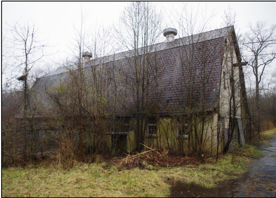
Photo 173: Building 0344, north elevation
