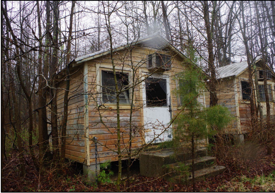
Photo 196: Building 0371, north elevation
