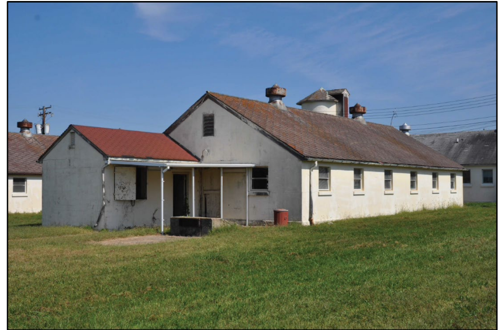
Photo 314: Building 1005, west and south elevations; photograph courtesy of Brian Clevon, 2017
