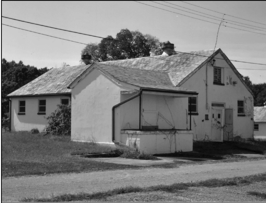
Photo 335: Building 1064, east and north elevations; photograph courtesy of Brian Clevon, 2017
