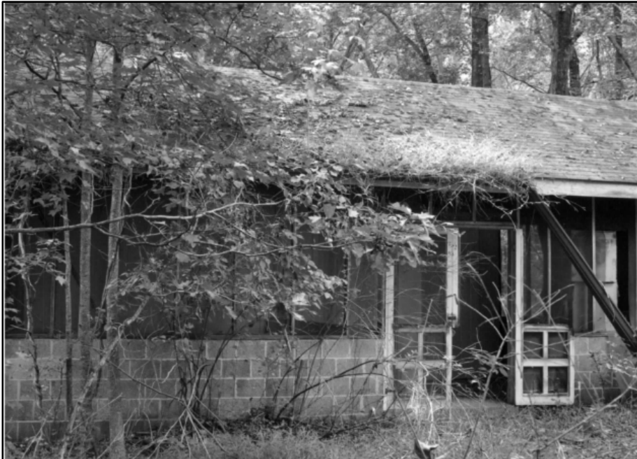
Photo 268: Building 0475, north elevation; photograph courtesy of Brian Clevon, 2017
