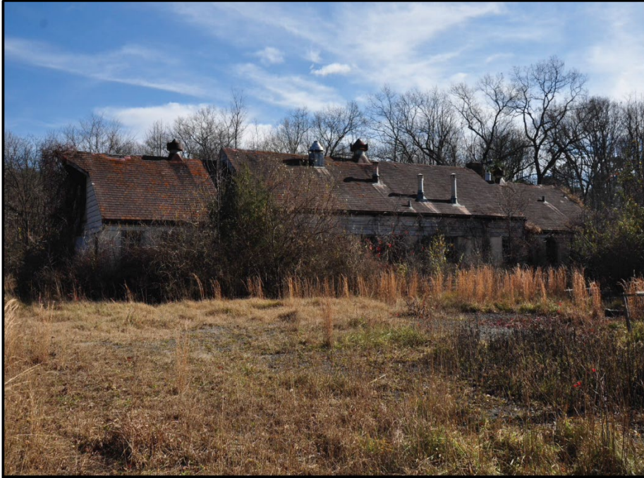
Photo 301: Building 0543, west elevation; photograph courtesy of Mark Edwards and Brian Clevon, 2016
