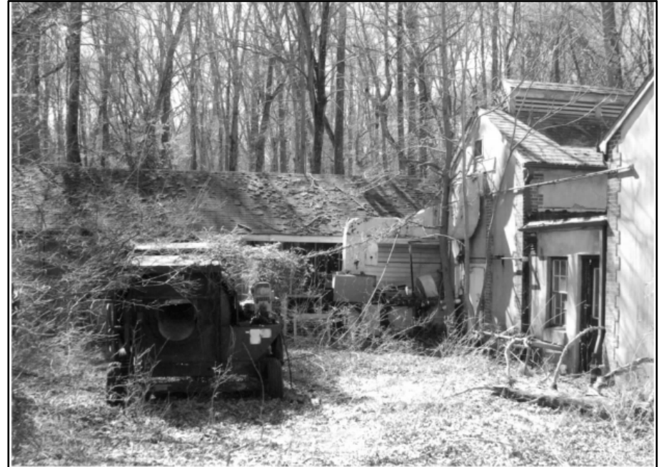
Photo 263: Building 0474, east and north elevations; photograph courtesy of Mark Edwards and Brian Clevon, 2016
