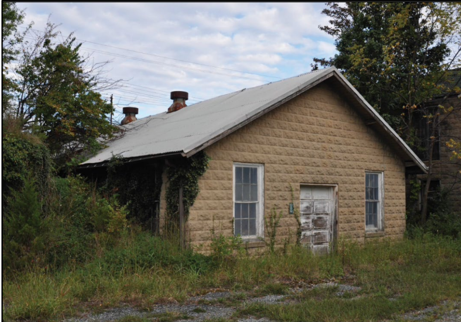
Photo 17: Building 0040, east elevation; photograph courtesy of Mark Edwards and Brian Clevon, 2016
