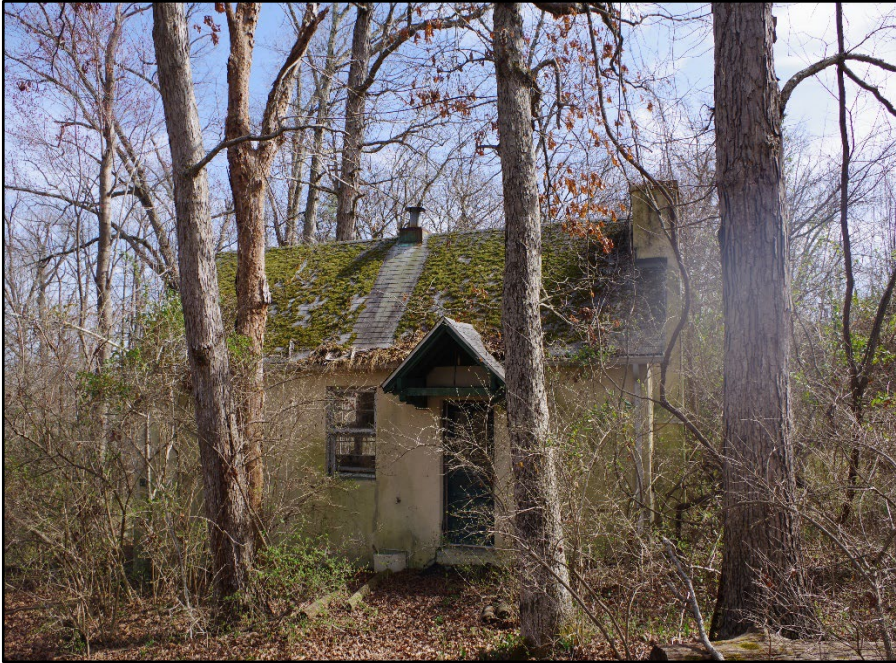
Photo 106: Building 0333, north elevation
