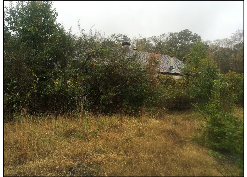
Photo 302: Building 0543, west elevation
