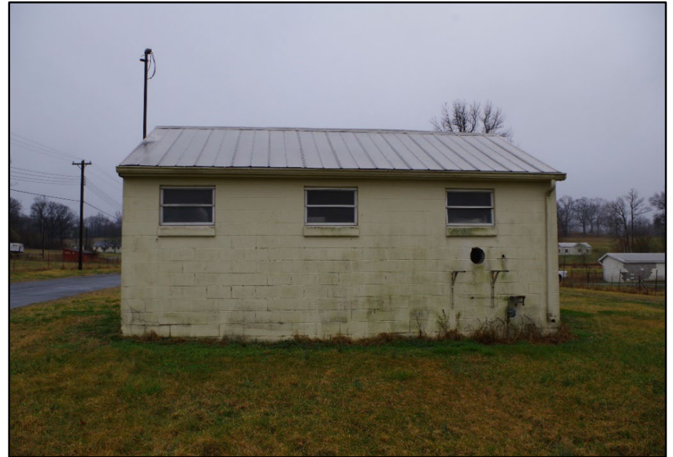
Photo 380: Building 1205, north facade
