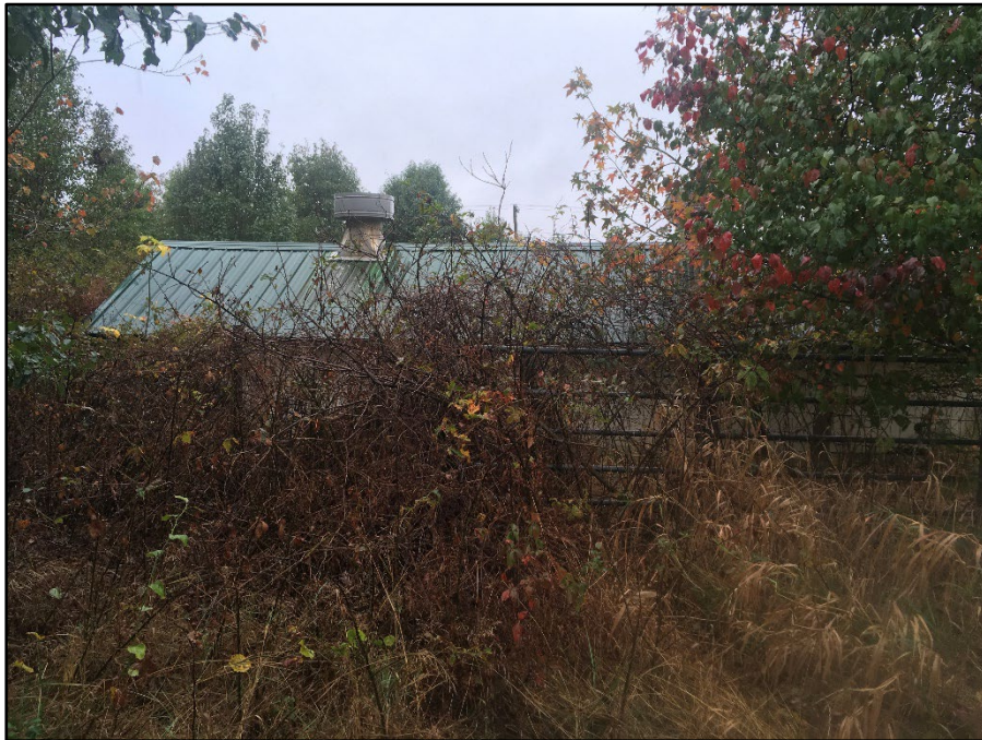
Photo 299: Building 0541D, west elevation
