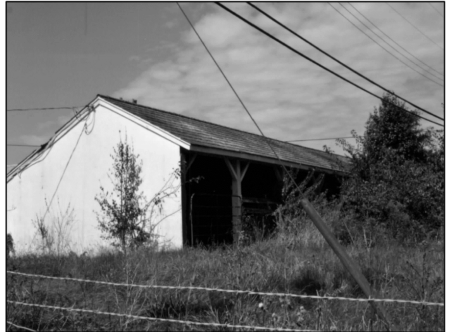
Photo 58: Building 0205, south and east elevations; photograph courtesy of Brian Clevon, 2017
