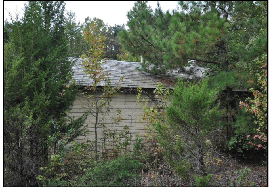
Photo 236: Building 0468, north elevation; photograph courtesy of Brian Clevon, 2017
