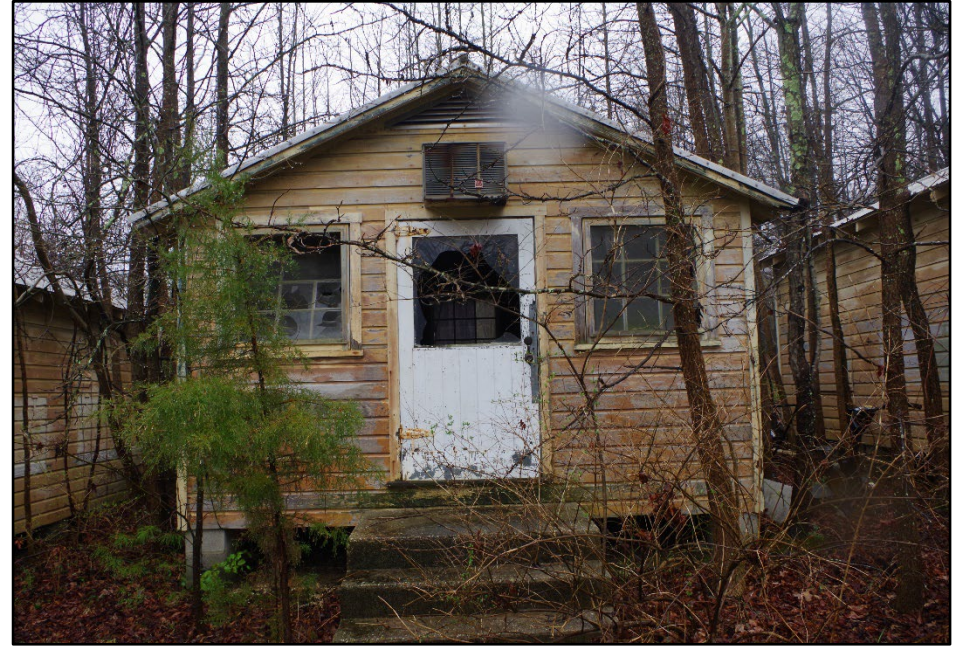
Photo 197: Building 0371, north elevation
