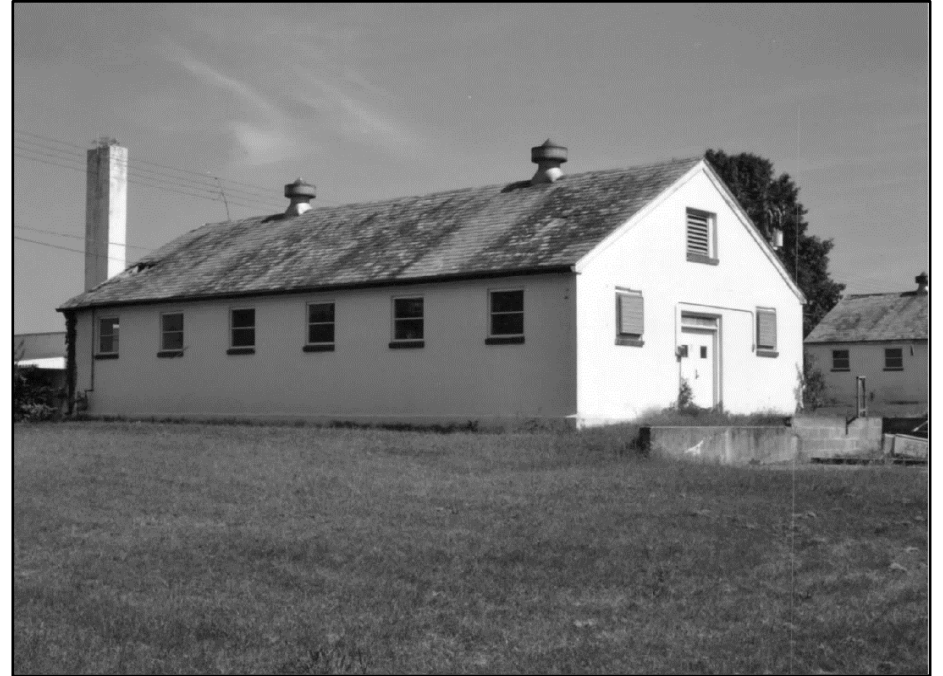
Photo 336: Building 1064, west and south elevations; photograph courtesy of Brian Clevon, 2017
