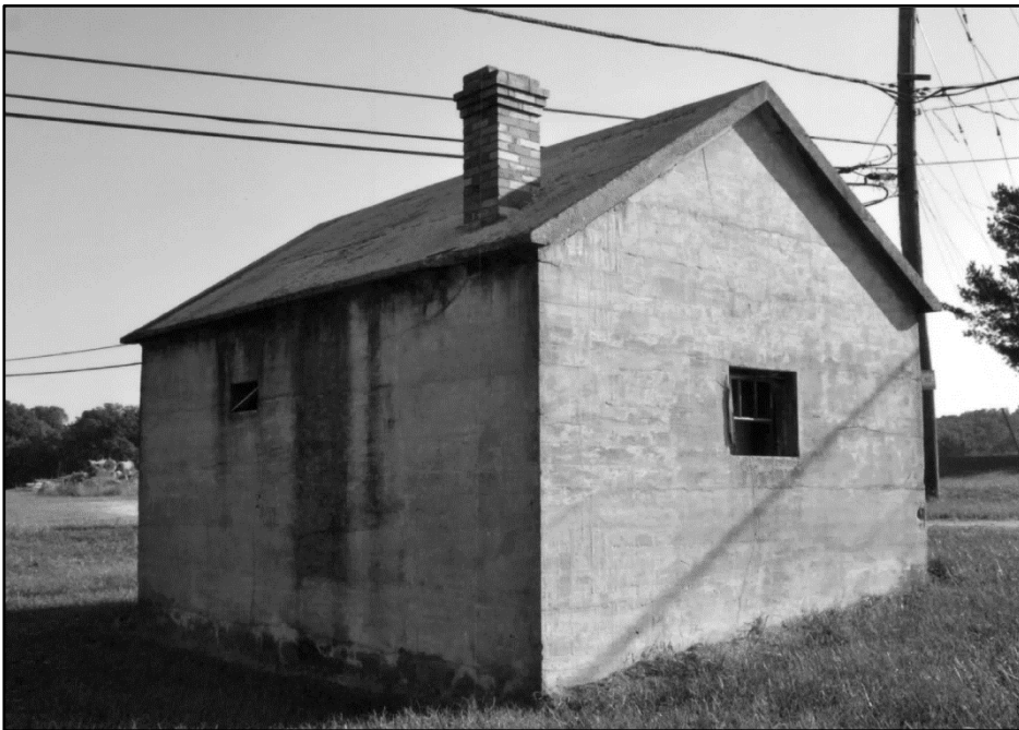
Photo 291: Building 0524, west and south elevations; photograph courtesy of Brian Clevon, 2017
