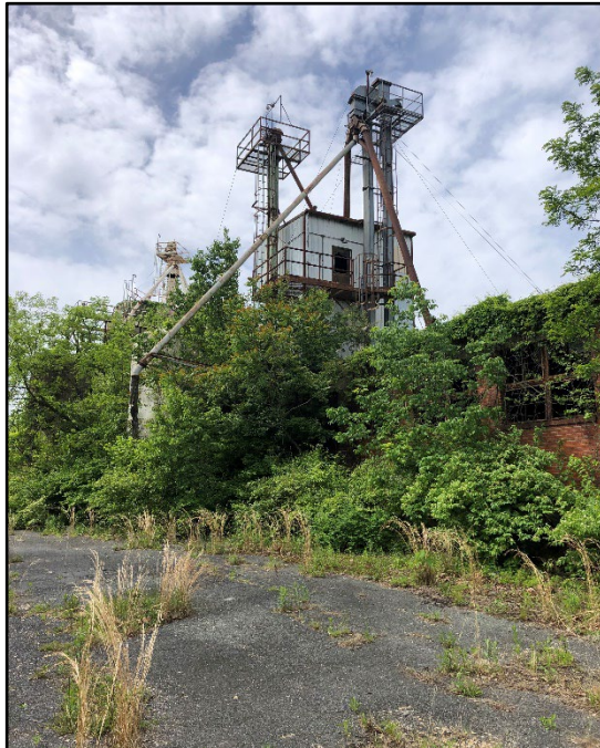
Photo 38: Building 0085, east elevation
