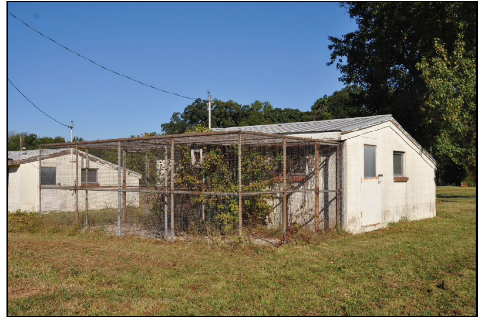
Photo 404: Building 1329, south and east elevations; photograph courtesy of Brian Clevon, 2017
