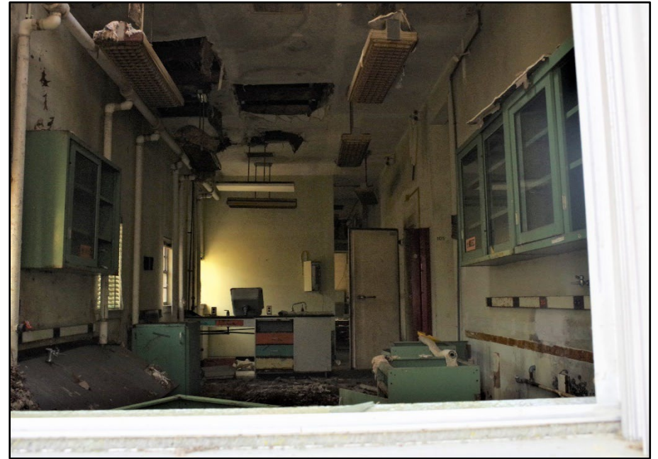
Photo 74: Building 0321, view of interior
