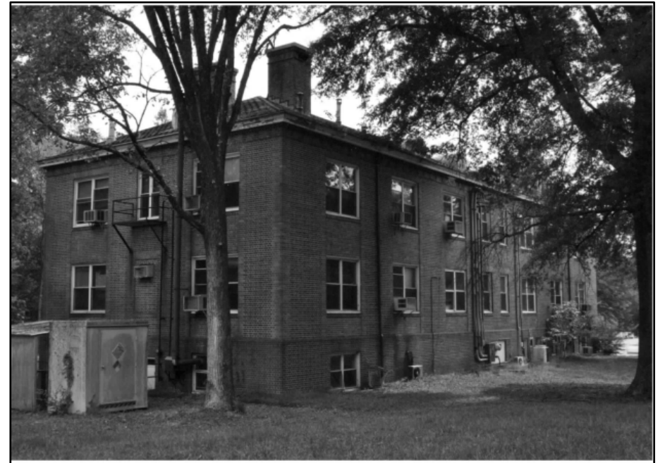
Photo 273: Building 0476, north and west elevations; photograph courtesy of Brian Clevon, 2017
