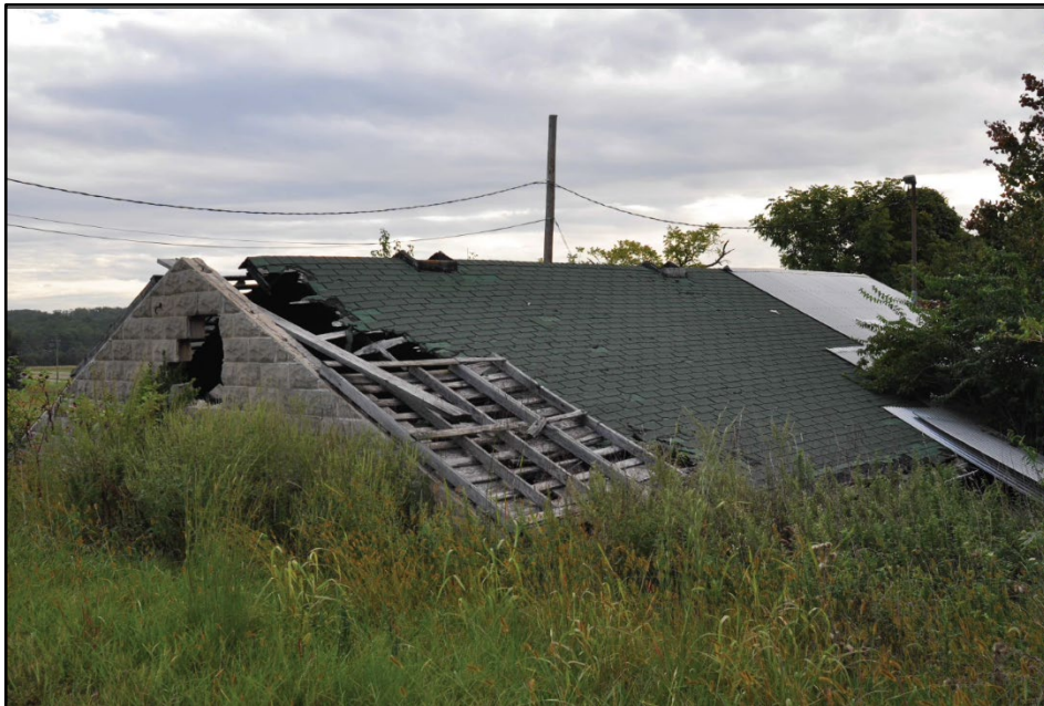
Photo 11: Building 0038, west elevation; photograph courtesy of Mark Edwards and Brian Clevon, 2016
