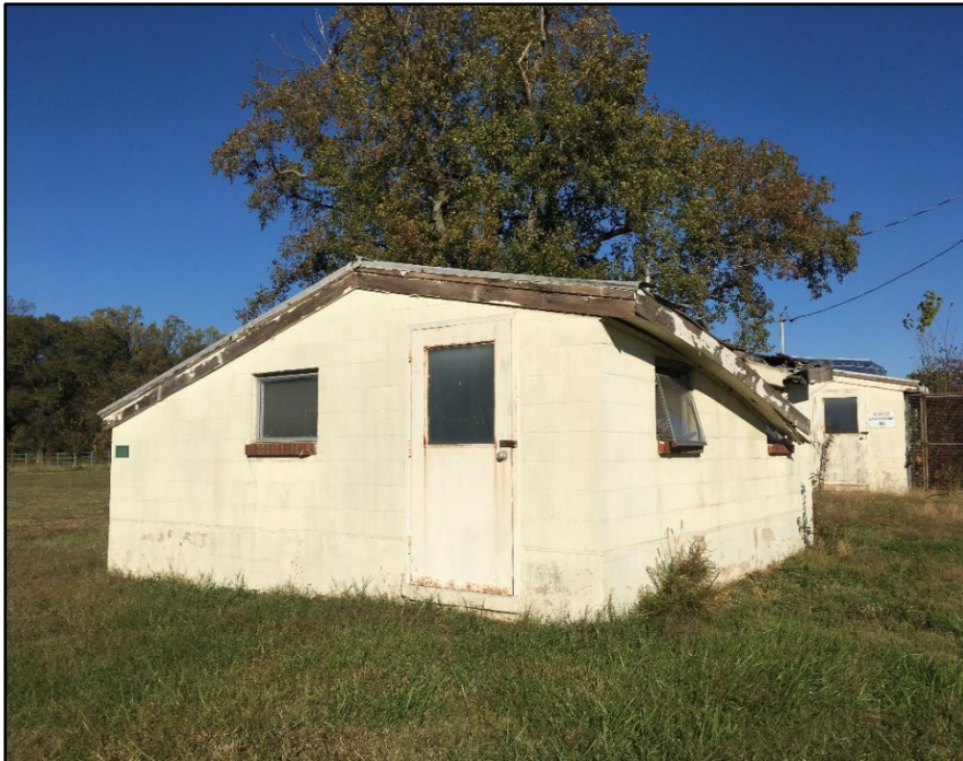
Photo 401: Building 1328, west and south elevations; photograph courtesy of Brian Clevon, 2017
