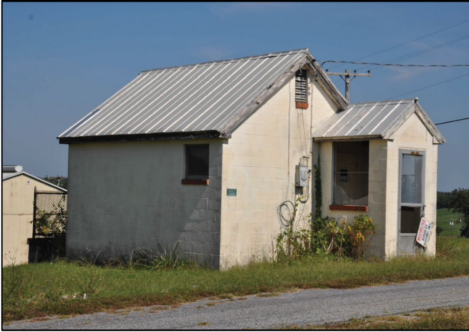
Photo 367: Building 1104, west and south elevations; photograph courtesy of Brian Clevin, 2017
