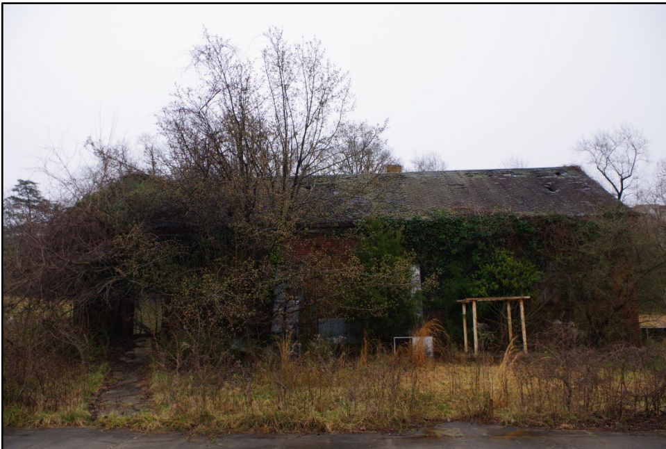
Photo 26: Building 0044, northwest elevation
