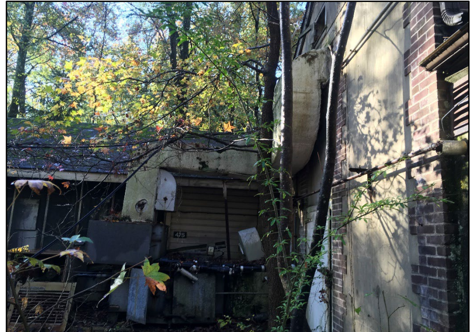
Photo 269: Building 0475, north elevation; photograph courtesy of Brian Clevon, 2017
