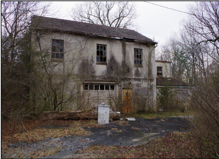
Photo 89: Building 0324, north elevation
