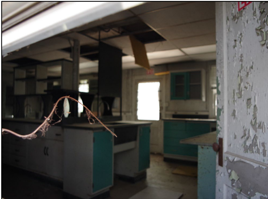
Photo 104: Building 0328, interior view
