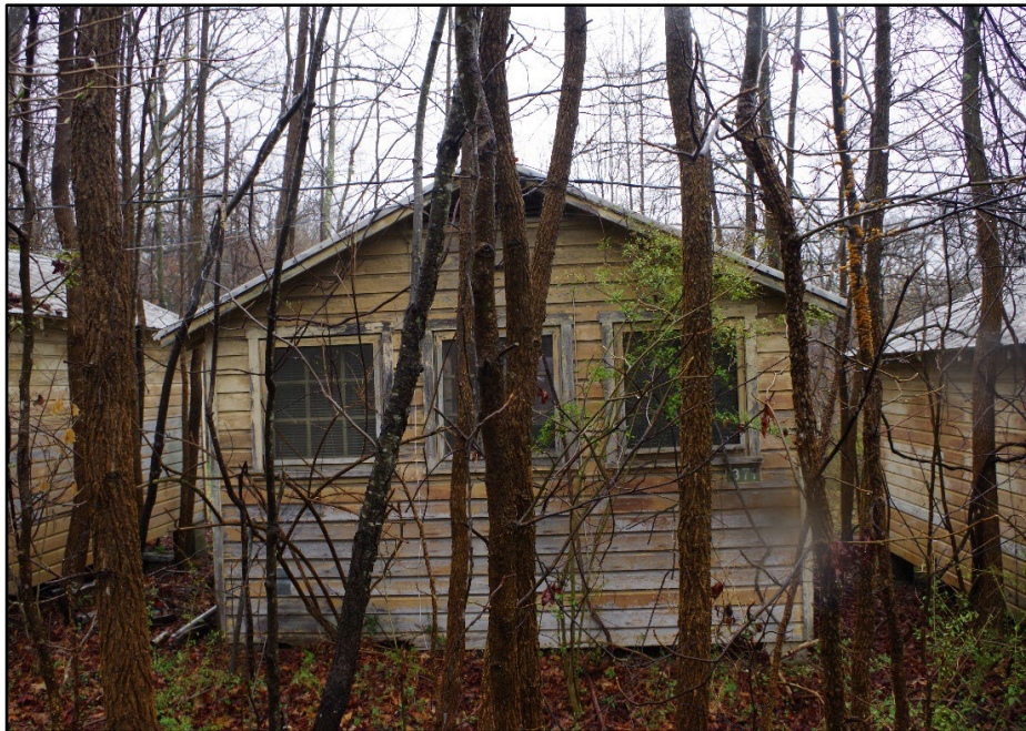
Photo 198: Building 0371, south elevation
