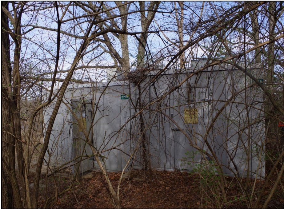
Photo 77: Buildings 0321A and 0321B, overview
